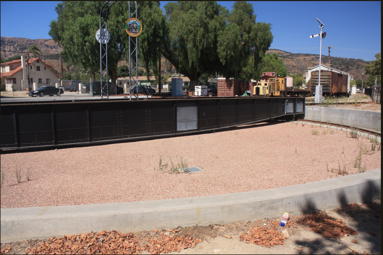
Another view of the F&W turntable. This 80-ton turntable was originally installed in Capreol, Ontario, in 1906. In 2007, the Santa Clara River Valley Railroad Historical Society purchased the turntable from the Canadian National Railway and was installed it here. The turntable allows not only turning of F&W locomotives and cars but also access to facilities in the narrow yard area.
