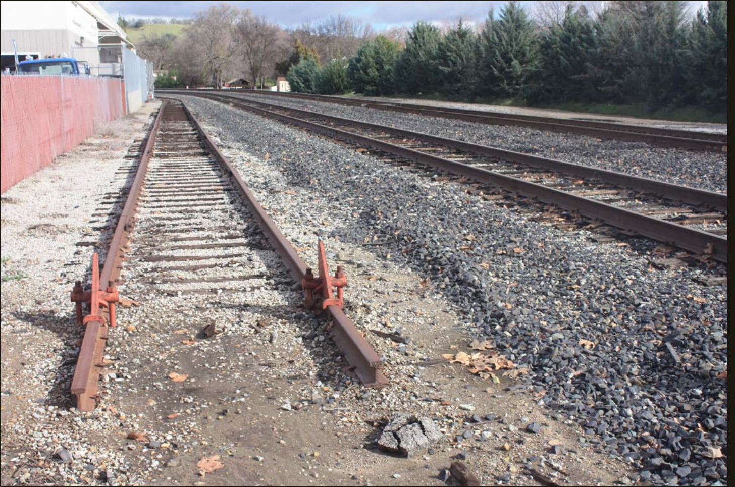
Northward view of the SP (1894) and two sidings at Santa Margarita.
