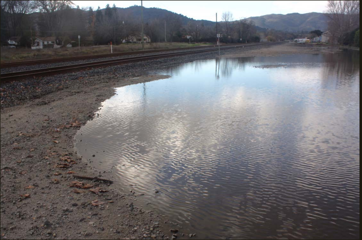
Southward view of the SP (1894) at Santa Margarita, with the Santa Lucia Mountains in the distance. In the 8 linear miles between here and San Luis Obispo, the line crosses the mountain and then drops about 1,000 feet to San Luis Obispo (at 230 feet above sea level).
