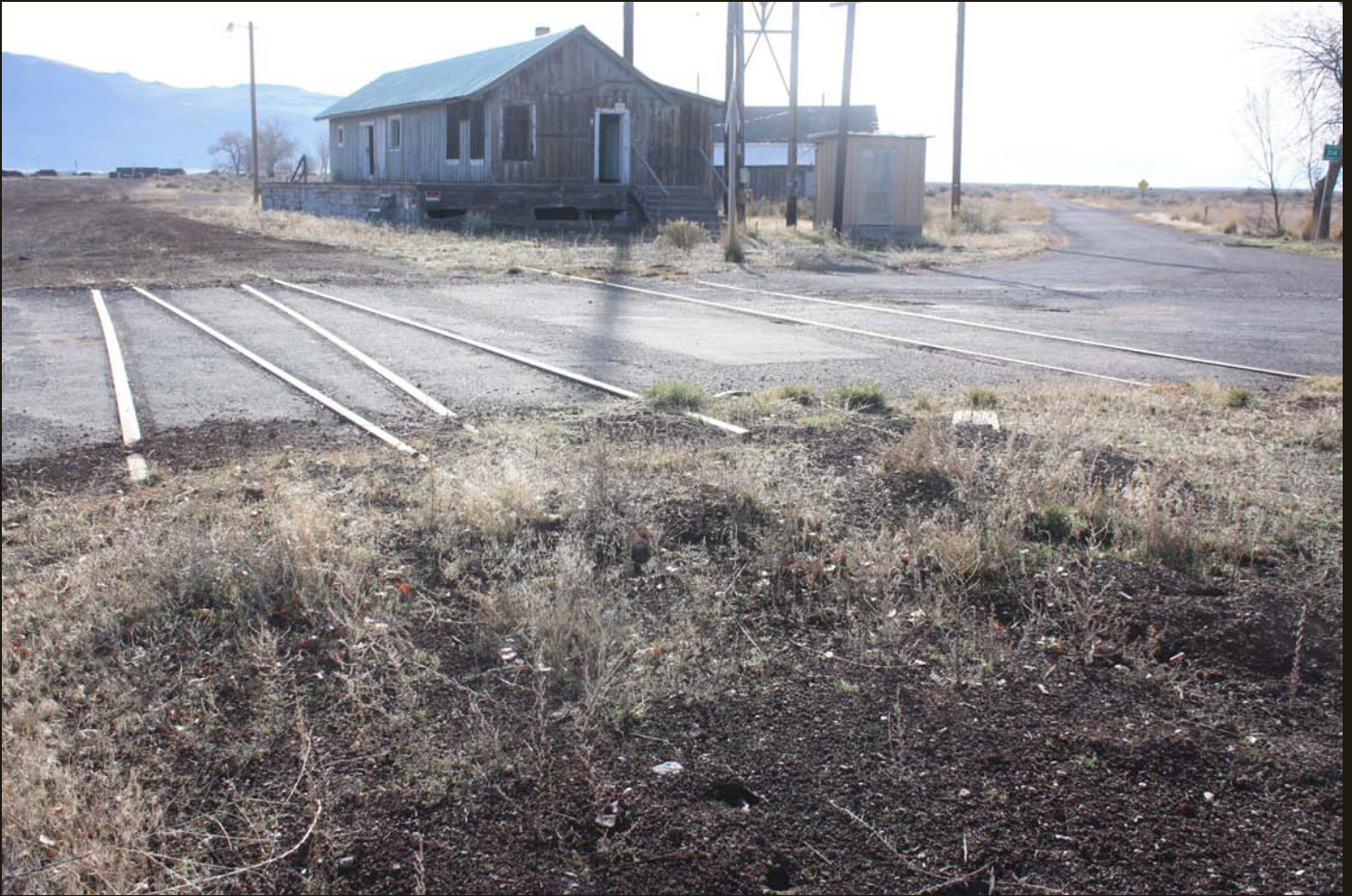
Same crossing as previous, showing an old loading facility along the F&L. The N-C-O rails have part of switch for a former siding.
