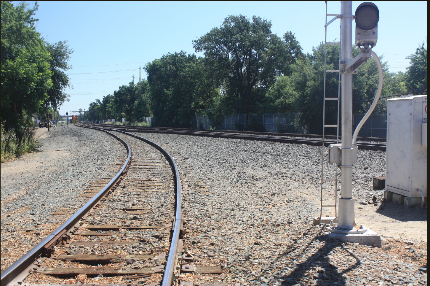
Eastward view of the Cal-P (1870) at Davis, a few steps north of the previous location. The bolted track in the foreground is the east branch of the Davis wye and the double track with the same mixed freight train as before is the UP/Amtrak line.
