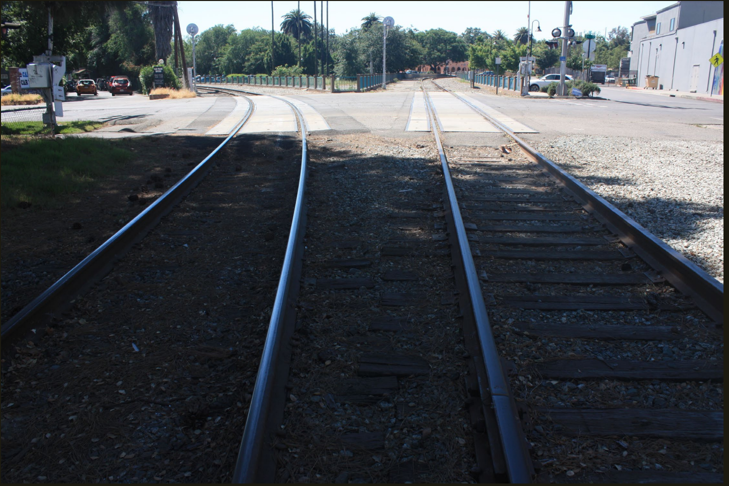
Southward view of the north tip of the Davis wye; the east branch is on the left and the west branch is on the right. The station is barely visible down the west branch.
