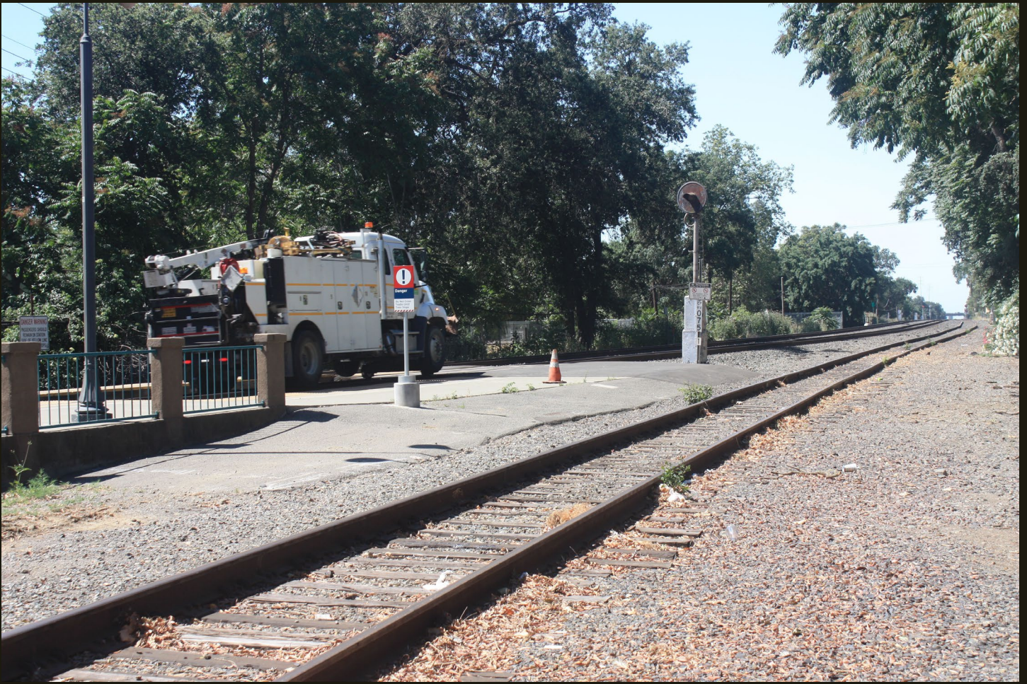
Southwestward view of the Cal-P (1870) route split at Davis, a few steps east of the previous location. The double track beyond the truck is the line to Sacramento and the track in the foreground is the west branch of the Davis wye.
