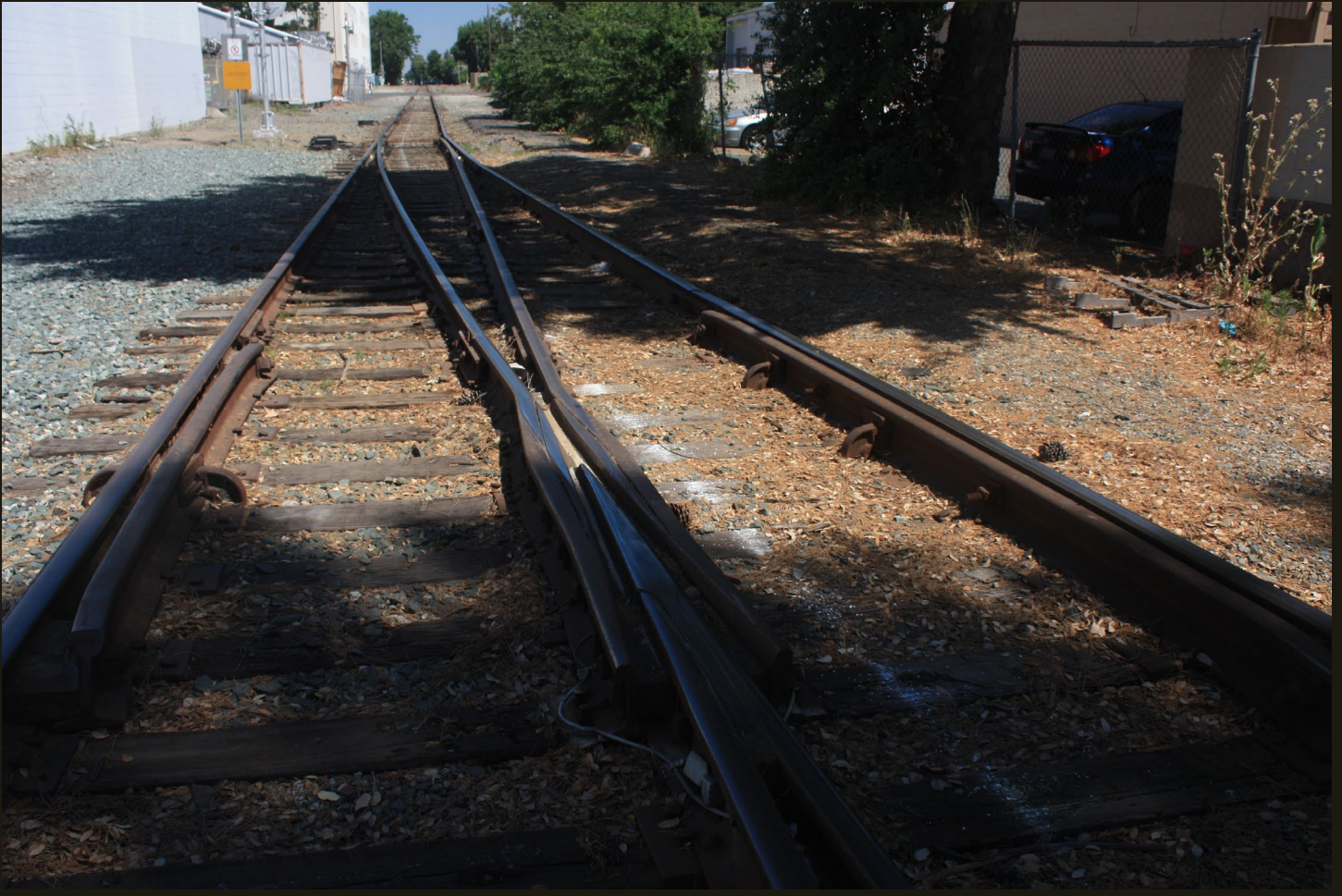
Northward view of the north tip of the Davis wye, which heads north to Woodland (10 miles north of Davis) where CN-operated trackage continues north along the former Northern Railway (1882).
