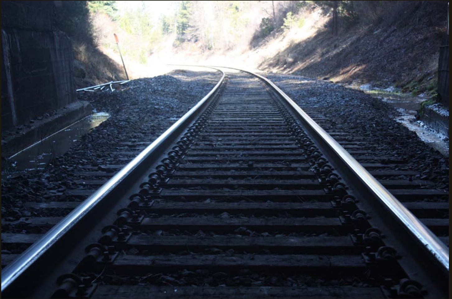
Groundwater drains out of the Spring Garden Tunnel.
