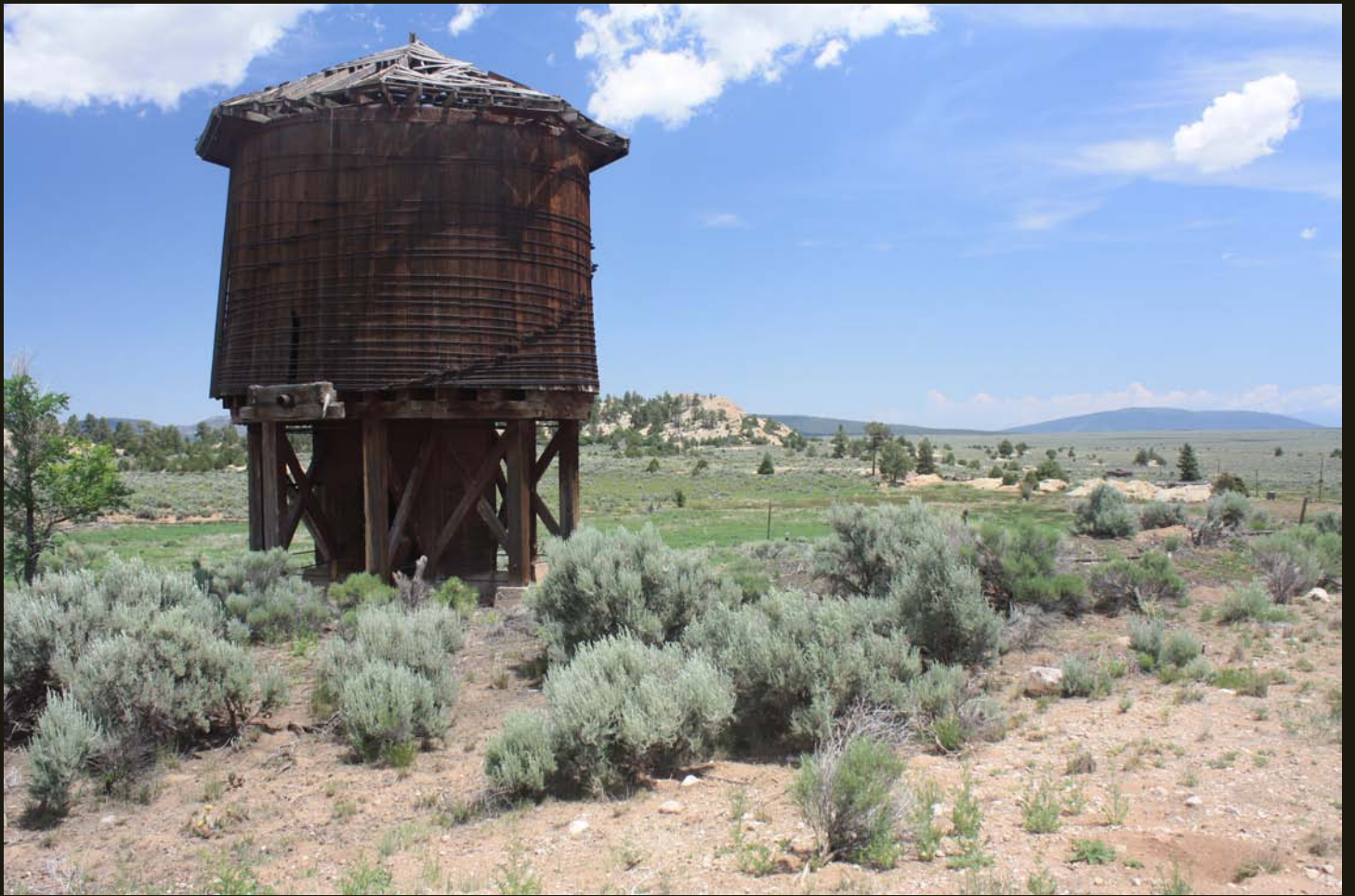
Closer view of the Tres Piedras water tower; the grade is not discernable in this view.
