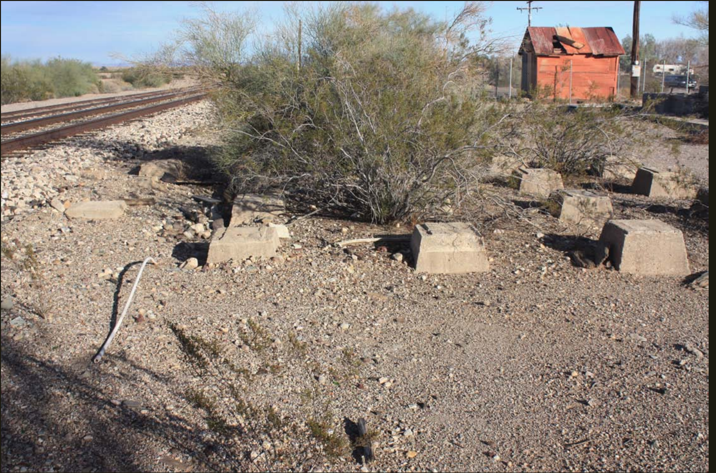
Eastward view of old facilities and foundations along the A&C at Vidal.
