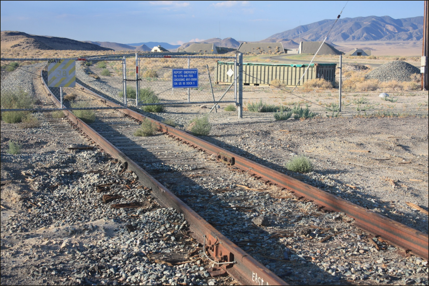
Southward view of the Army's loop track, same location as previous (after crossing to the south side of U.S. Highway 95). Several bunkers are visible. The track is curving to the right (west) to complete the loop.
