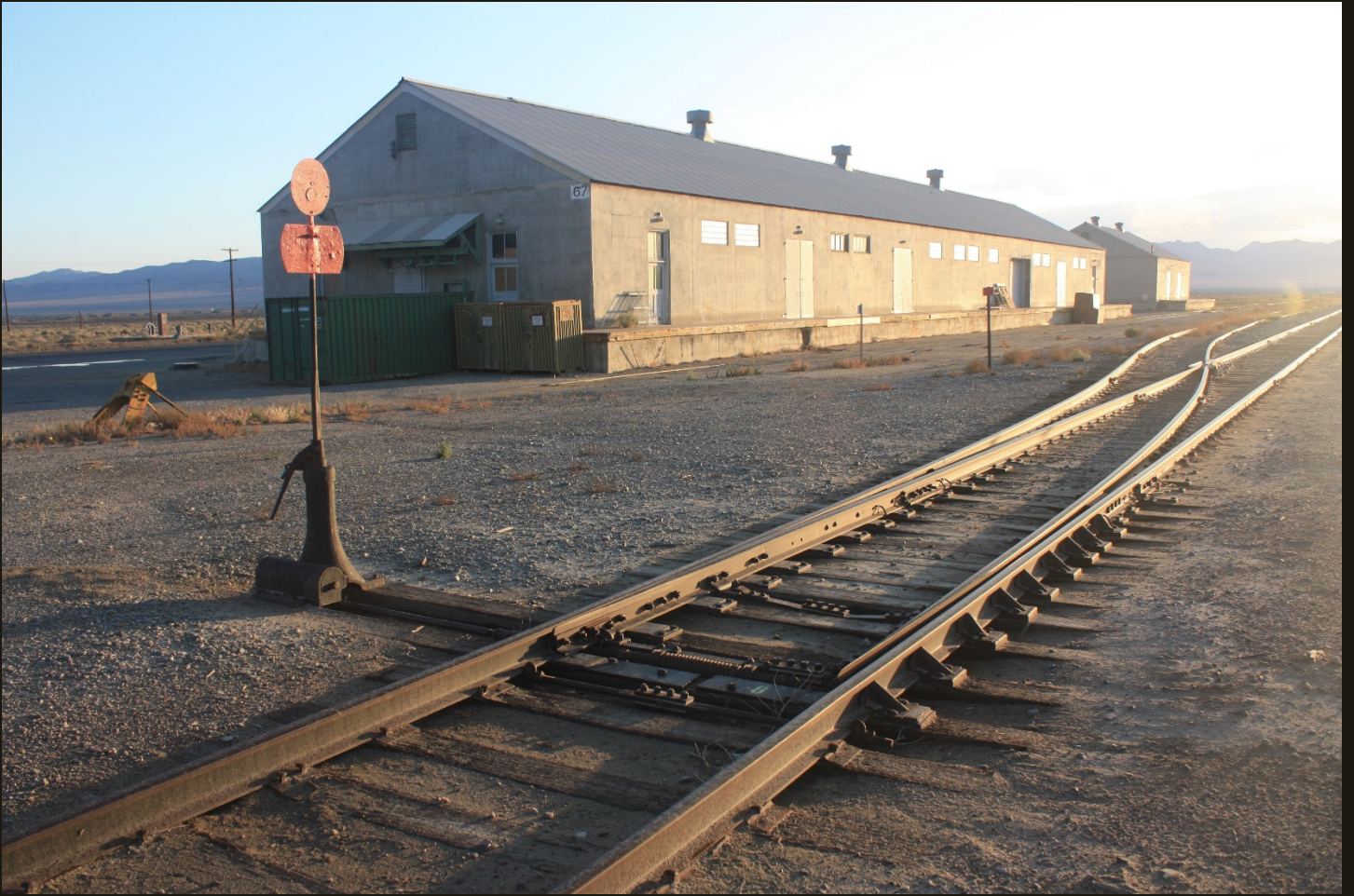
Northeastward view at the same location as previous with the same switch in the foreground. The switch is for a siding for an apparently abandoned Army loading facility.
