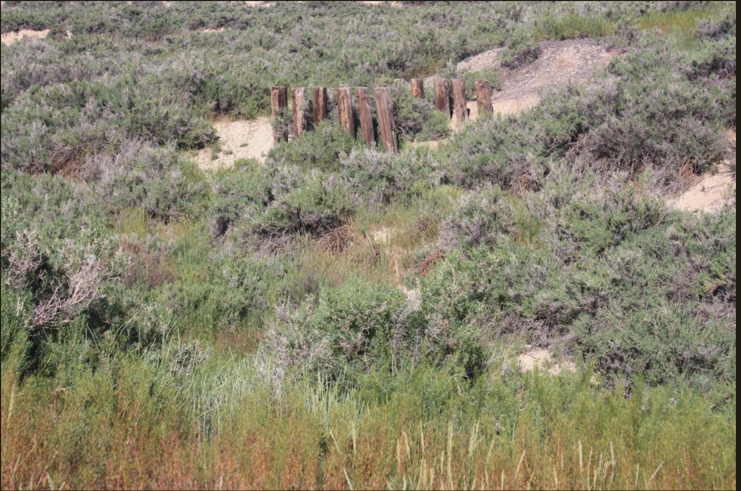
The dry creek of Horsethief Canyon at Thayer Junction. The piles carried the Superior Branch over the dry creek to the grade visible on the right. A web page for the town of Superior notes that "about 1903 plans were laid for the construction of a railroad from Thayer Junction on the main line to Superior," so I estimate the construction completion year as c1905.
