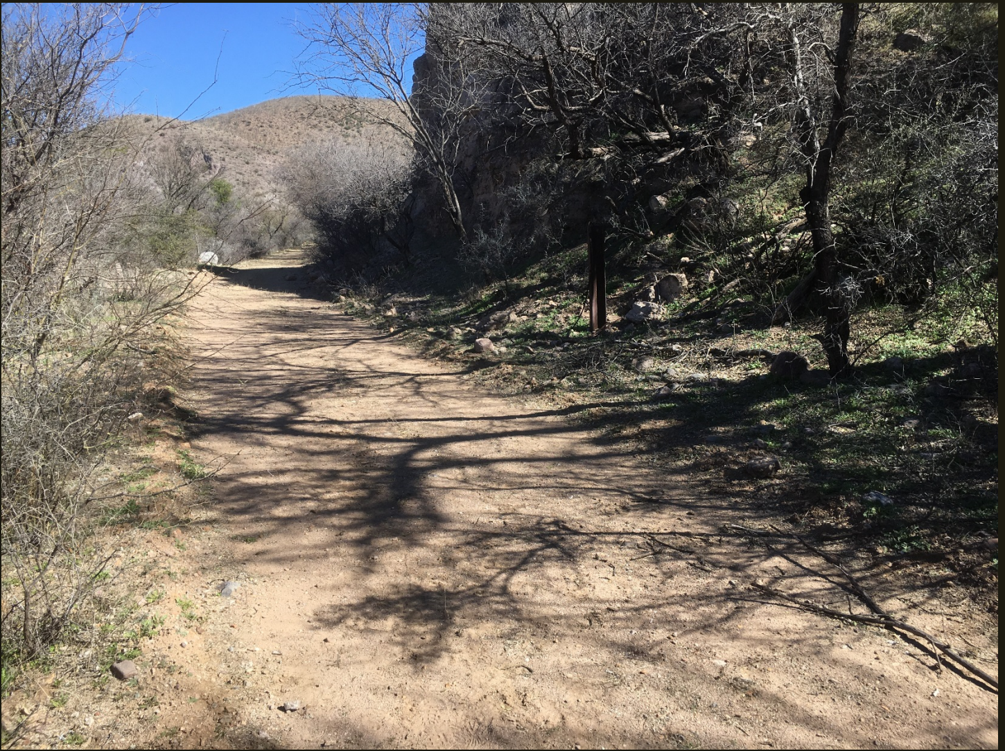
Northward view of the NM&A (1882), 500 feet southwest of the previous location. The fill grade of the first two photos is replaced here by a substantial cut grade to negotiate a narrow part of Sonoita Creek.
