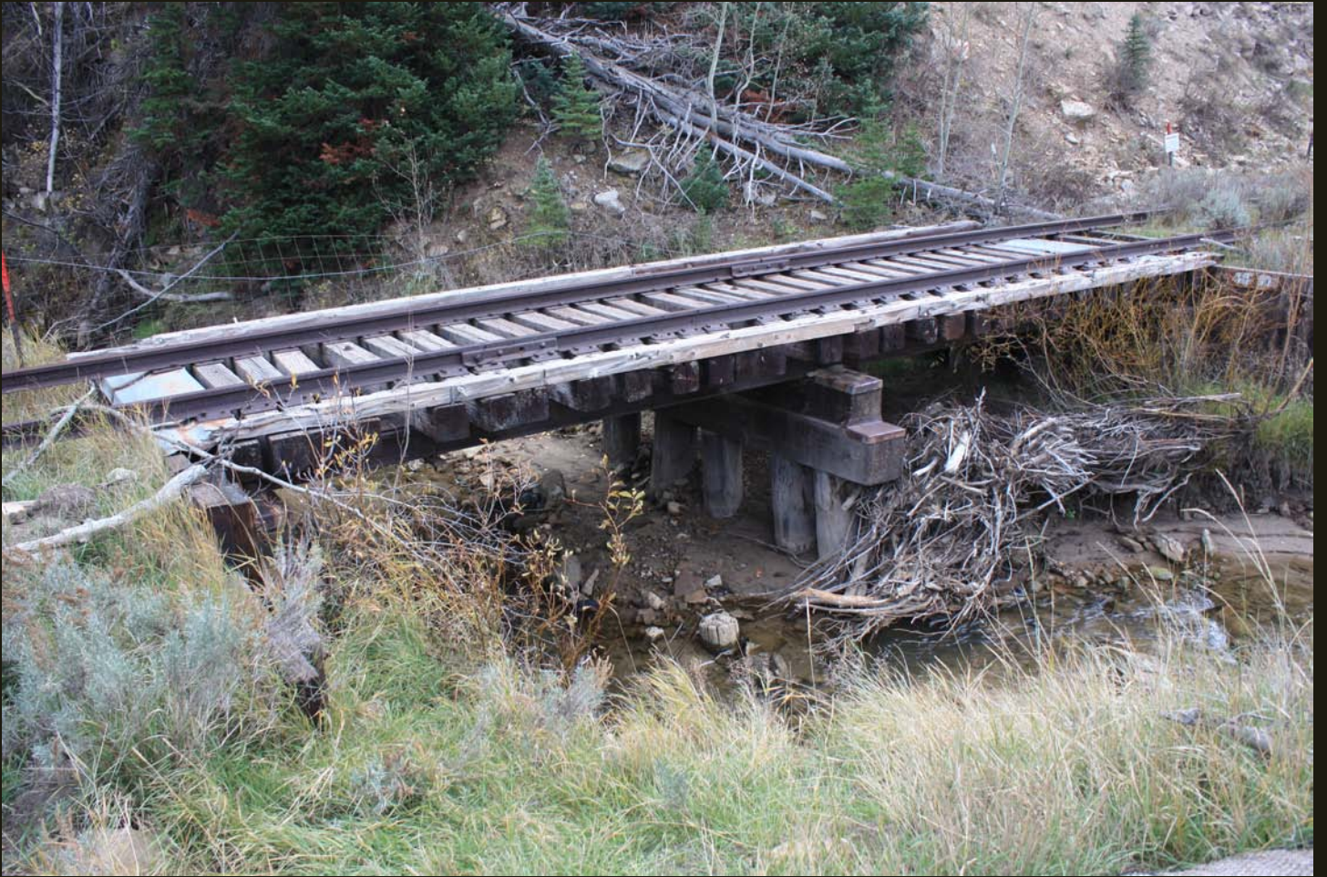
Some of the small trestles are in OK shape.
