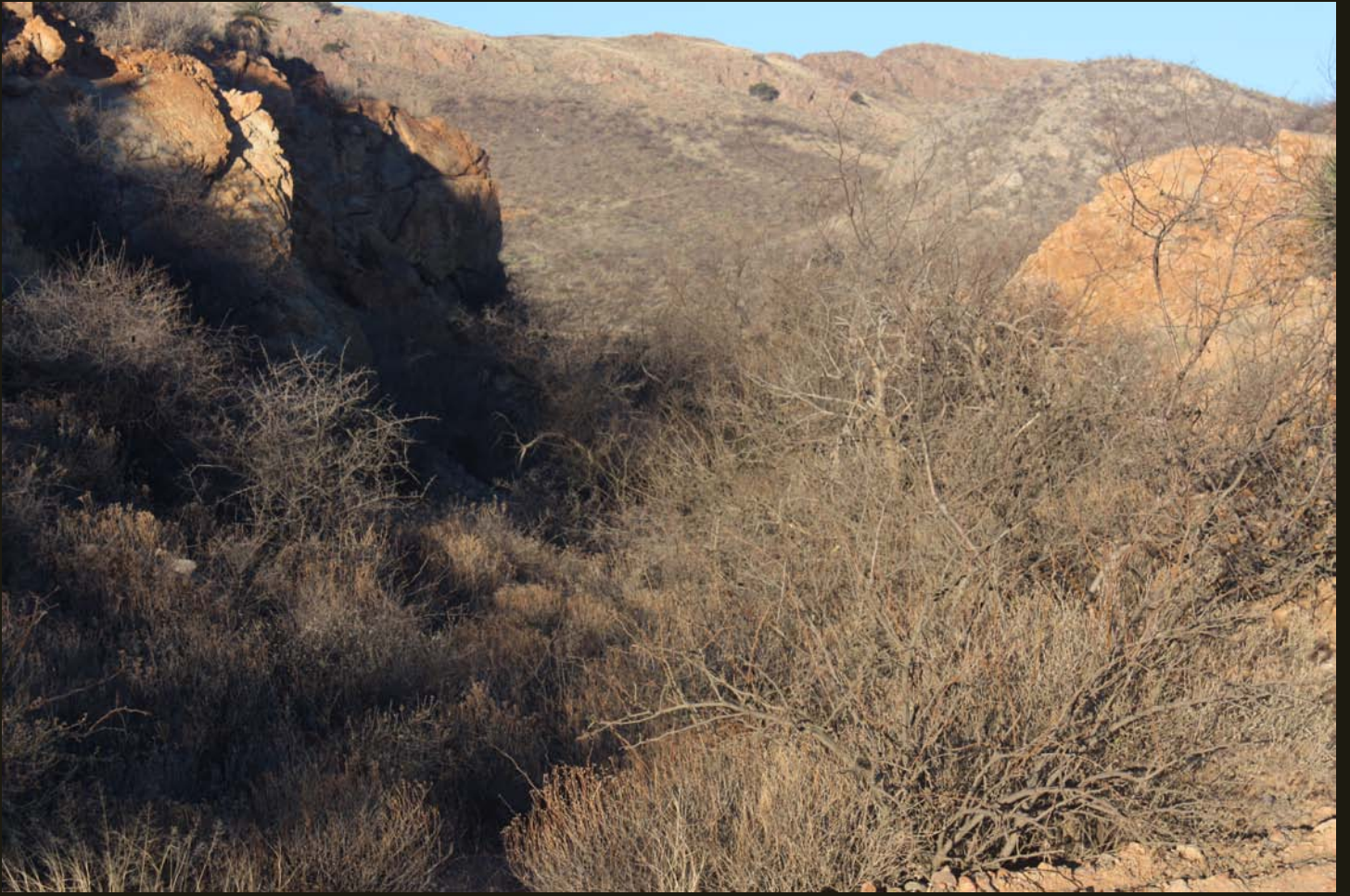
Westward view of the M&C (1908), at the same location as previous, where a significant rock cut was required. The end of the line was less than a quarter mile up from here.
