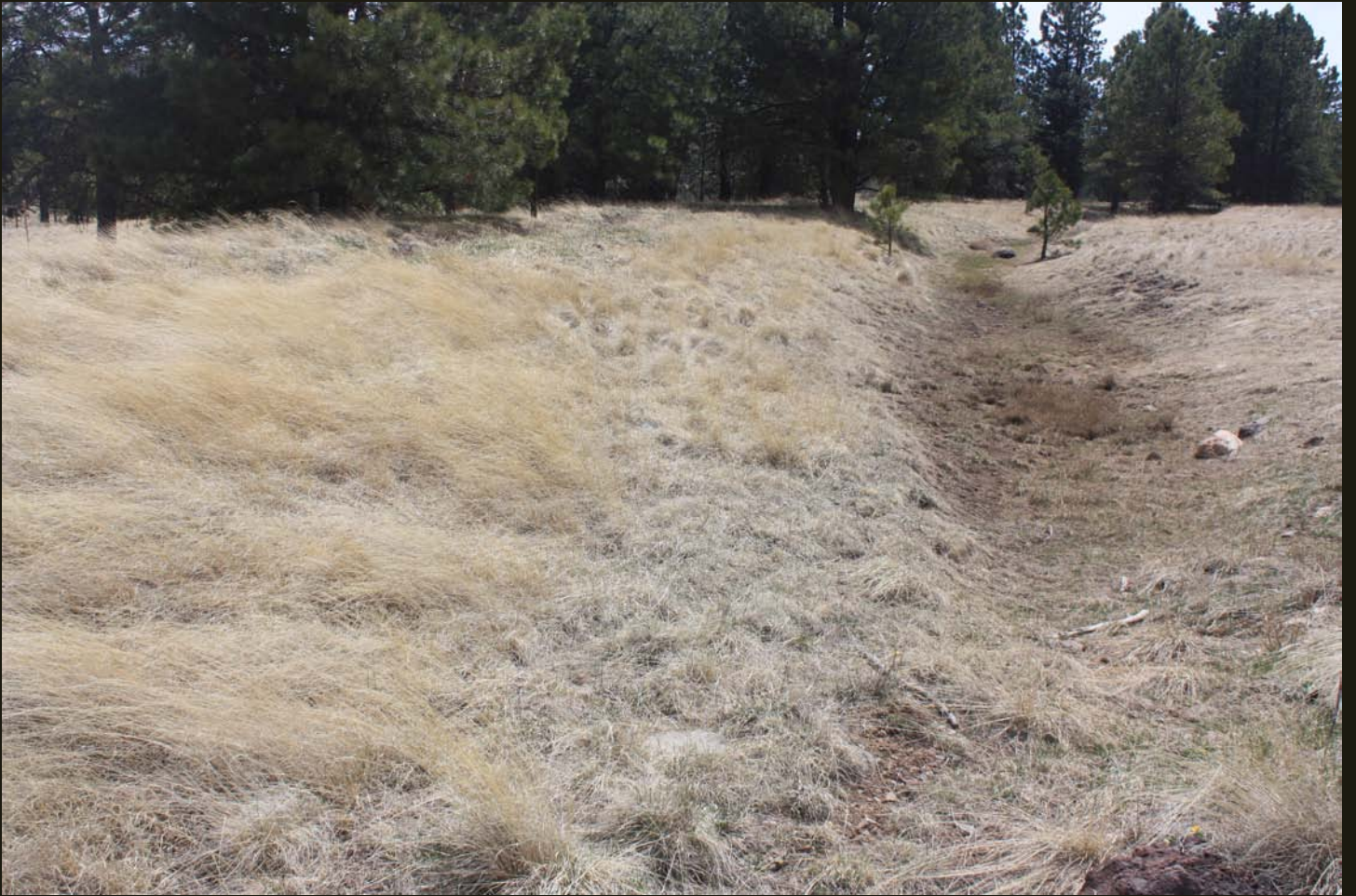
Same location as previous. The ditch provided fill for the SWFI (1944) grade on the left, which curves to the right in the distance.
