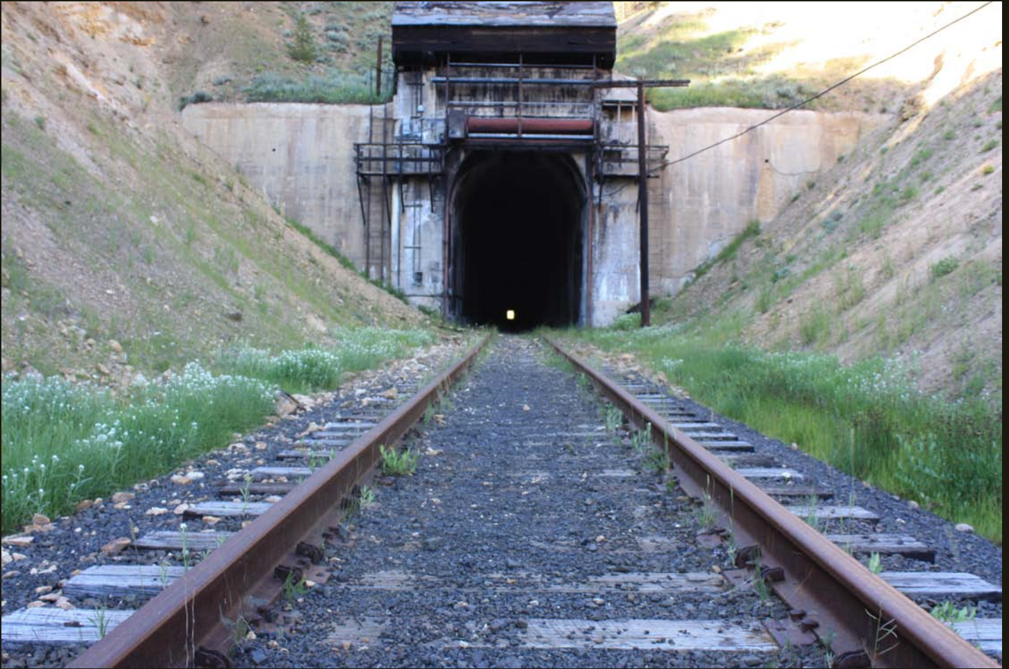
The D&RG Royal Gorge route crosses the continental divide at Tennessee Pass, where a summit tunnel was constructed to lower the grade across the pass.
