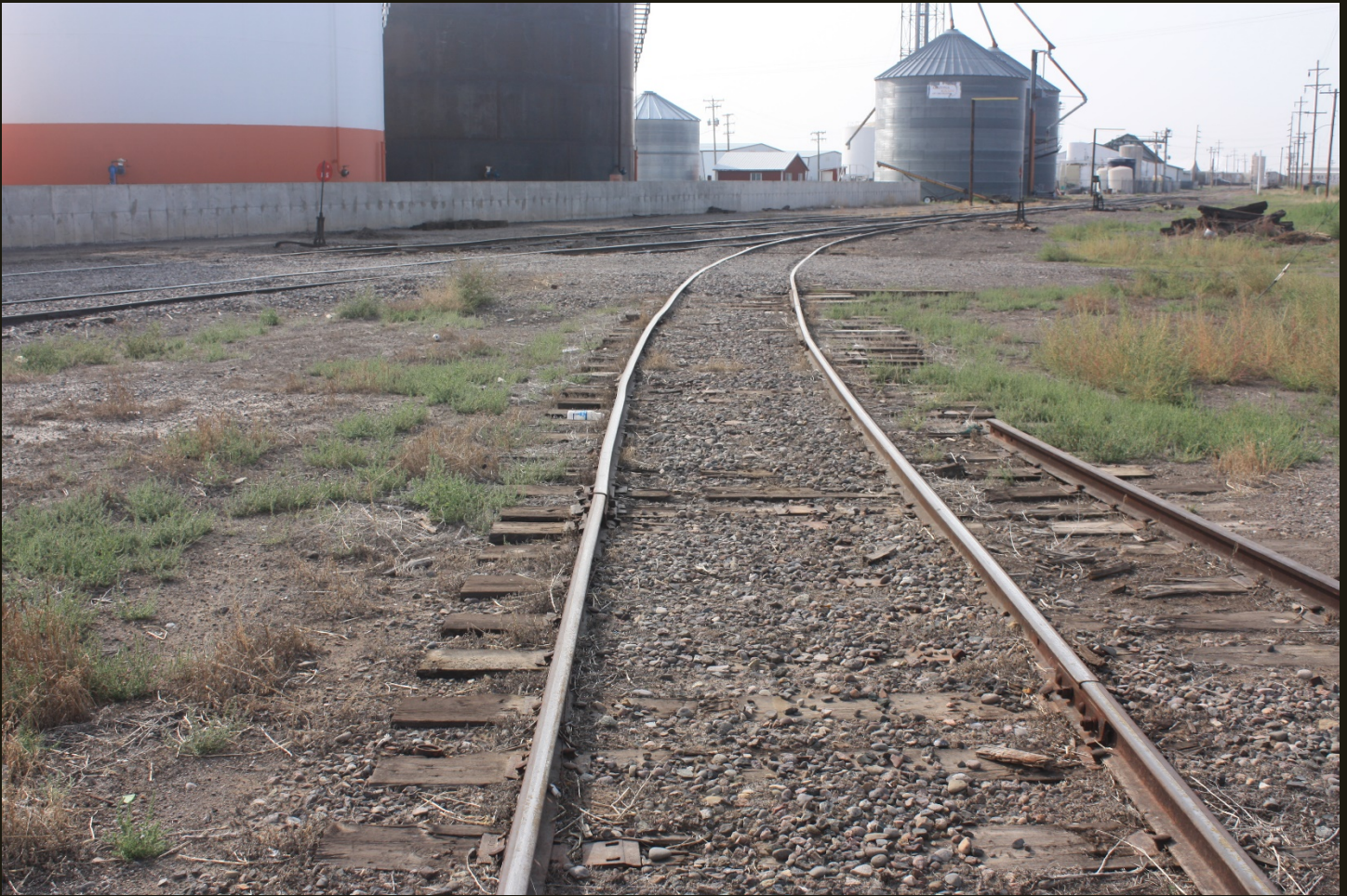
Southeastward view a few steps west of the previous location. The curved track in the foreground is the spur noted in the previous photo; it connects in the distance with the SLC (1913). The rail to the right is another spur, which once connected to the main spur via a now-removed switch.
