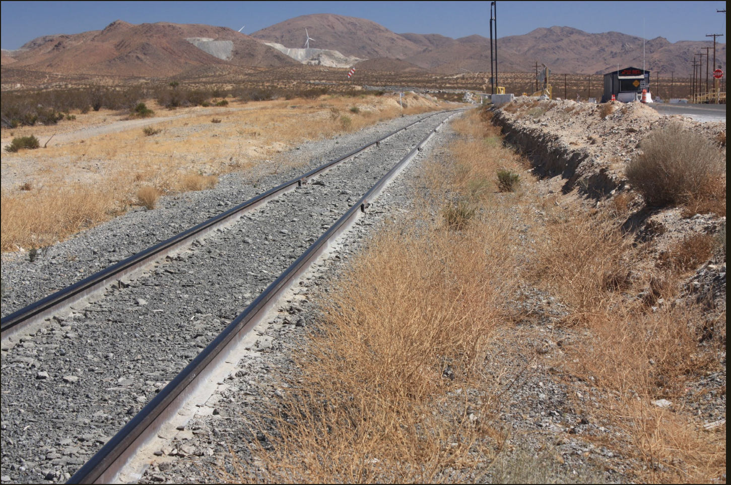
Eastward view of the MN (1916-1951), 2 miles east of the previous location. This part of the MN was built in 1951 and the track ends at the quarry on the hillside. A guard house prevents exploration of the last 5 miles of the MN between here and the Reserve/Black Mountain Quarry.
