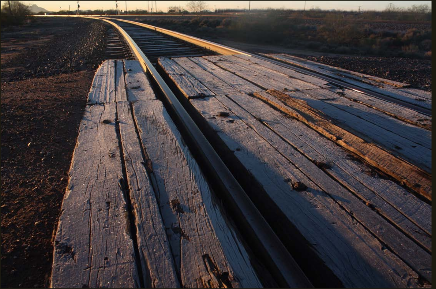
A minor crossing of the eastern branch of the Picacho wye. Picacho Peak is in the far left distance.
