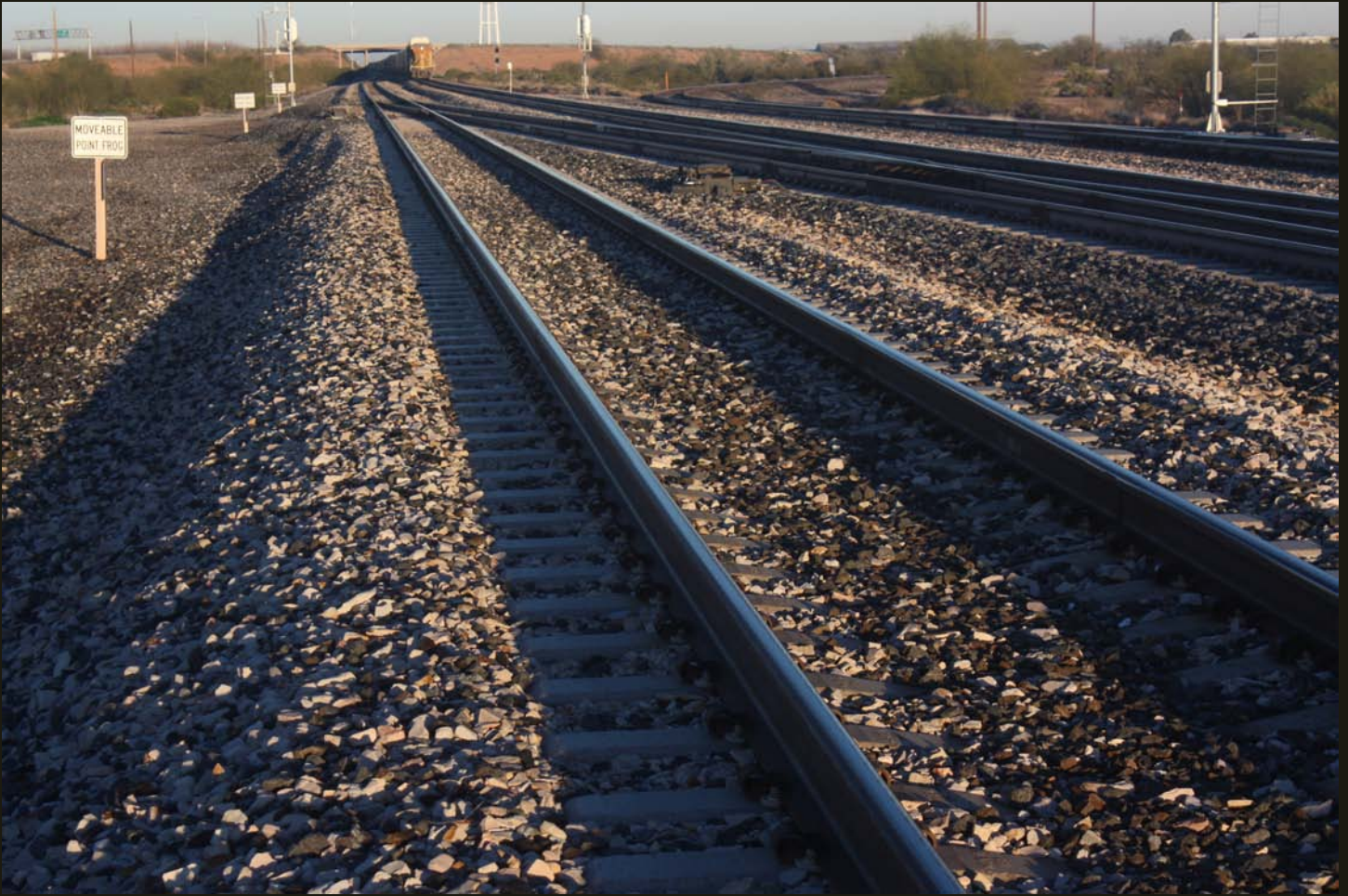
Another northwestward view of the junction of the eastern branch of the Picacho wye. Note the double-track mainline with concrete ties and a crossover track.
