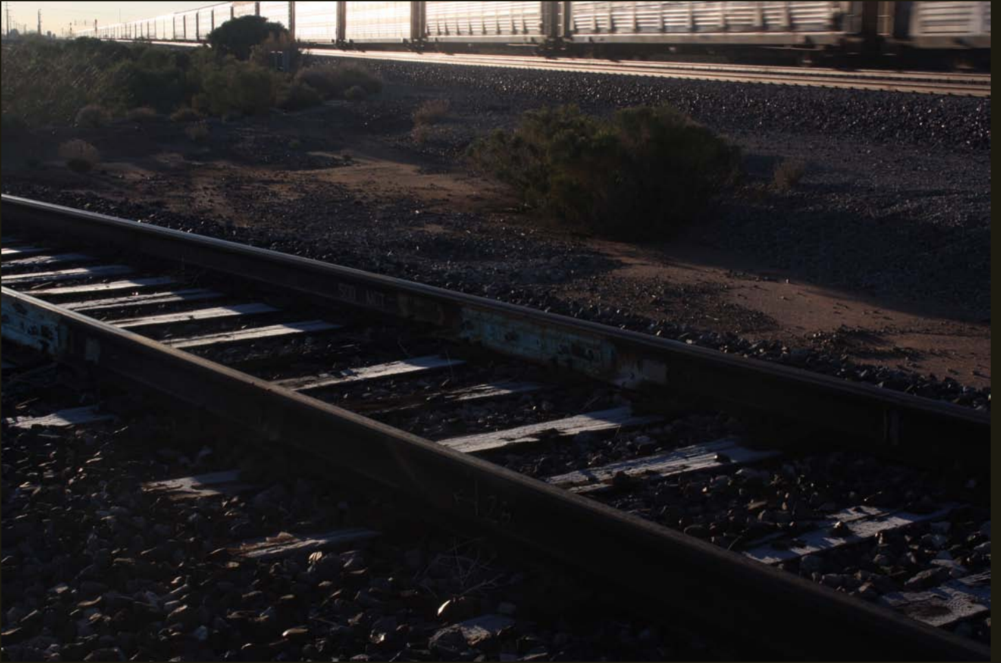
Southward view of the west branch of the Picacho wye, with yet another train speeding by on the busy mainline.
