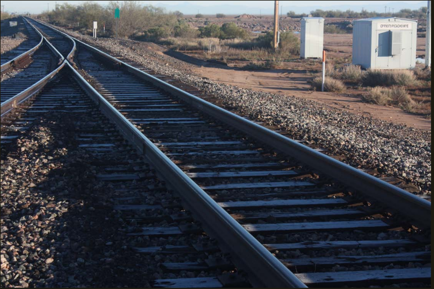
Northward view of the north tip of the Picacho wye. Note that the east (right) branch is straight, needing only to make a long 45^\circ curve to head southeast on the mainline behind the viewer. By contrast, the west (left) branch makes a short 135^\circ turn to head northwest.
