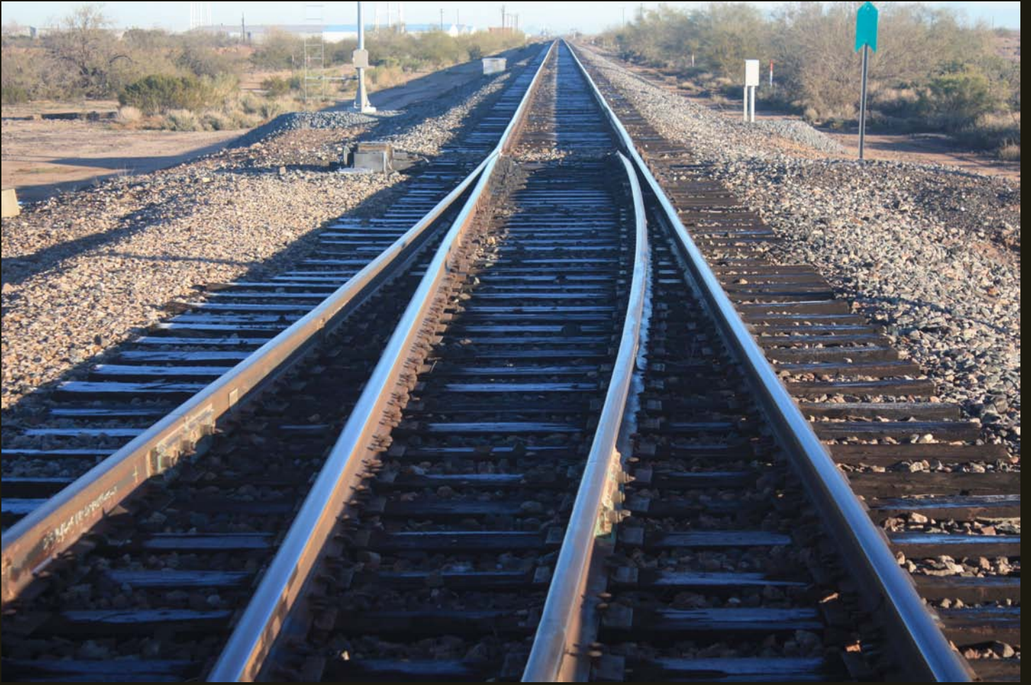
Northward view of the north tip of the of the Picacho wye.
