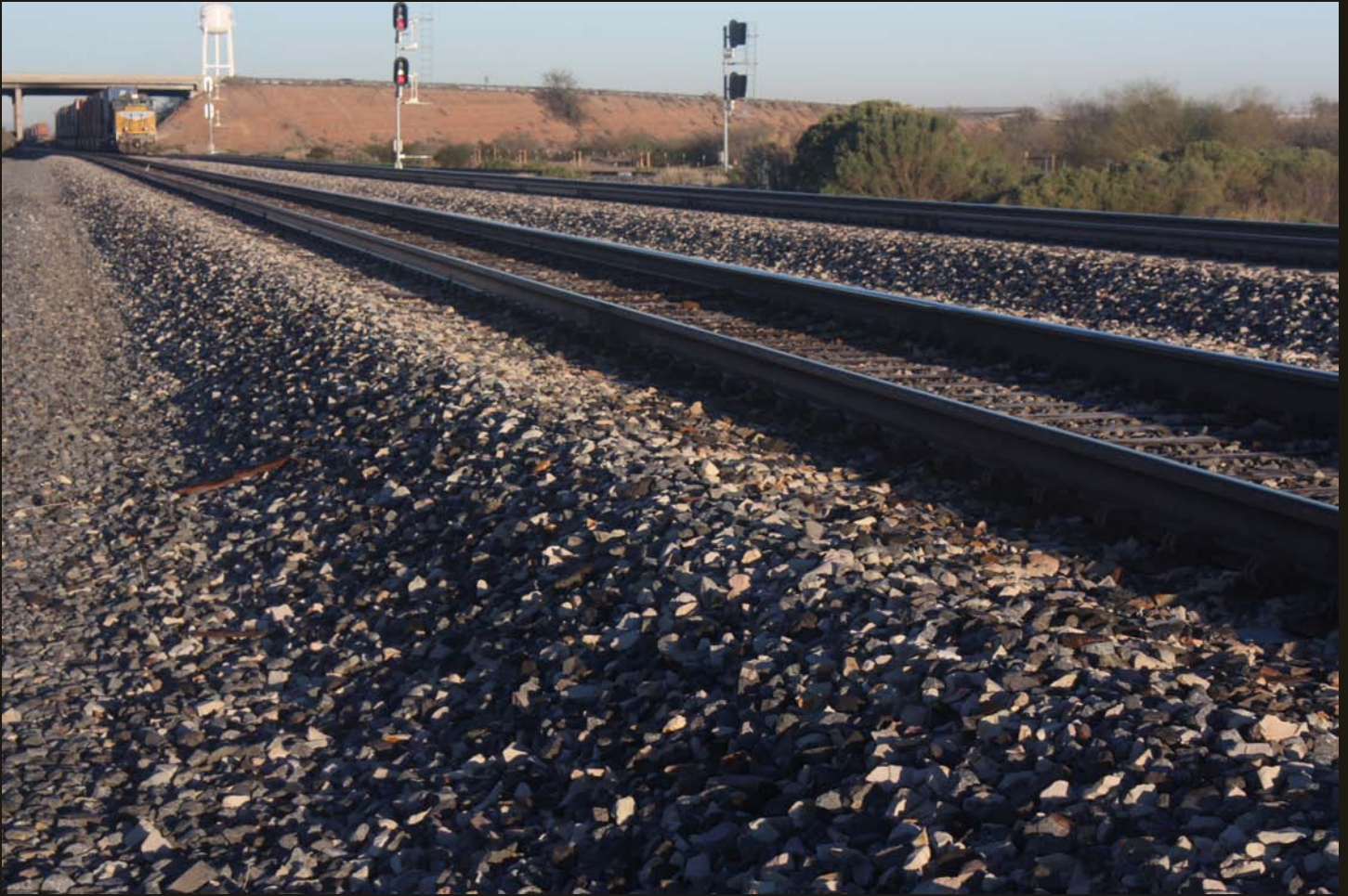
An eastbound train on the mainline and signals for the west branch of the wye, the tracks of which are visible between the two signals.
