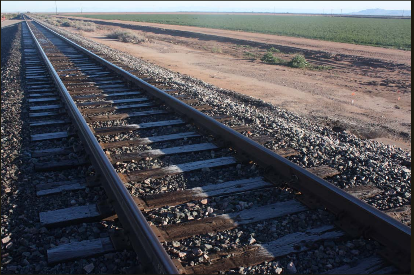
Northward view of the SP (1924), north of the Picacho wye. Note the irrigated fields on the flat lakebed. Note also the very straight track and easy build afforded by the flat topography, which continues north to Magma and Phoenix.
