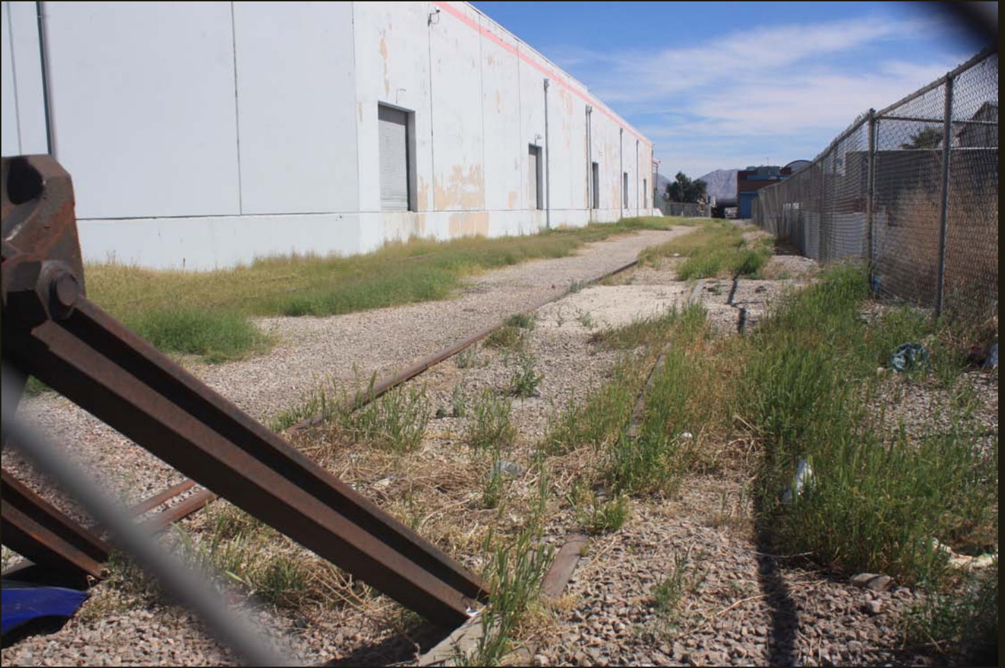
Westward view of the end-of-track of the pre-1952 industrial spur, 3,500 feet west of its junction with the SPL&SL/LA&SL/UP mainline.
