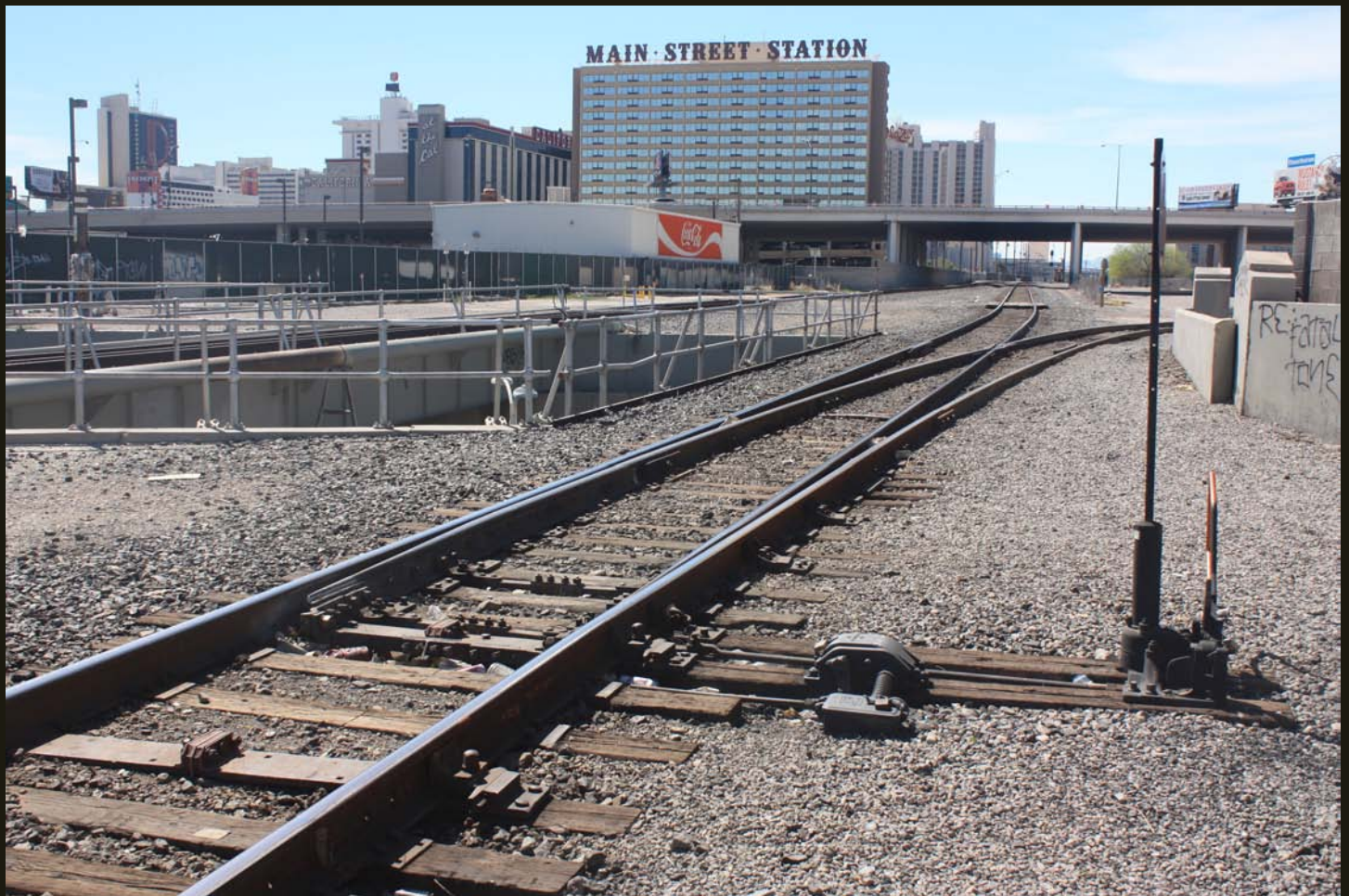
Southwestward view of the SPLA&SL (1905), same location as previous, showing the mainline (left), the siding (foreground), and switch to an industrial spur to the right (west). The spur is present on a 1952 topo map and we'll explore that spur a little more. The skyline of downtown Las Vegas looms above all. I suspect the Main Street Station Hotel refers to the SPLA&SL Las Vegas Station, which is long gone.
