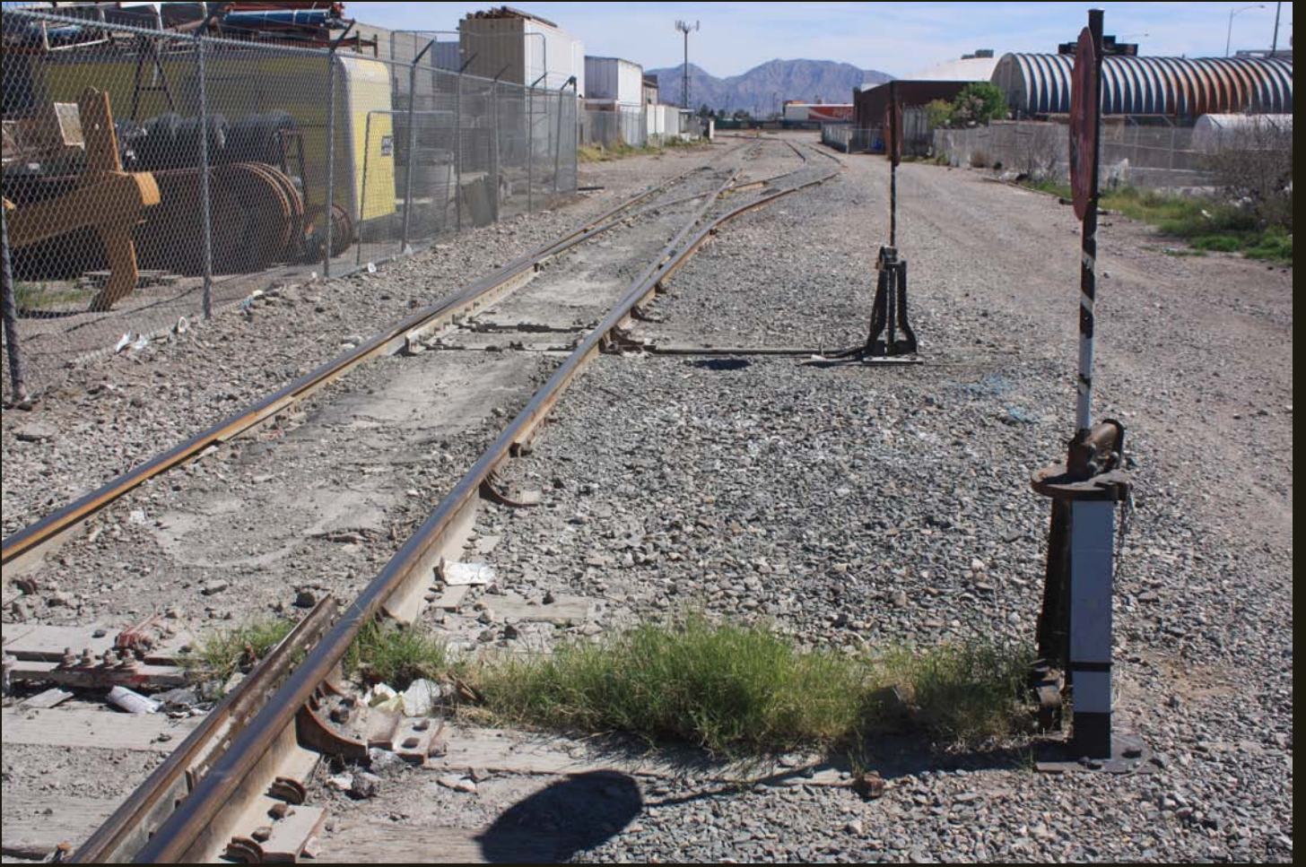
Eastward view of the pre-1952 industrial spur; a short siding is in the distance and a switch for another siding is in the foreground.
