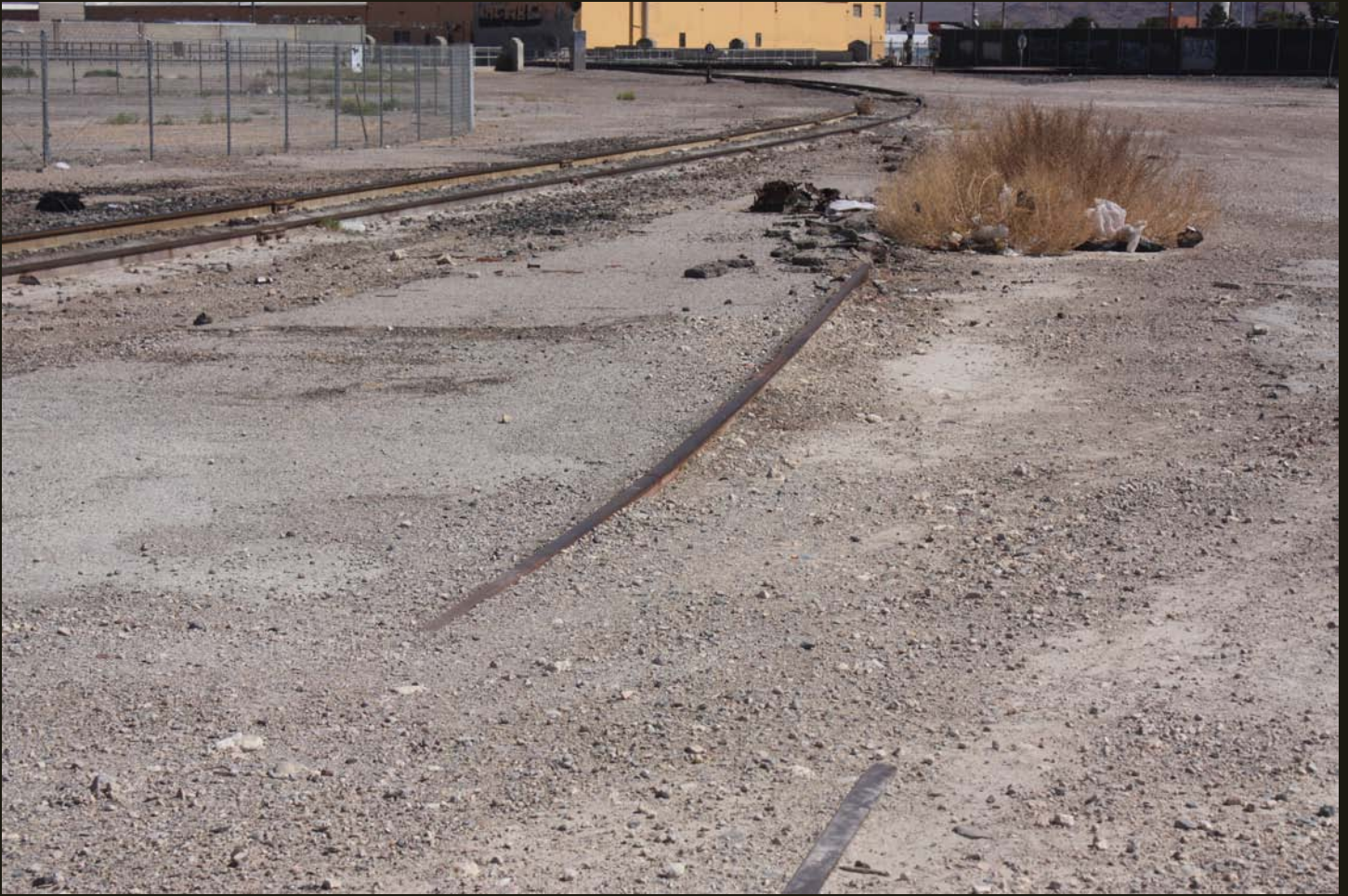
Northeastward view of the pre-1952 industrial spur; the SPLA&SL (1905) is in the distance. Old track in the foreground hints at possible additional spurs.
