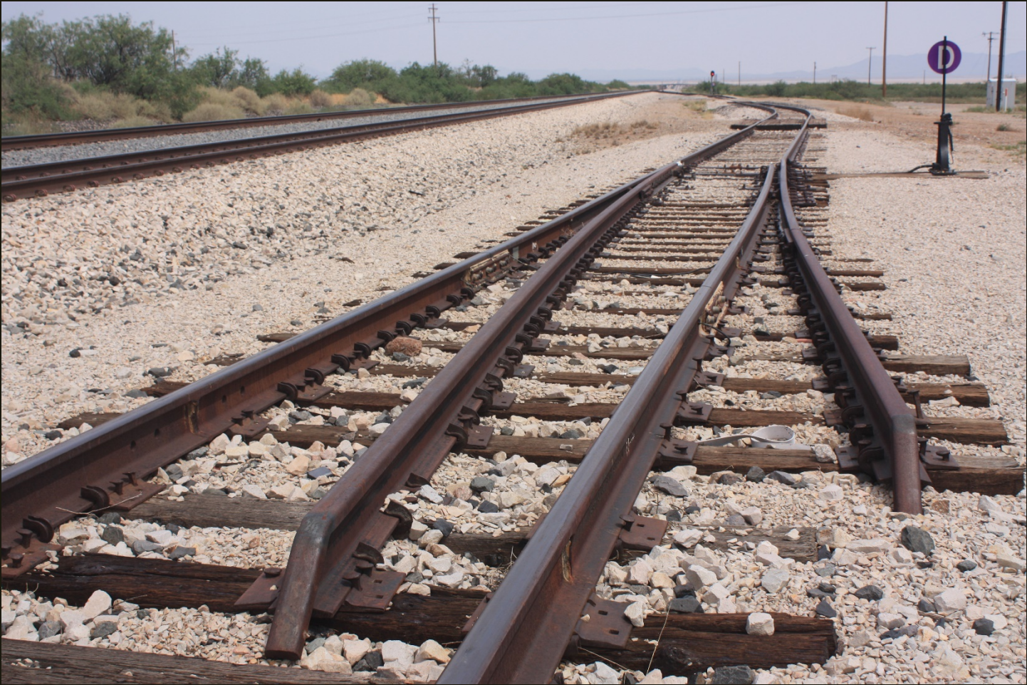
Northeastward view at the same location as previous with the same derail switch in the foreground. The red light at the far end of the siding is an identical derail switch facing the other way.
