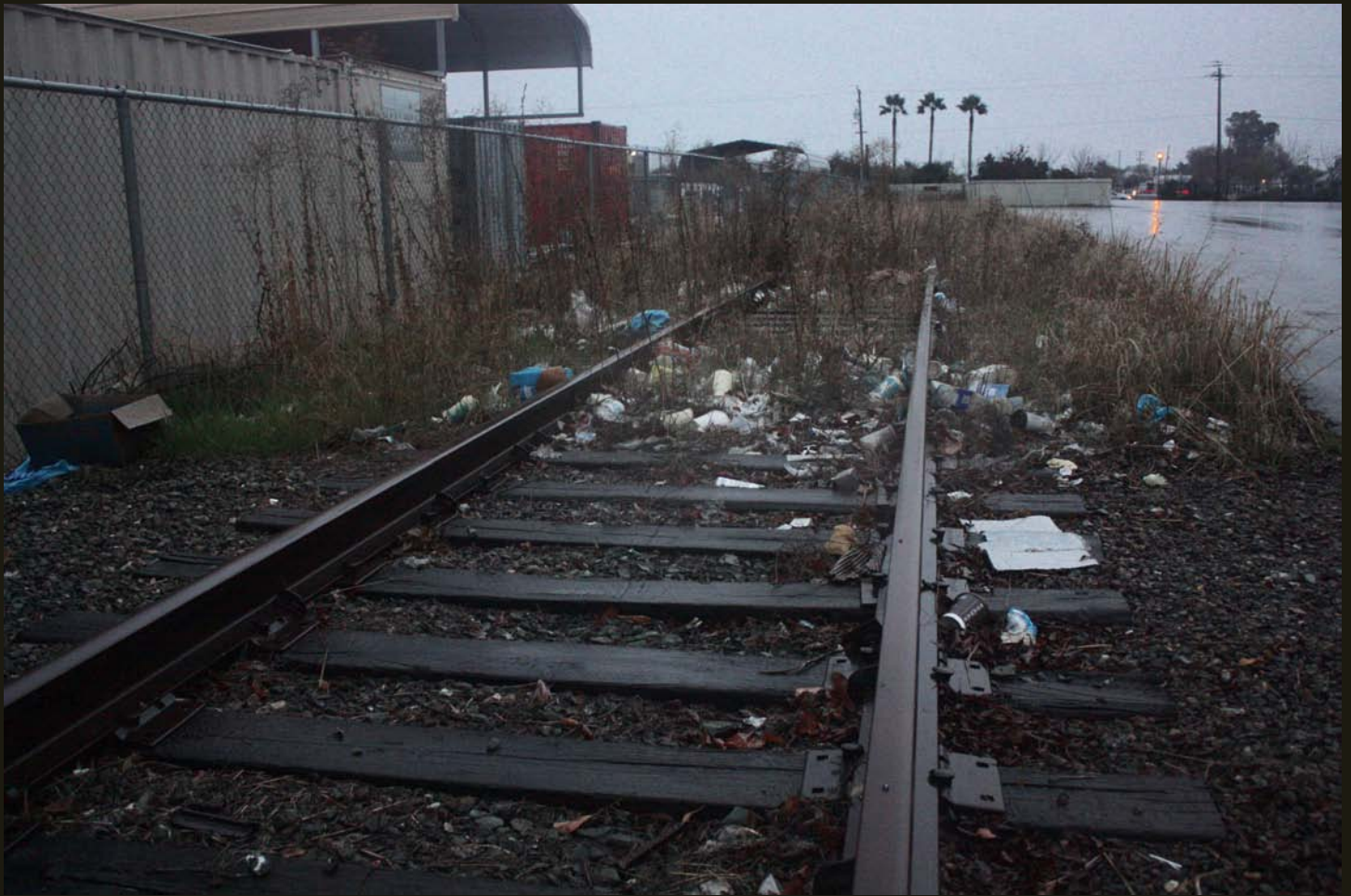
Southeastward view of the SP West Side Line (1891), the main line probably ran in the flat area to the right. The track ends at a loading facility in the distance, which now is the end-of-track of the California Northern.
