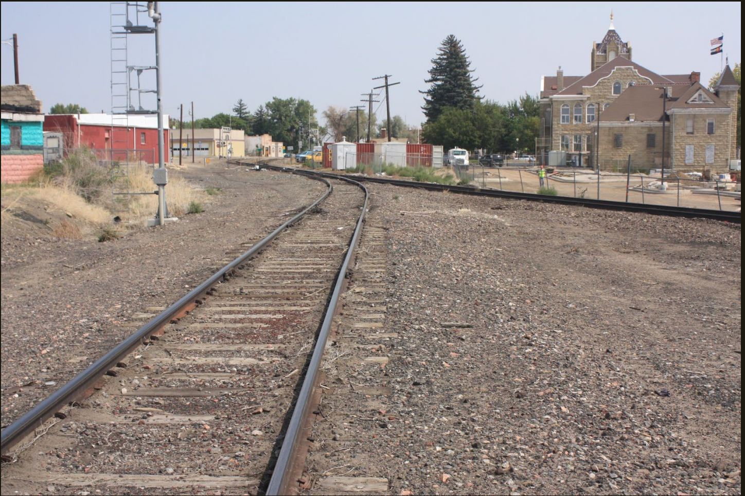
Now we are back at the junction looking northeastward at the bolted rails of the D&RG San Juan Extension (1878n) in the foreground and the welded rails of the UPD&G (1895) curving to the right (south). The historical building on the right is the Huerfano County Courthouse.
