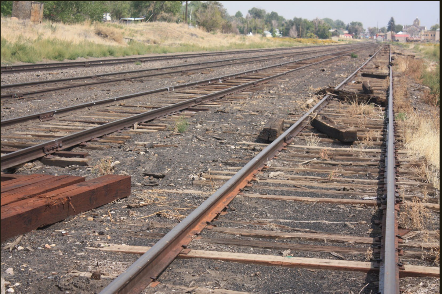
Northeastward view 2,500 feet southwest of the previous location. The D&RG San Juan Extension (1878n) mainline is the second track from the right. Barely visible in the right distance are the three parked tanker cars and the Huerfano County Courthouse. Also in the distance, the mainline has split off one siding to the south (right) and two to the north (left), thus four tracks in this view.
