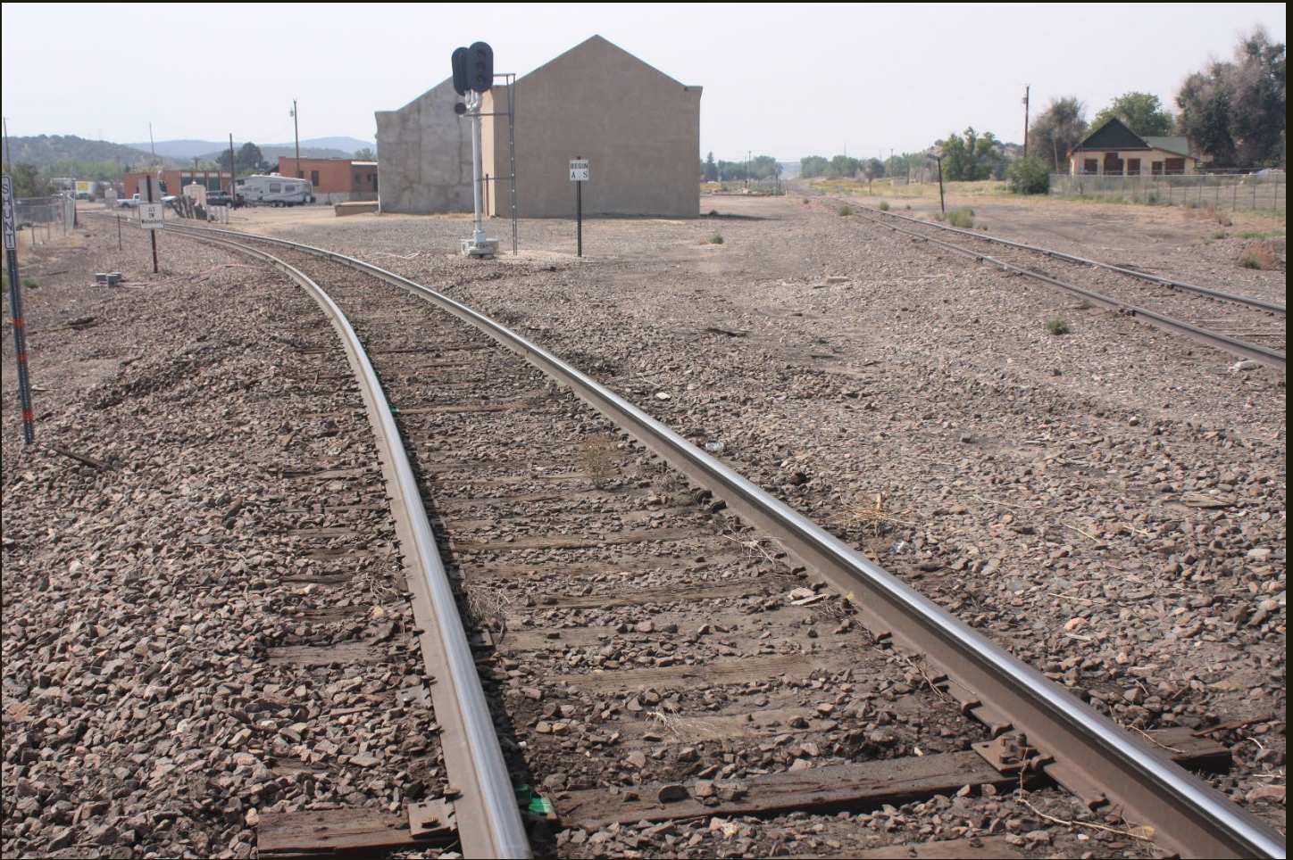
Southwestward view at the same location as previous. The welded rail of the UPD&G (1895) is in the foreground and the bolted rails of the D&RG San Juan Extension (1878n) run straight on the right. The abandoned building between the tracks is railroad-related, but I could find no information on its history.
