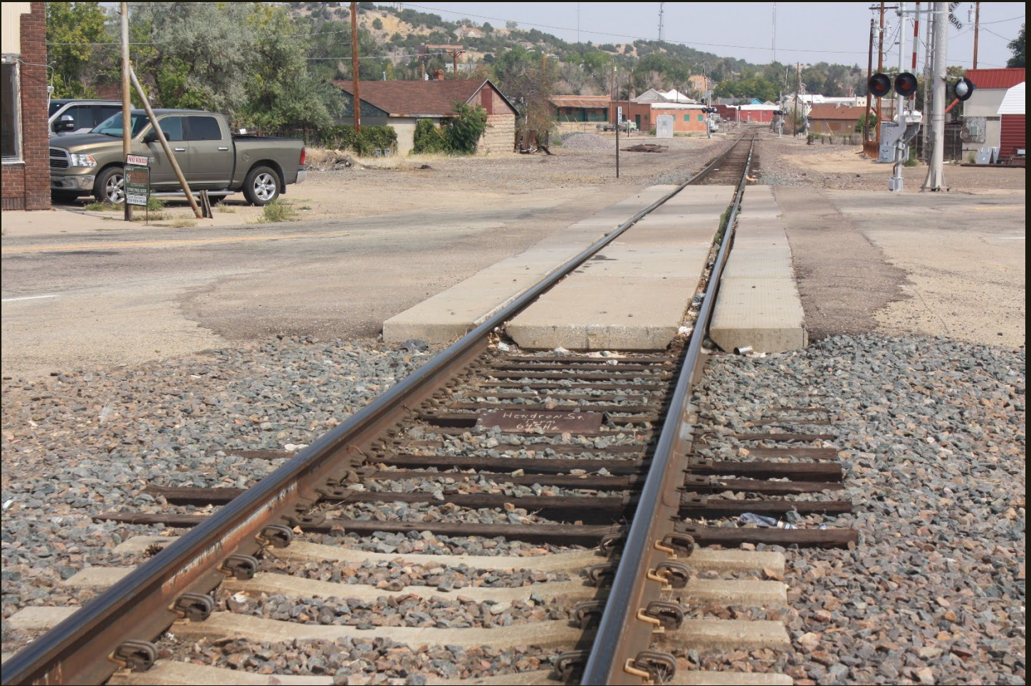
Northeastward view of the UPD&G (1895) about 1,600 feet southwest of the previous location. The curved track in the distance is the location of the junction with the D&RG San Juan Extension (1878n). Note the transition from wooden ties to concrete in the foreground.
