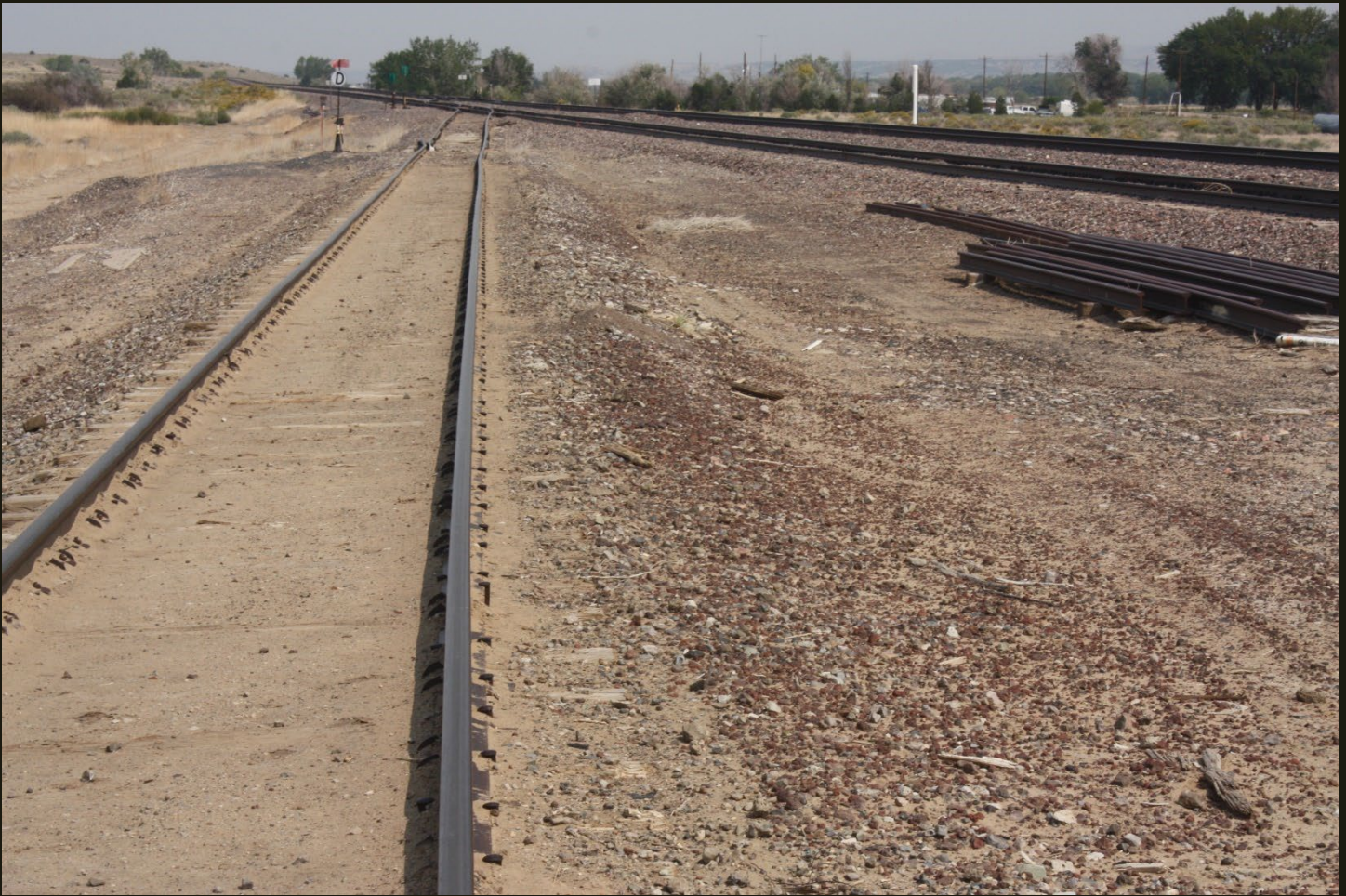
Eastward view of the D&RGW-C&S (1911) at the same location as previous. The line in the foreground is a siding that connects in the distance to the double-track mainline via a switch and, barely visible to the left of the switch, a crossover track to the farther of the two mainline tracks.
