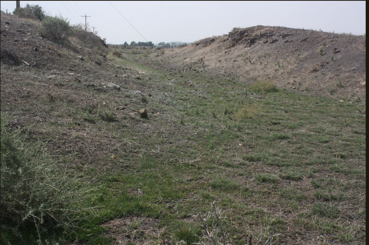
Southwestward view of the same cut grade for the D&RG San Juan Extension (1878n).
