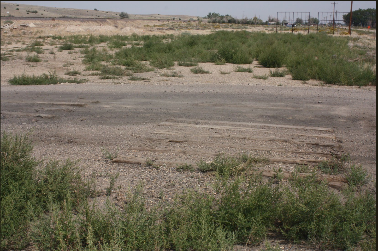
Northeastward view of the abandoned D&RG San Juan Extension (1878n), 2 miles west of the previous location and 0.5 miles east of the intersection with the D&RGW-C&S (1911) at Walsenburg. The ties in the foreground are remnants of the D&RG San Juan Extension (1878n), which was standard-gauged in 1894 and abandoned sometime between 1917 and 1936. The track in the left distance is the D&RGW-C&S (1911) Southern Joint Line.
