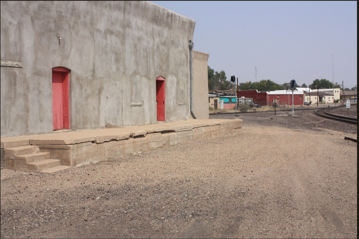
Northeastward about 100 feet west of the previous location, with the same split of the UPD&G (1895) curving to the right and the D&RG San Juan Extension (1878n) running straight to the left (behind the railroad-related building with the red doors). From here we'll explore the UPD&G (1895) first.
