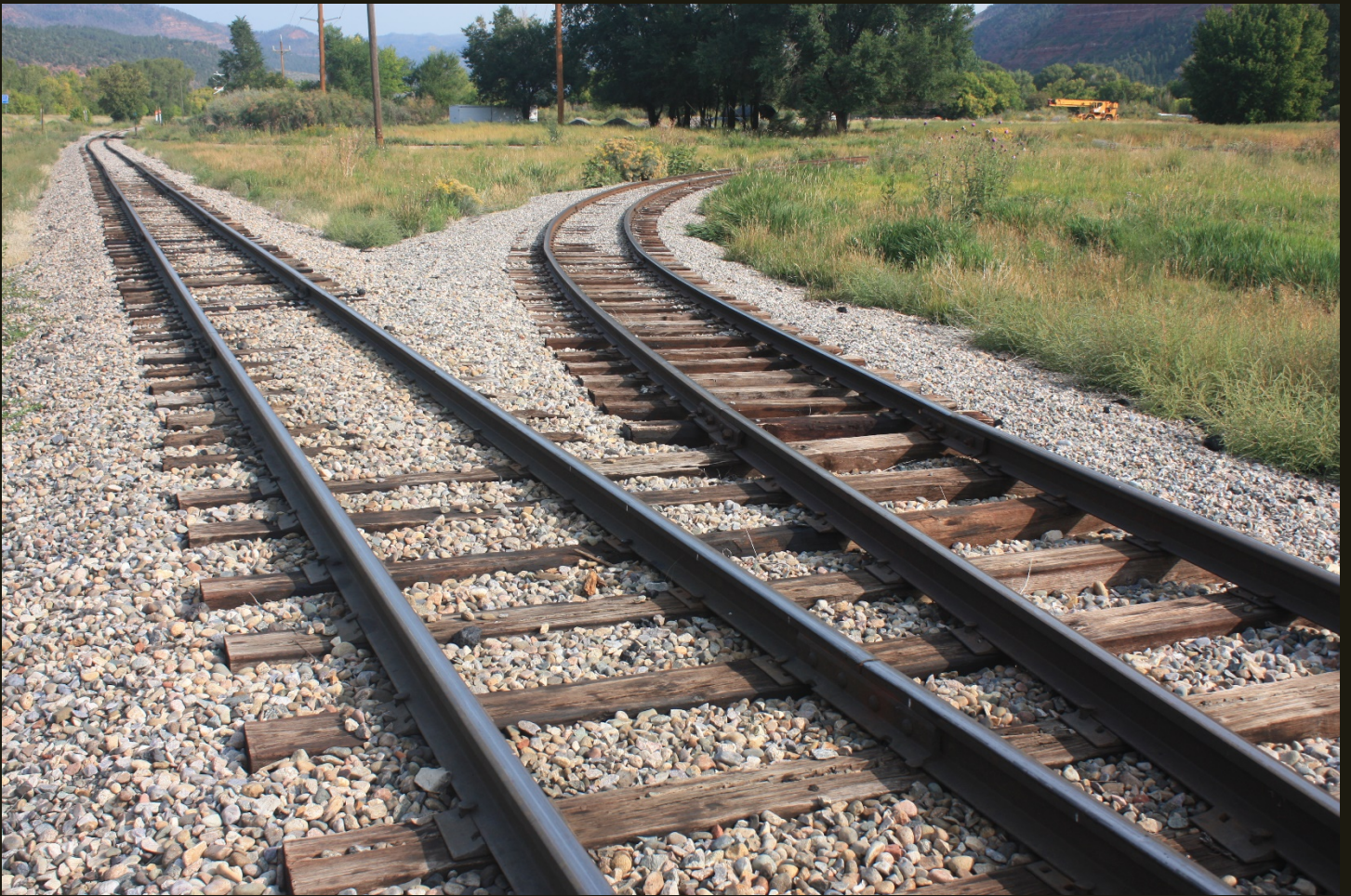
Northward view of the D&RG Silverton Branch (1882n) and the D&SNGRR-built wye at the same location as previous.
