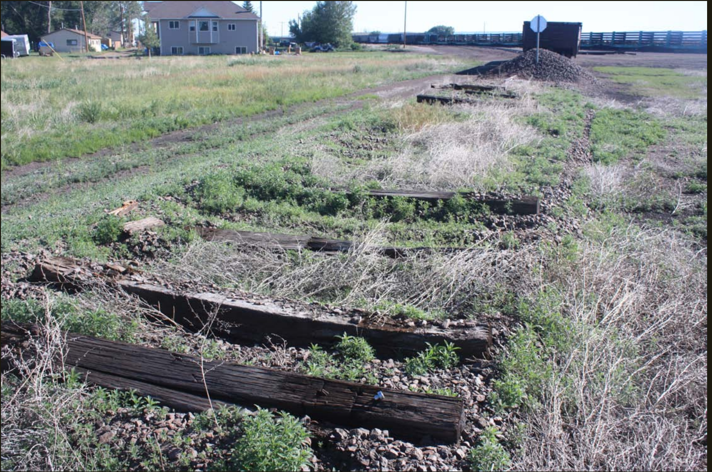
The cars just beyond the gravel pile and stop sign are the two cars seen stored in the previous photo on the only rails that remains on the LHP&P grade. Note LHP&P ties left in place in the foreground.
