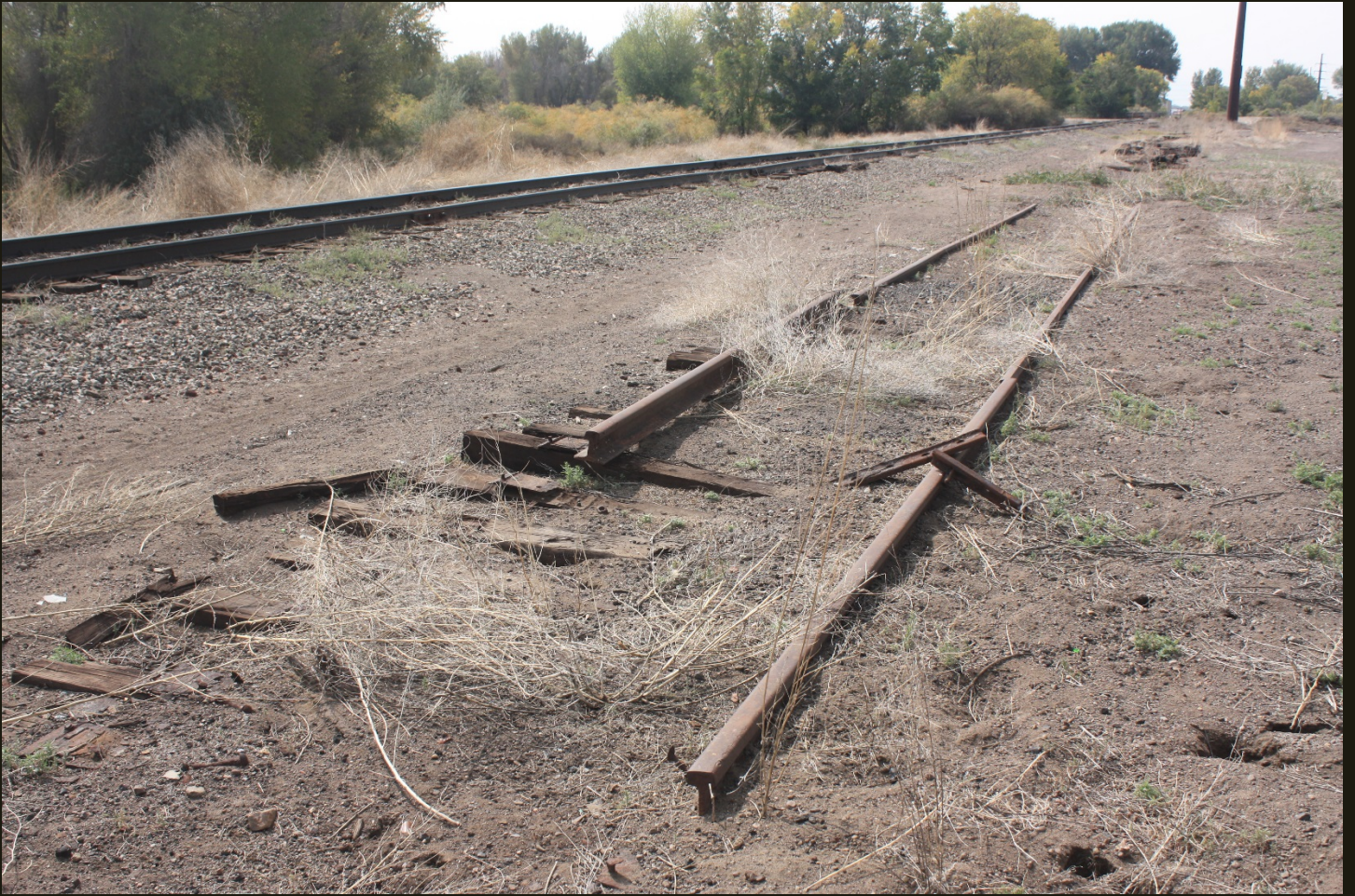
Southwestward view of the D&RG San Juan Extension (1878n) at the same location as previous. Both rails of the abandoned siding are still present here. Note the line of loose ties just beyond the intact rails.
