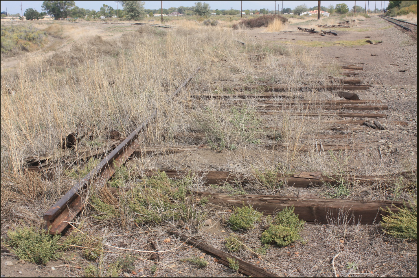
Eastward view of the D&RG San Juan Extension (1878n) 350 feet west of the previous location. The intact track in the right distance is the San Juan Extension mainline. The track with one rail in the foreground is the west branch of the wye for the Hooper Spur. Note the very long ties in the foreground, much longer and needed for two rails. This was the switch where the siding, indicated by the line of ties to the right of the utility poles, joined the west branch of the wye.
