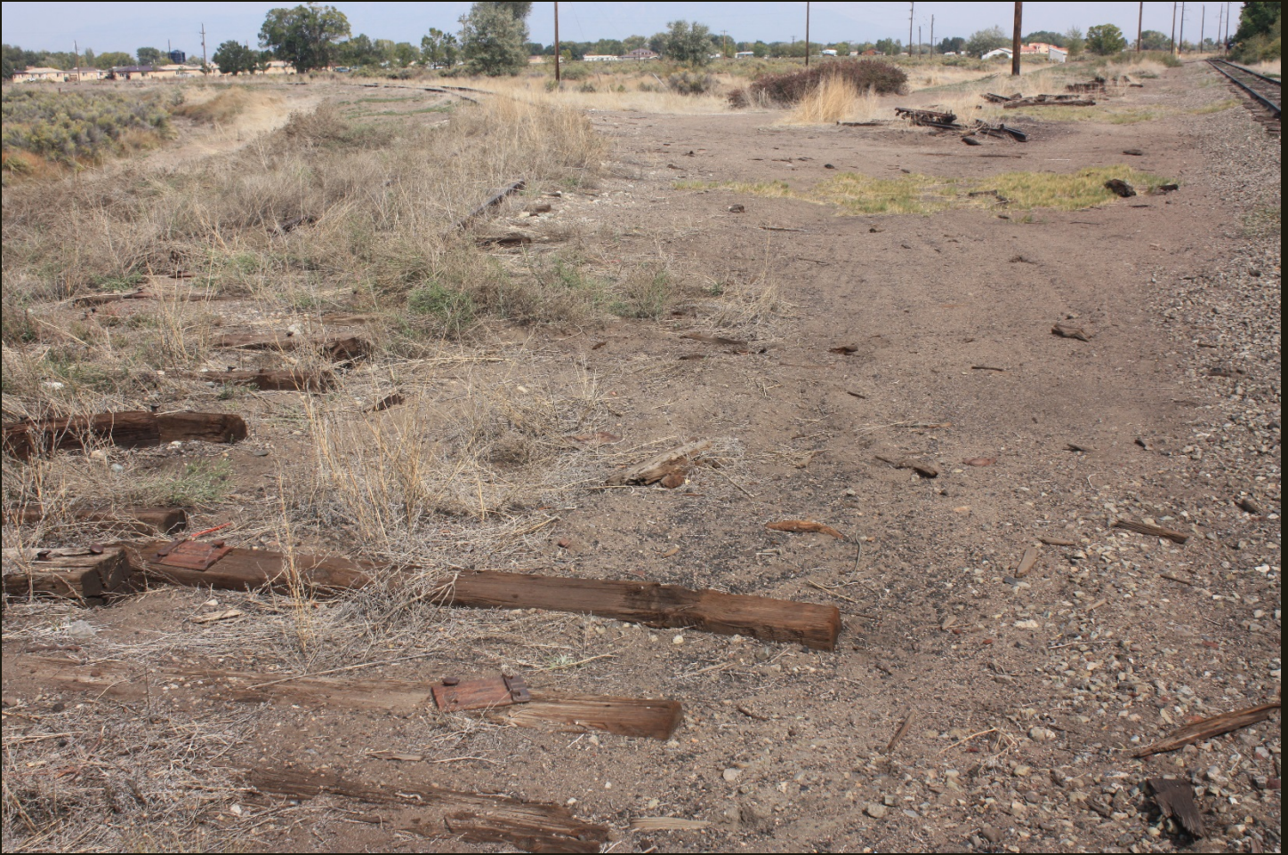
A slightly different eastward view just a step or two south of the previous location. The intact track in the right distance is the San Juan Extension mainline and the curved track to the left is the west branch of the wye for the Hooper Spur. The long ties in the foreground once supported the switch where the siding, indicated by the line of ties to the right of the utility poles, joined the west branch of the wye.
