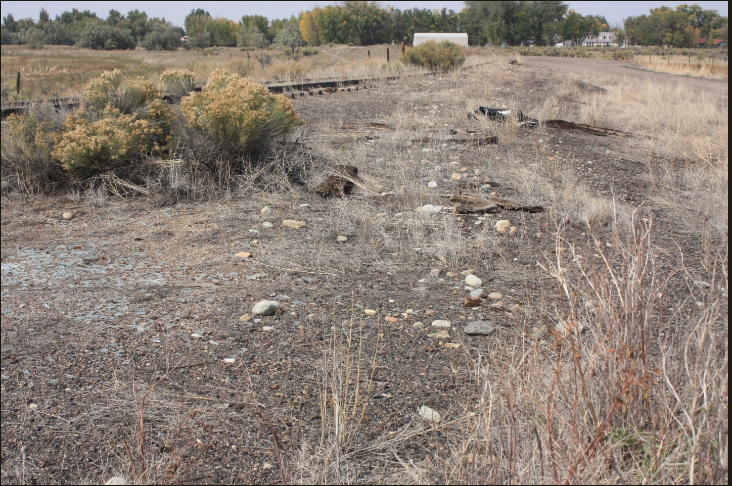
Northwestward view, 450 feet northeast of the previous location. The gravel in the foreground is the east branch of the wye for the Hooper Spur. The track in the middle distance is the west branch of the wye. The north tip of the wye was located at about the farthest right track that is visible. For future reference, note the white building beyond that of the wye.
