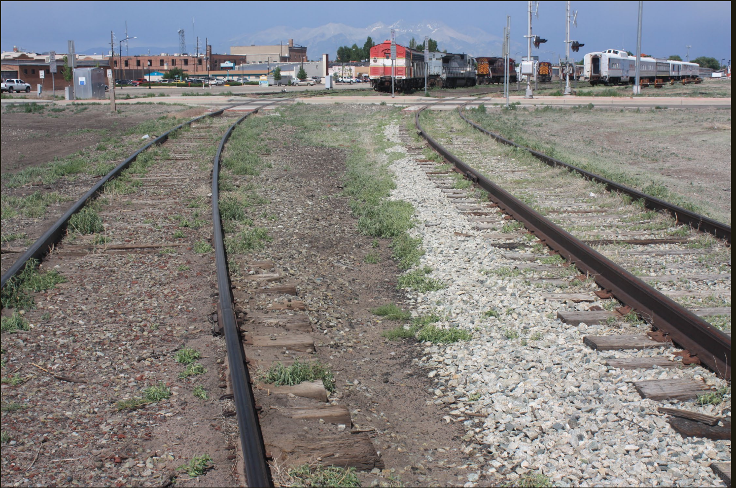
Northeastward view 200 feet southwest of the previous location. The un-rusted (active) track on the left is the mainline of the D&RG San Juan Extension (1881n), the rusted track on the right is a siding that joins the mainline behind the viewer, and the same diesel engine in red Carolina Southern livery is on a siding between the two. The D&RG Creede Branch (1883n) is barely visible in the upper left.
