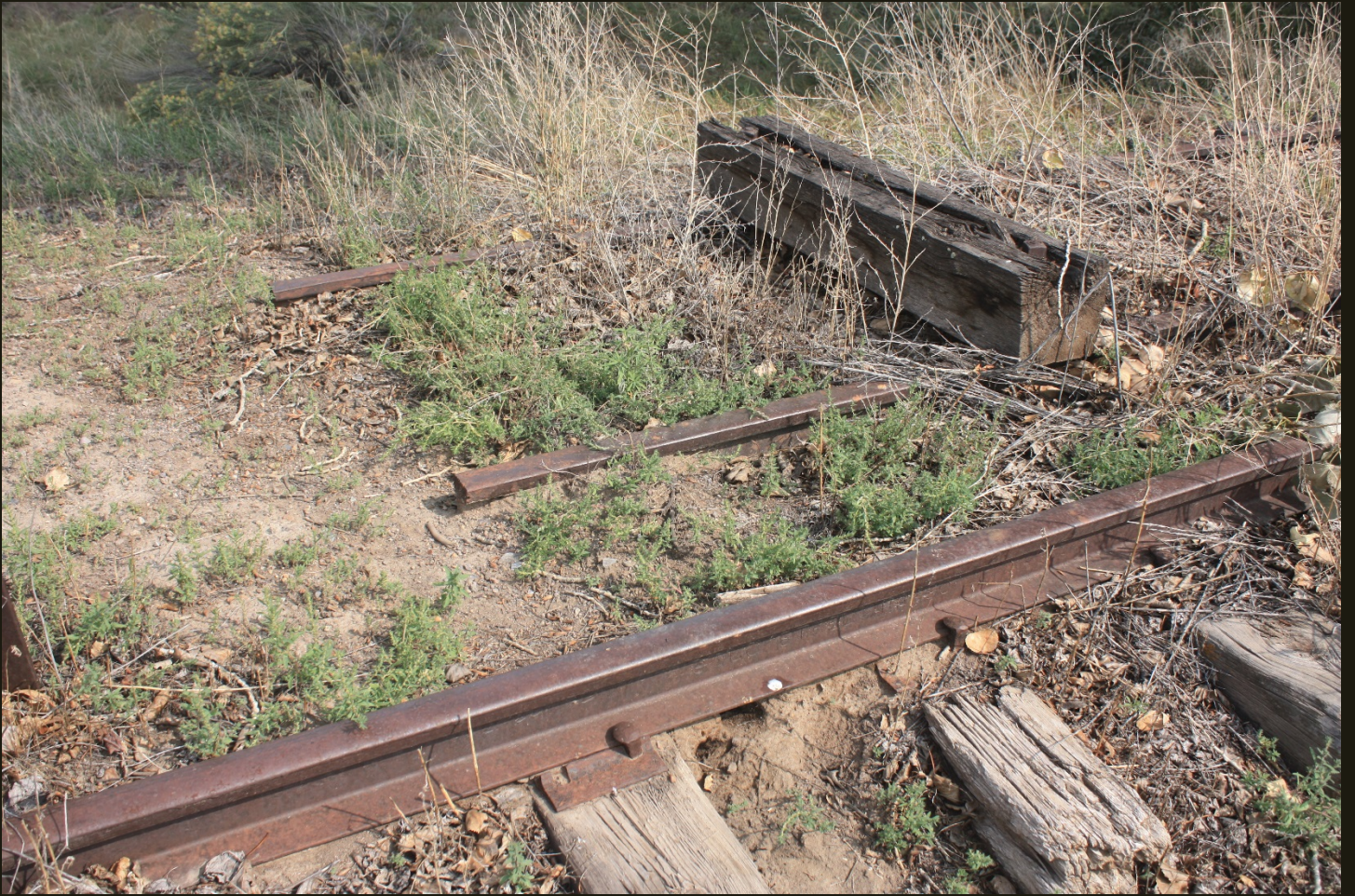
Closer view of the dual gauge track at the north end of the remaining track of the Hooper Spur. Note the same block of wood as in the previous photo.
