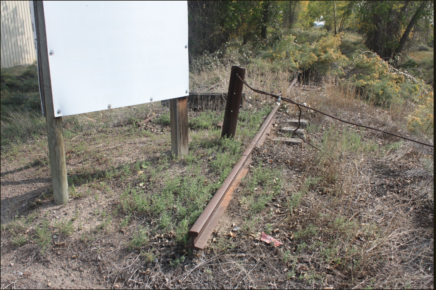
Southward view, 1,600 feet north of the previous location, at the north end of the remaining track of the Hooper Spur (former D&RG Valley Line 1890n). Note the block of wood on the track behind the white sign. Look carefully and you'll see that that block of wood is on two tracks; this is dual gauge track!
