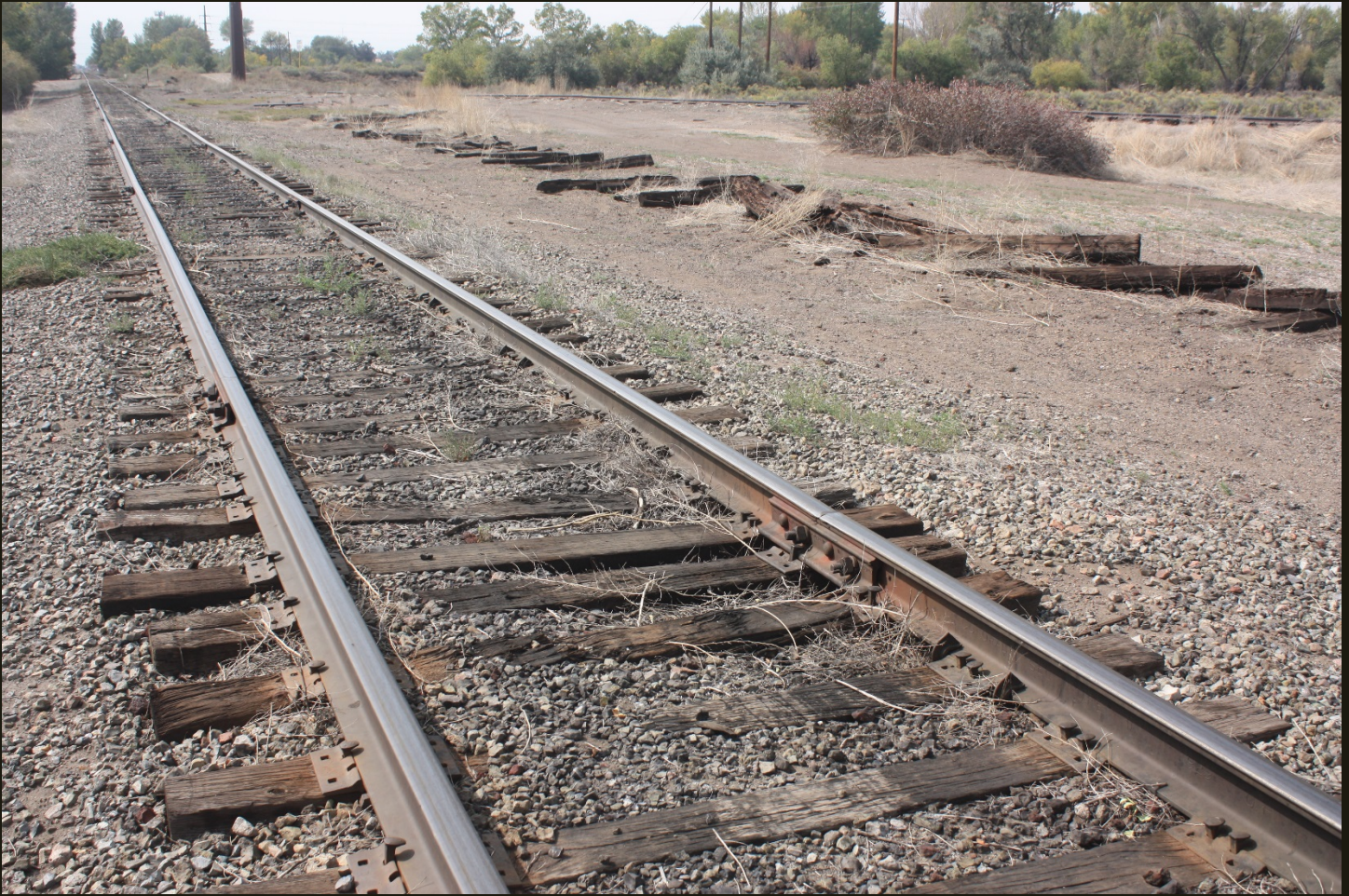
Westward view of the D&RG San Juan Extension (1878n) 150 feet west of the previous location. The line of loose ties is the same as in the previous photo and are remnants of the abandoned siding for the wye for the Hooper Spur (former D&RG Valley Line 1890n). The west branch of the wye is the track just beyond the line of loose ties.
