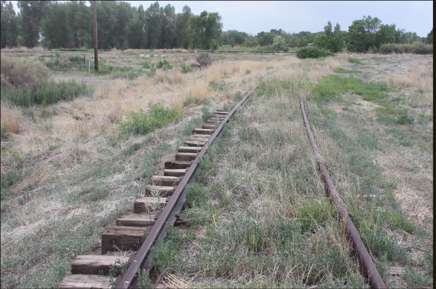
Southwestward view of the west branch of the wye for the Hooper Spur, 500 feet southwest of the previous location. The D&RG San Juan Extension (1878n) is in the distance.
