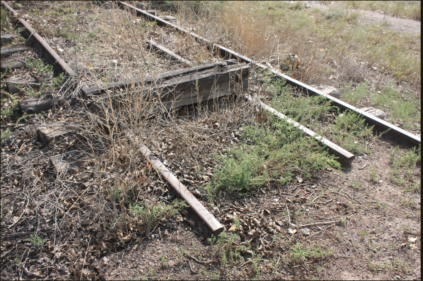
Another view of the dual gauge track at the north end of the track of the Hooper Spur (former D&RG Valley Line 1890n). In this view we can see the south (farther) end the center rail, which may have been the south end of narrow gauge operations, and the block of wood may have been used to prevent narrow gauge rolling stock from going south of this point, which would cause a derailment. I am not sure why any dual gauge track remains, because the center rail was reportedly removed in 1951.
