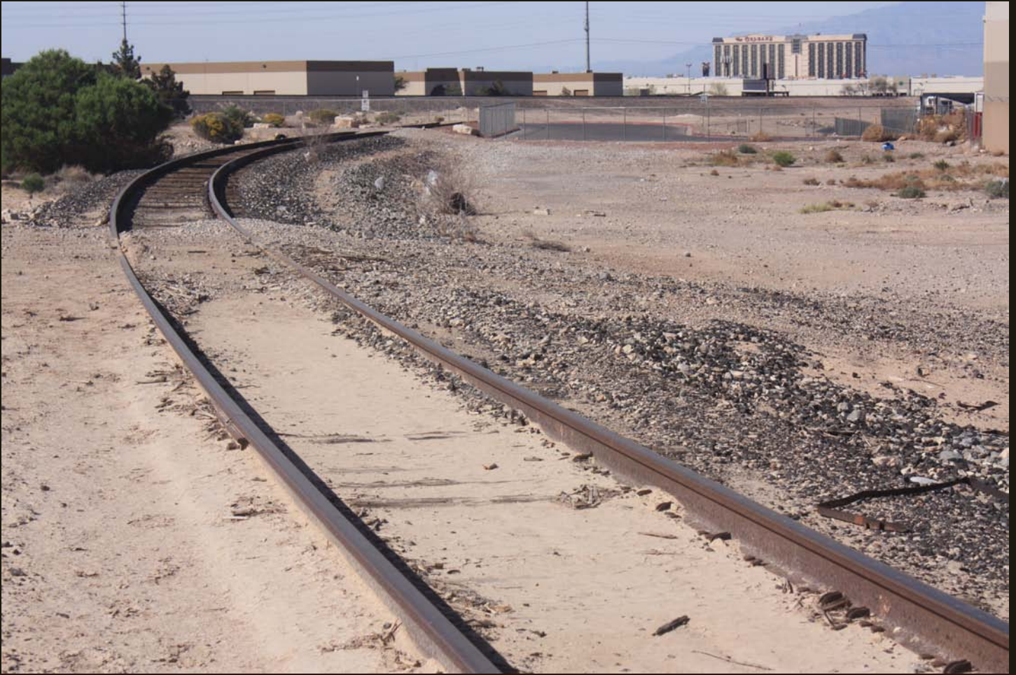
Northwestward view of the north branch of the wye for the LA&SL Boulder City Branch (1931). The track is cut just to the left of the chain-link fence and the SPLA&SL/LA&SL/UP mainline is on a higher grade in the distance.
