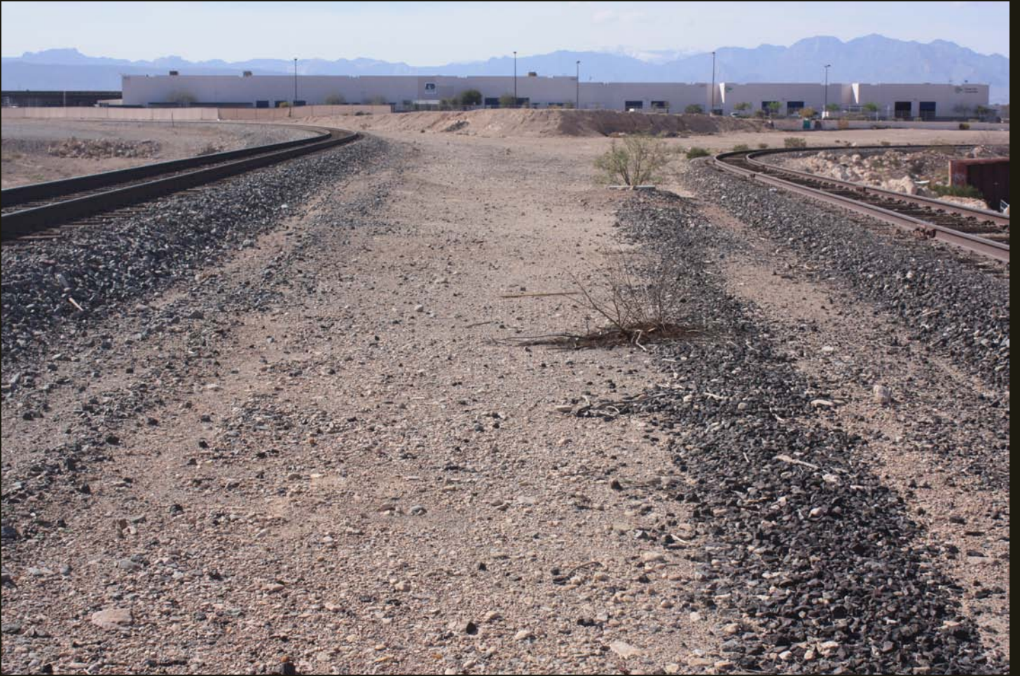
Westward view of the two branches of the wye for the LA&SL Boulder City Branch (1931).
