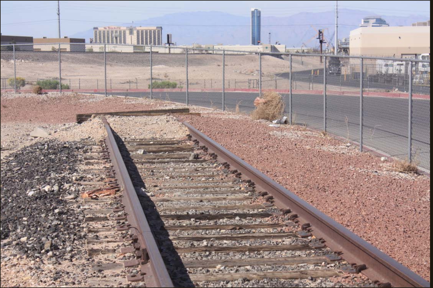
Closer view of the cut end of the north branch of the wye for the LA&SL Boulder City Branch (1931).
