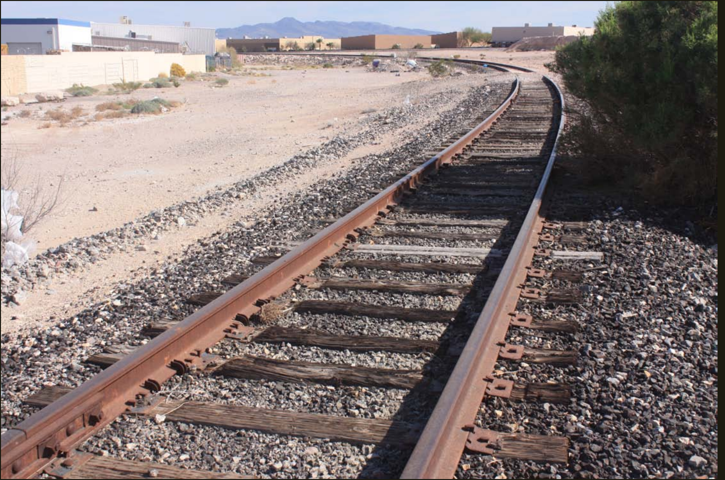
Southeastward view of the north branch of the wye for the LA&SL Boulder City Branch (1931).
