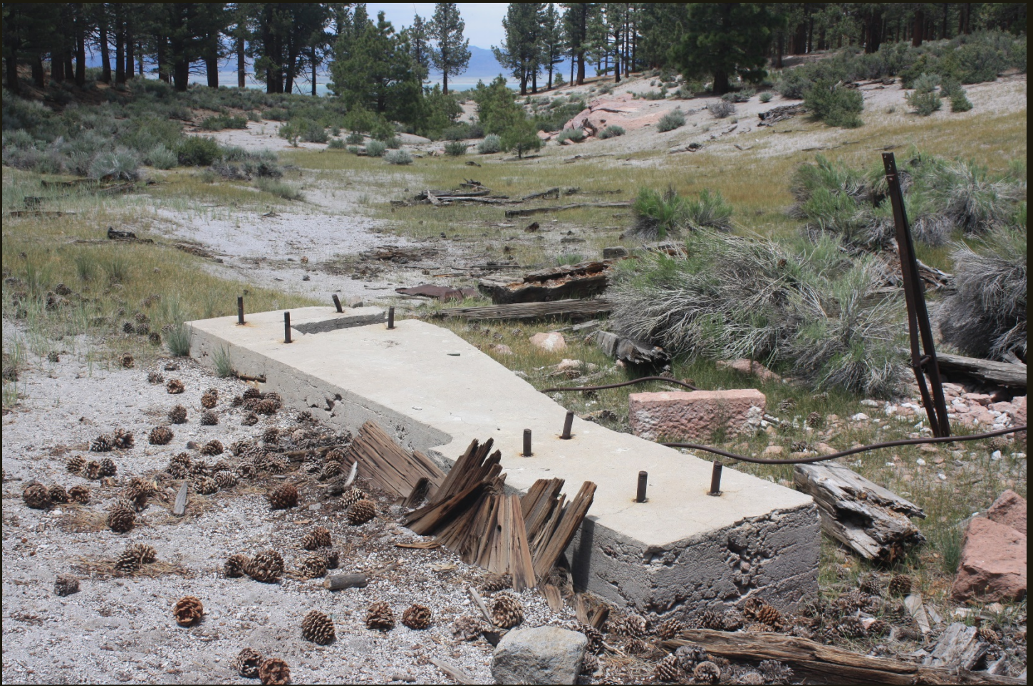
Closer view of foundations, discarded lumber, and the linear depression at Mono Mills.
