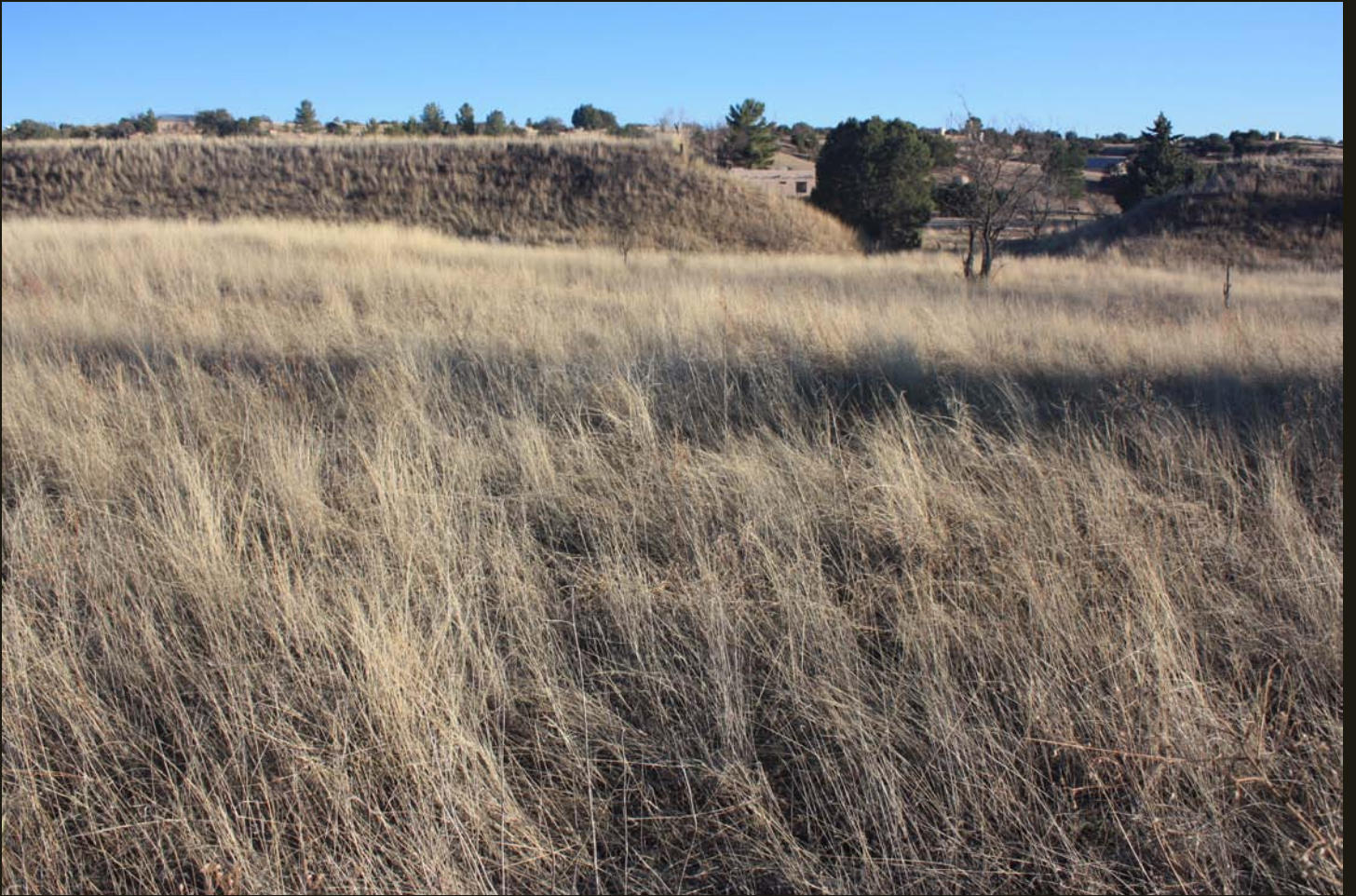
Southeastward view of the NM&A/EP&SW/SP grade, 1 mile west of Sonoita. Note the high fill grade and former overpass.
