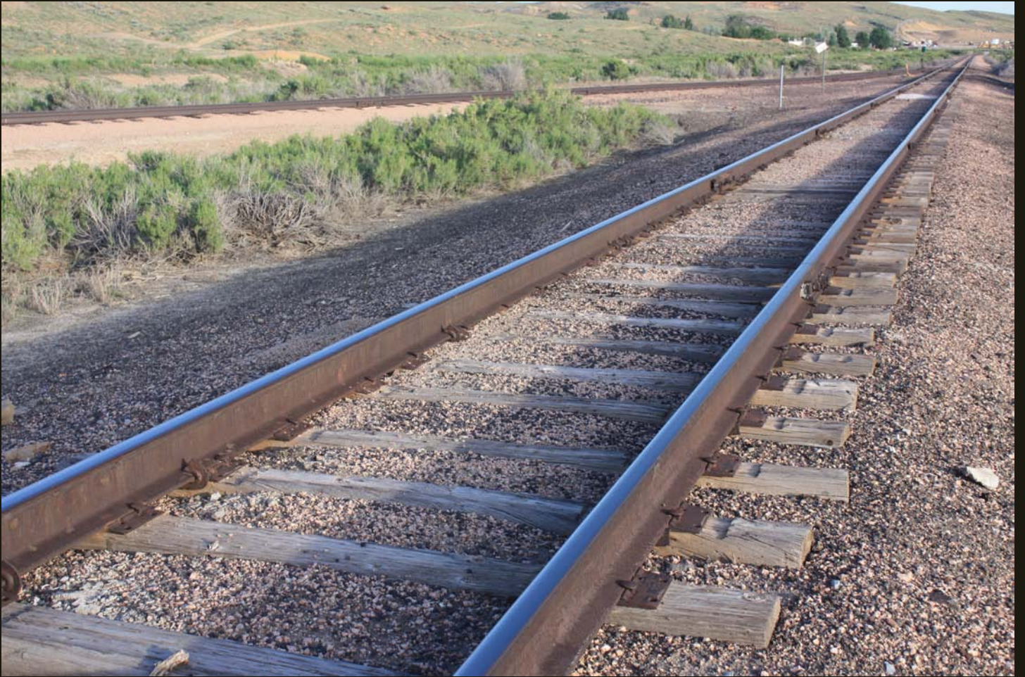
Southward view of the Winton Branch (right) and the Reliance Spur.
