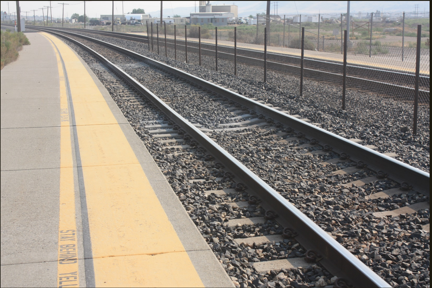
Eastward view of the CP (1869) on the left (north) and the WP (1909) on the right (south) at the Elko depot (same location as previous). Although both lines are now UP and, at this location, both tracks are on new alignments built in the 1980's, outside of town the north and south tracks connect to the CP (1869) and WP (1909) alignments, respectively. I'm not sure why the CP (1869) has concrete ties and the WP (1909) has wooden ties.
