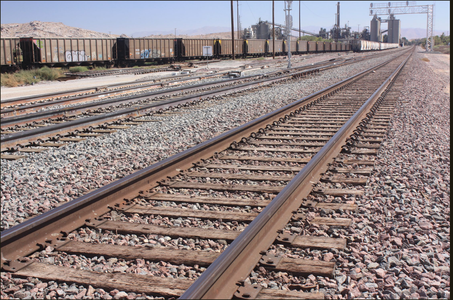
Southeastward view at the same location as previous. The double track in the foreground is the CS/AT&SF/BNSF mainline with sidings to the left. The ore cars on the left are on the big loop track, and additional cars are stored on one of the sidings in the distance with the plant just beyond.
