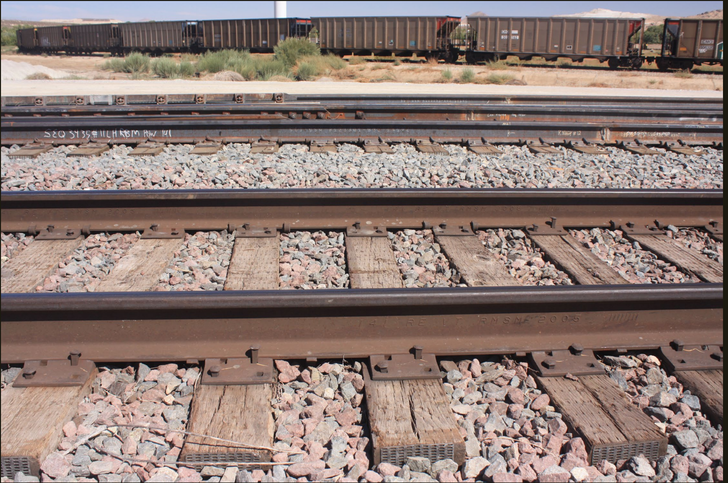
Northeastward view 2,000 feet northwest of the previous location. The double track in the foreground is the CS/AT&SF/BNSF mainline, and multiple sidings are visible just beyond. The ore cars are on the northwest end of a big loop track.
