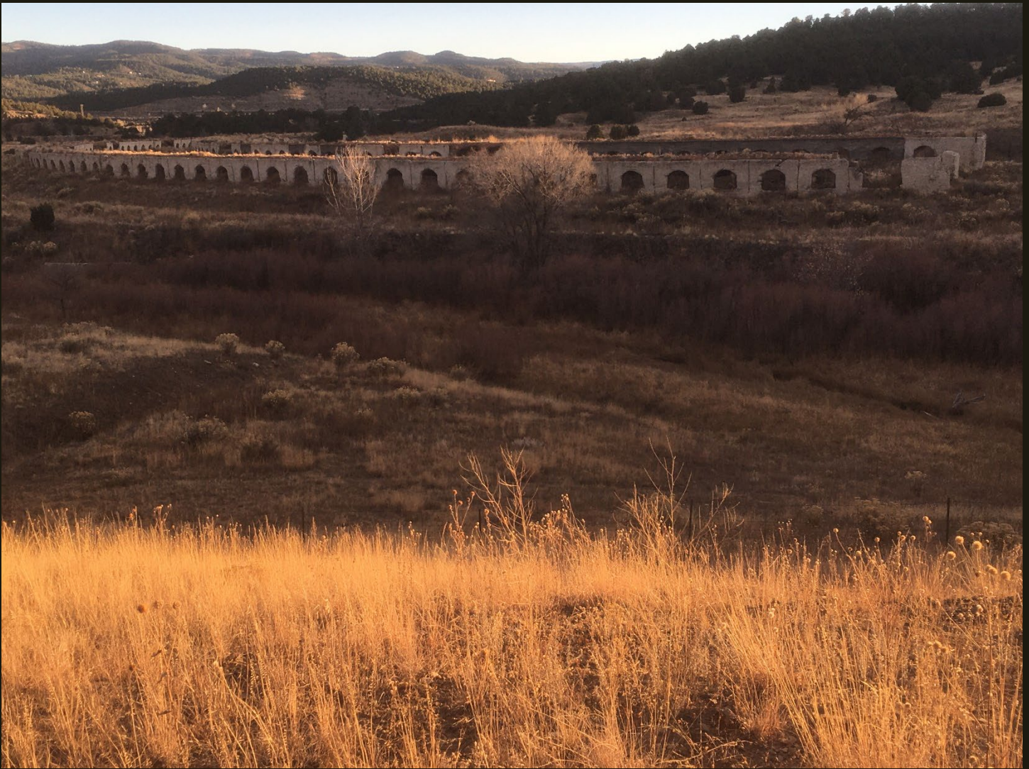
Southward view of the other side of the Cokedale ovens. The 2 bare trees in the center of the photo are growing along the small drainage of Reilly Canyon and the berm just on the other side of the trees and the stream is the fill grade of the Cokedale spur. The spur may have extended 7 miles to the northwest (right) up Reilly Canyon to Boncarbo and the connection to the C&W (1903) is one mile to the south (left) down Reilly Canyon to the confluence of this stream with the Purgatoire River. The ovens were served by one or more sidings off of the main spur.
