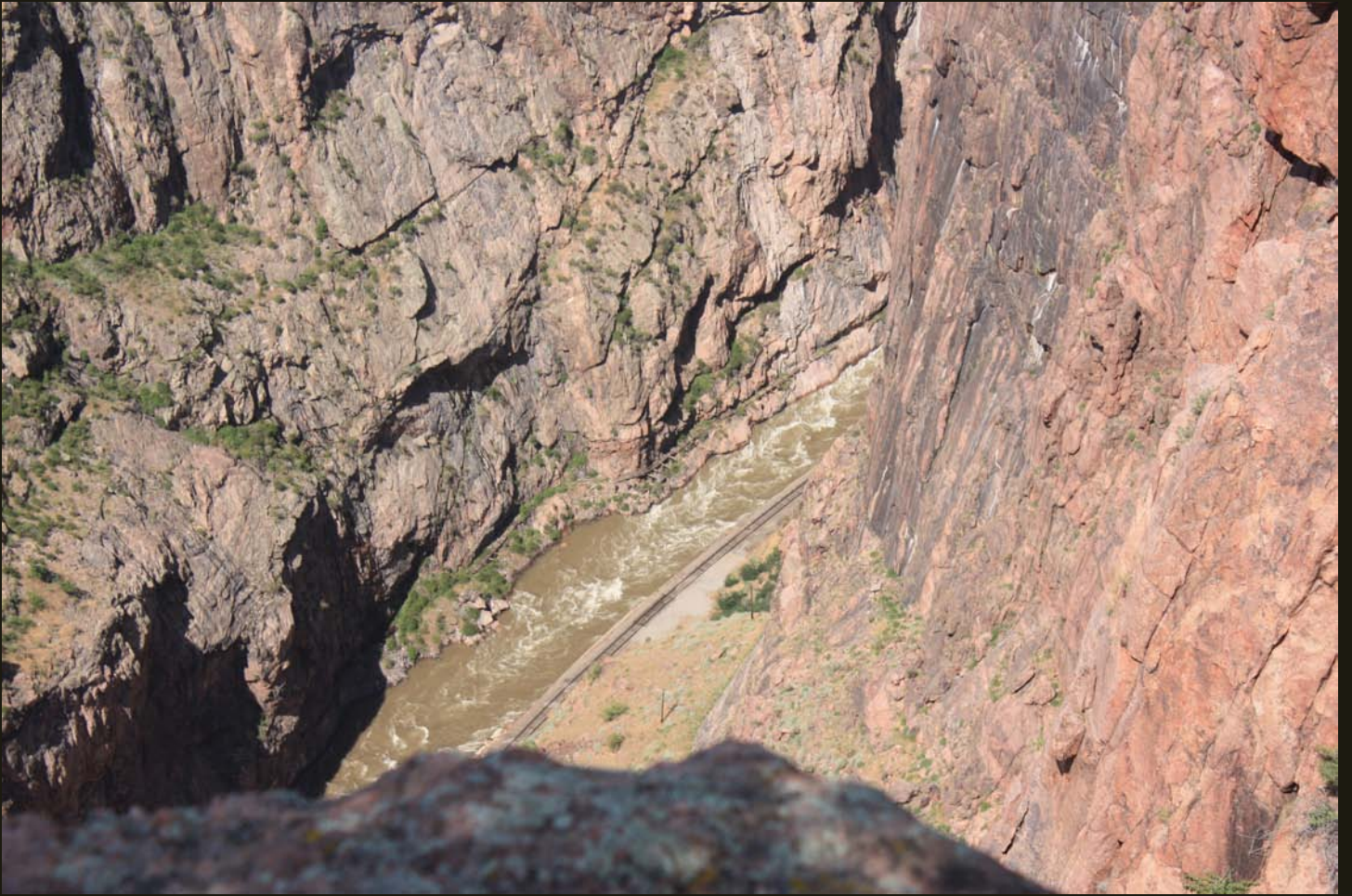
Closer view of the D&RG line through Royal Gorge, first built as a narrow gauge line in 1879 and converted to dual gauge in 1888.
