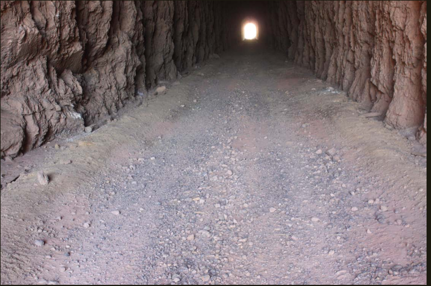
Eastward view of the EP&SW (1904) grade in the Crook Tunnel.
