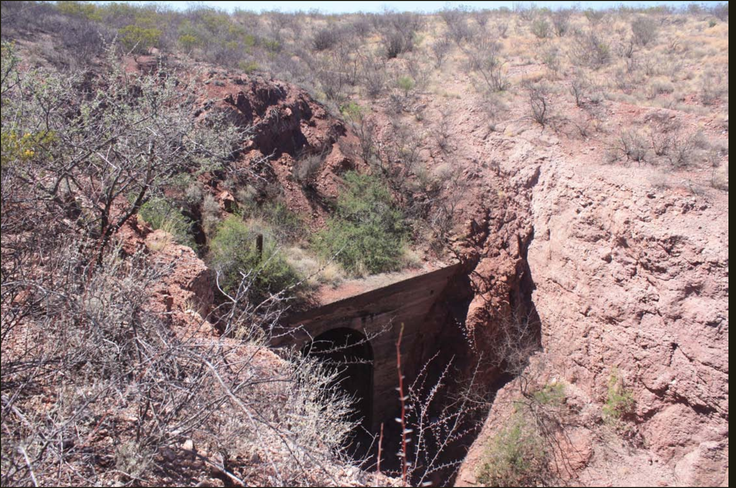
East entrance to the Crook Tunnel.
