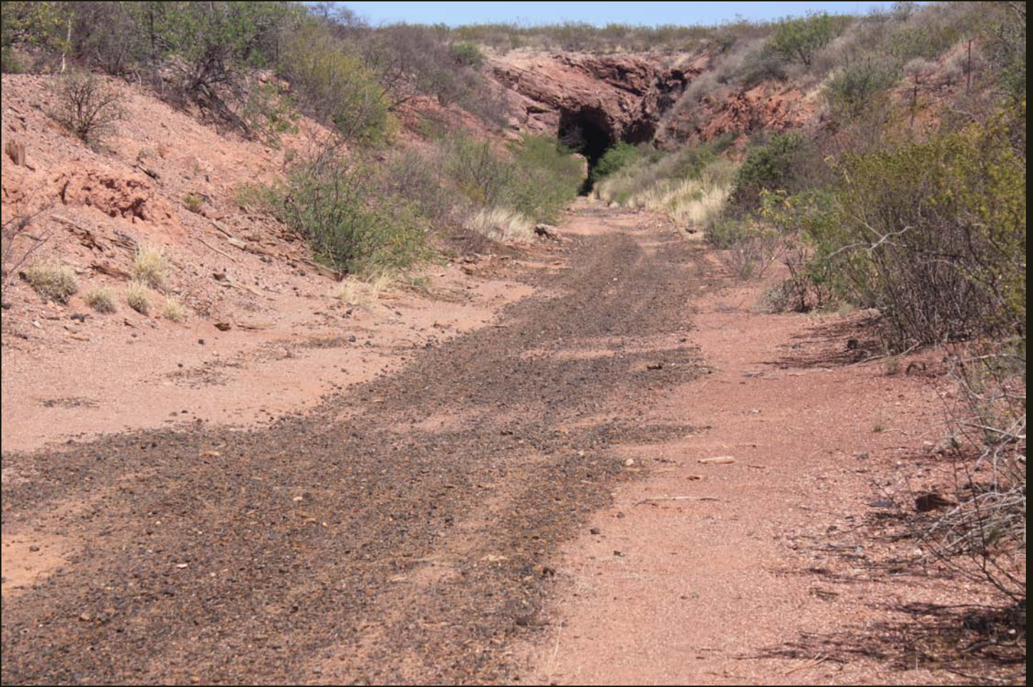
Eastward view of the west entrance of the Crook Tunnel on the EP&SW (1904). On-line sources indicate the tunnel was built in 1902, but the entire re-alignment south of Bisbee was completed in 1904. Note that the west entrance is unfinished rock, whereas the east entrance is concrete.
