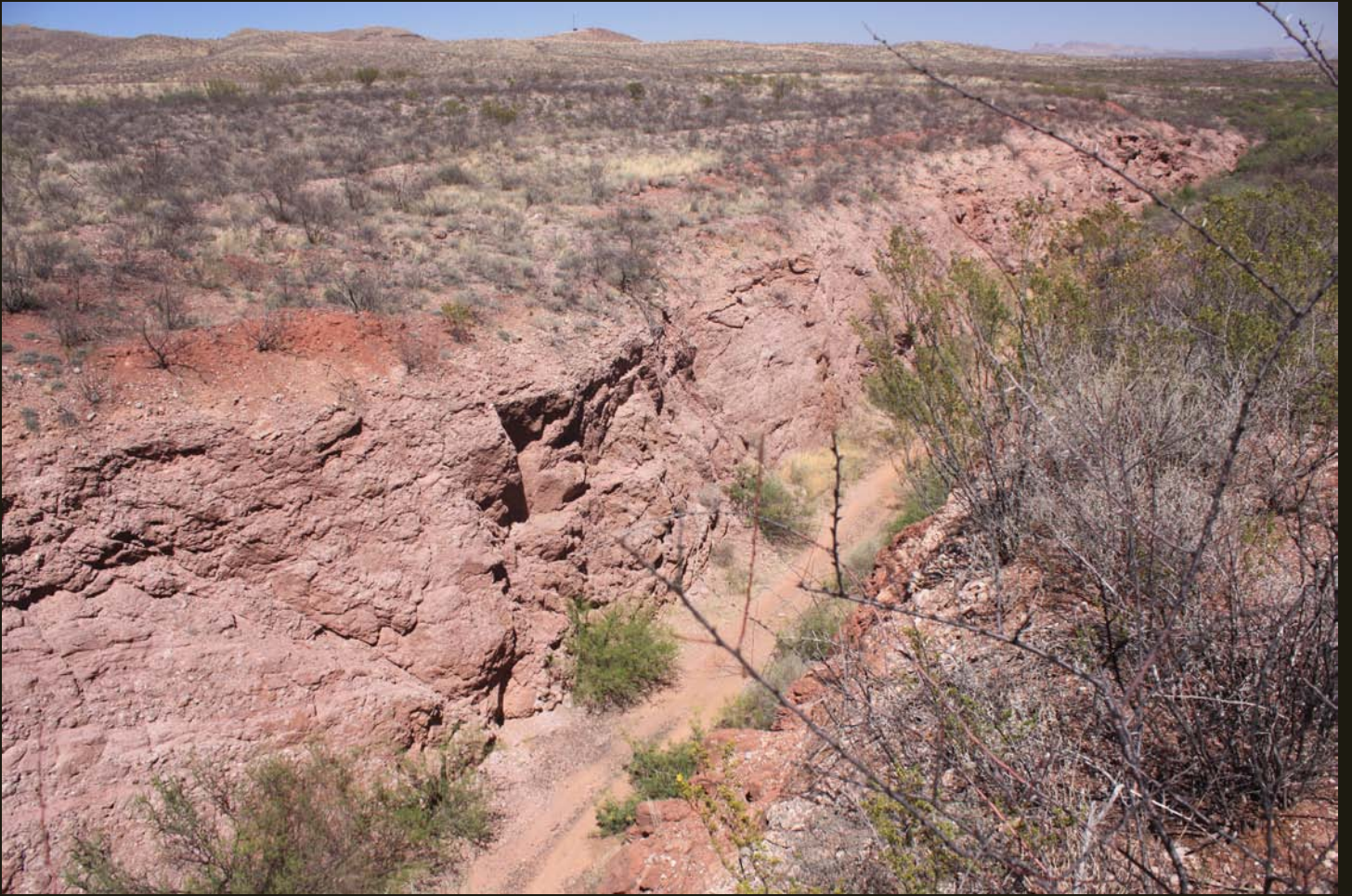
Northeastward view of the cut grade of the EP&SW (1904) just east of the Crook Tunnel.
