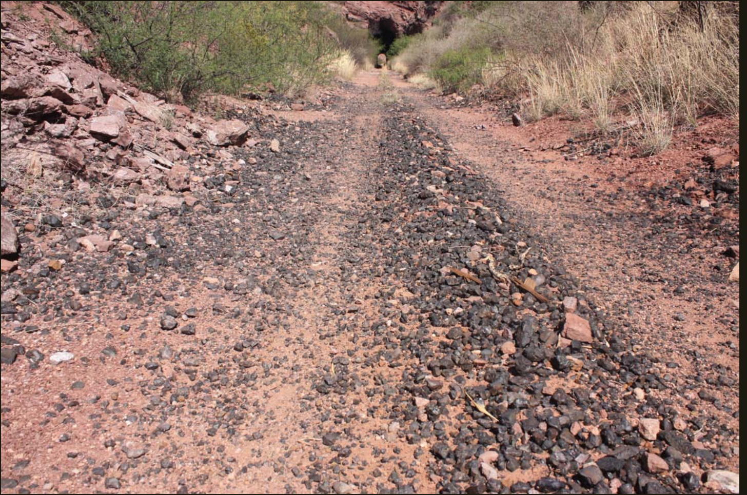
Eastward view of the west entrance of the Crook Tunnel, showing detail of the slag ballast, which is essentially man-made obsidian (volcanic glass).
