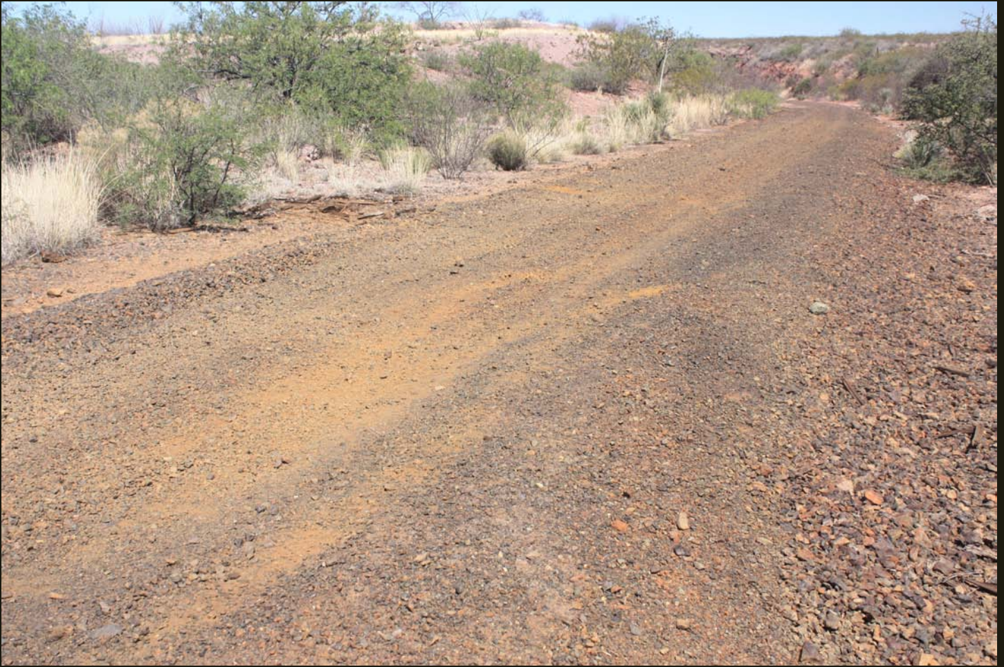
Eastward view of the approach to the west entrance of the Crook Tunnel on the EP&SW (1904), 2 miles east of previous location. This section of the line was abandoned in July 2006.
