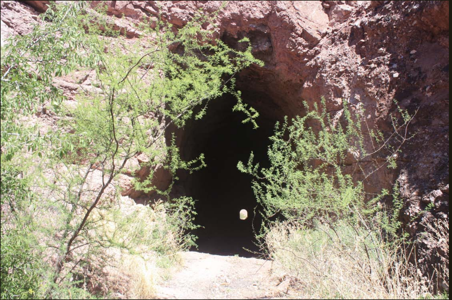
Eastward view of the west entrance of the Crook Tunnel on the EP&SW (1904), showing the unfinished rock entrance and the smoother outline of the concrete east entrance at the far end. The small trees are mesquite. The piece of a tie pictured below is all I could find of the EP&SW other than the grade and tunnel.
