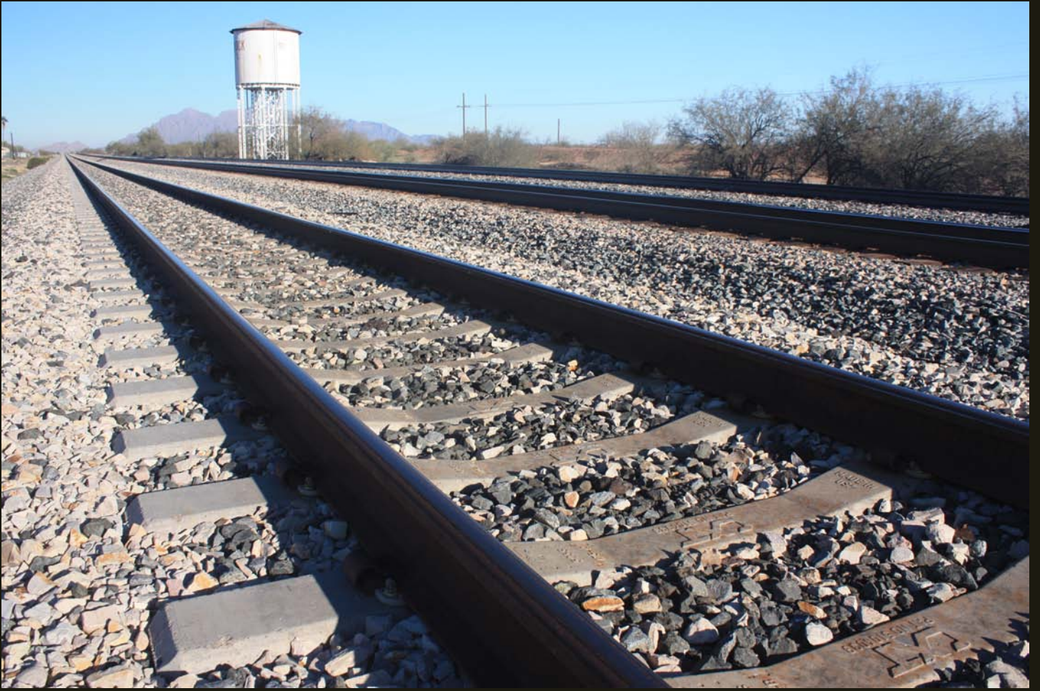
Another view of the water tower at Red Rock. Note the double track, one with upgraded concrete ties.
