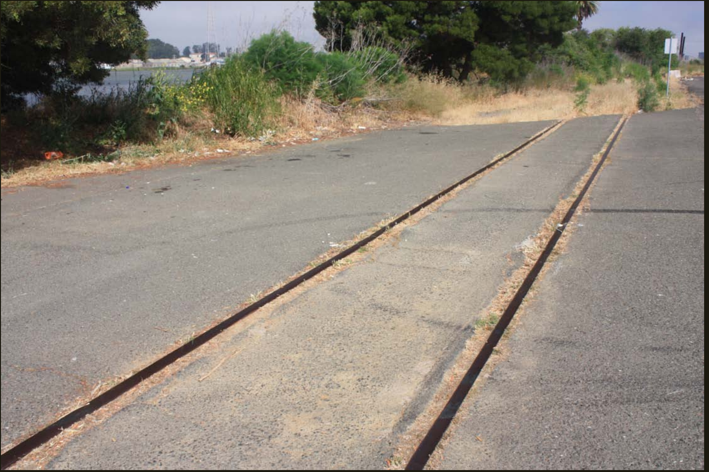
Northward view, 800 feet south of the previous location, of the single track that continues south of the yard.
