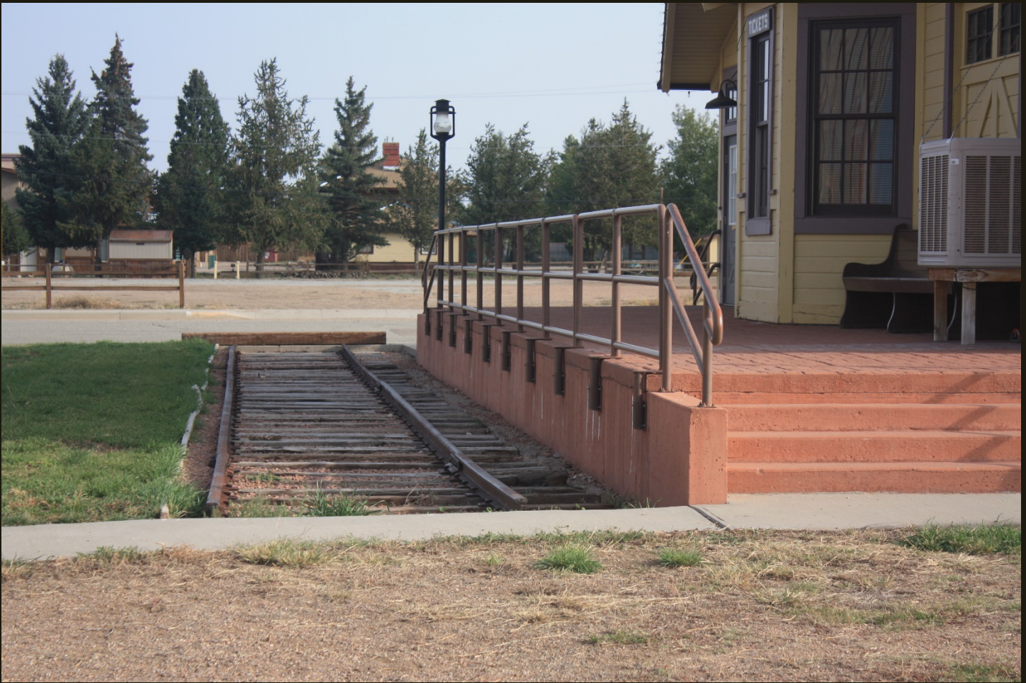
Some track along a loading dock on the other side of the warehouse. This track is on the same north-south alignment as the track next to the depot, which is visible through the trees in the center distance.
