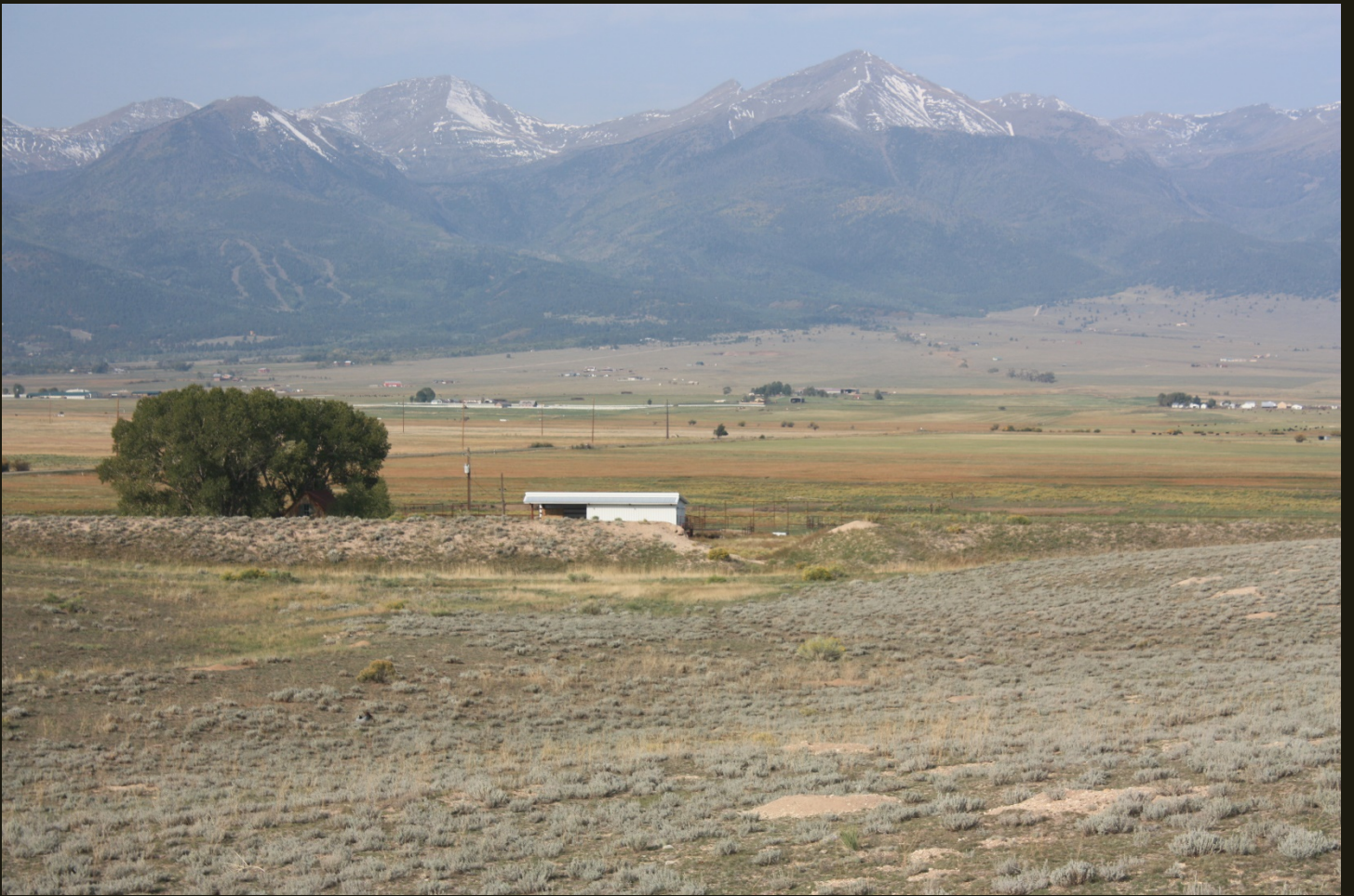
Westward view of the breached fill grade (just in front of the white building and trees) of the D&RG Westcliffe Branch (1900) 6 miles southeast of the previous location and 1 mile northwest of Westcliffe. The backdrop is the 13,000-foot Sangre de Cristo Range.
