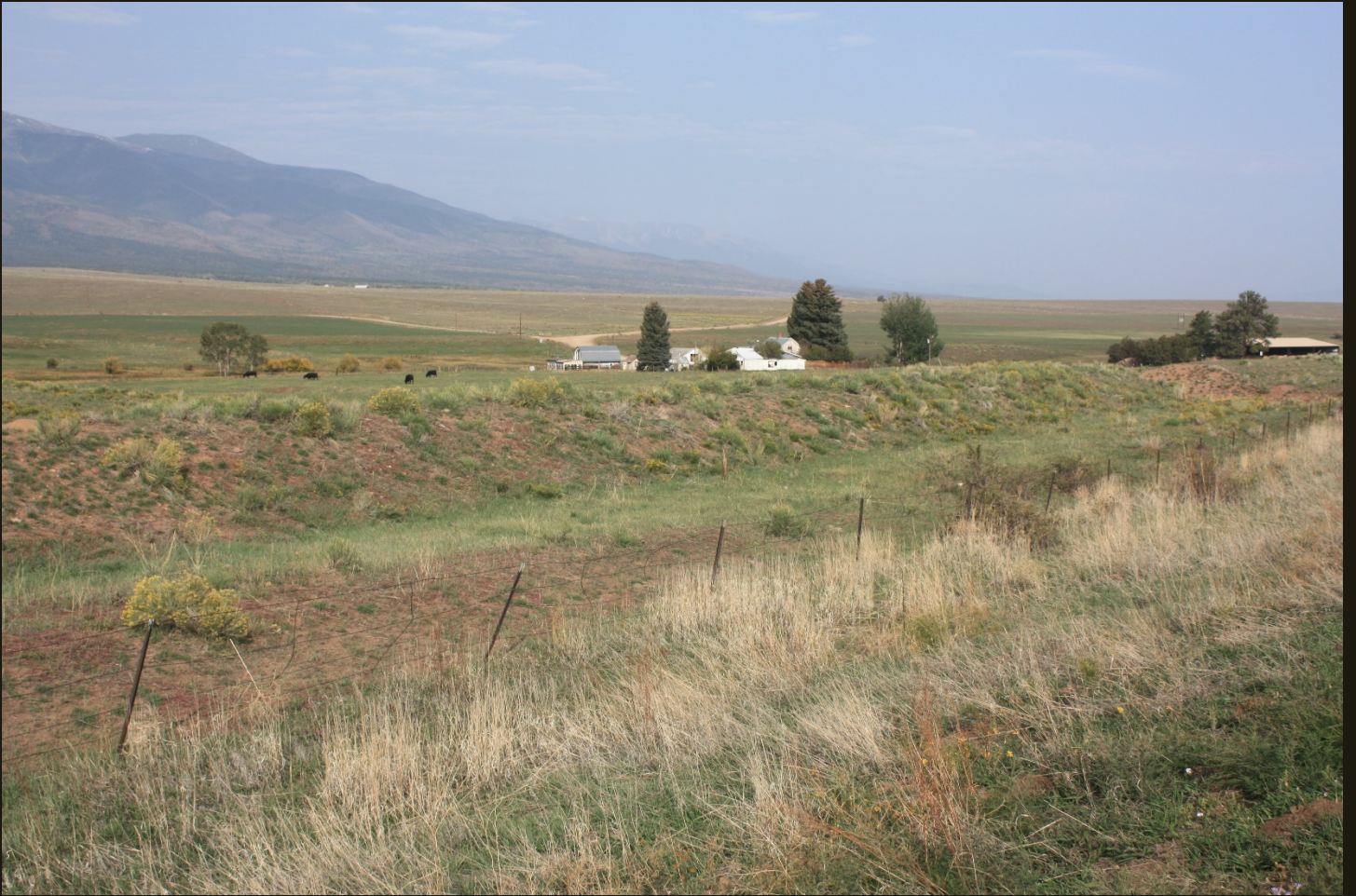
Northwestward view of the fill grade of the D&RG Westcliffe Branch (1900) one mile south of the previous location.
