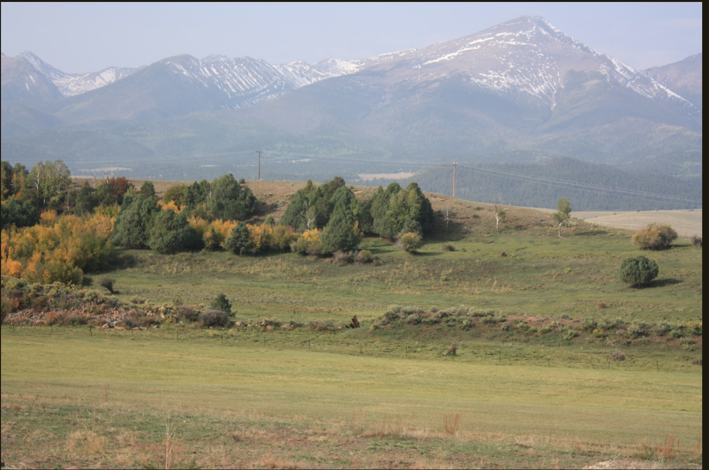
Closer view of the pilings and fill grade of the D&RG Westcliffe Branch (1900).
