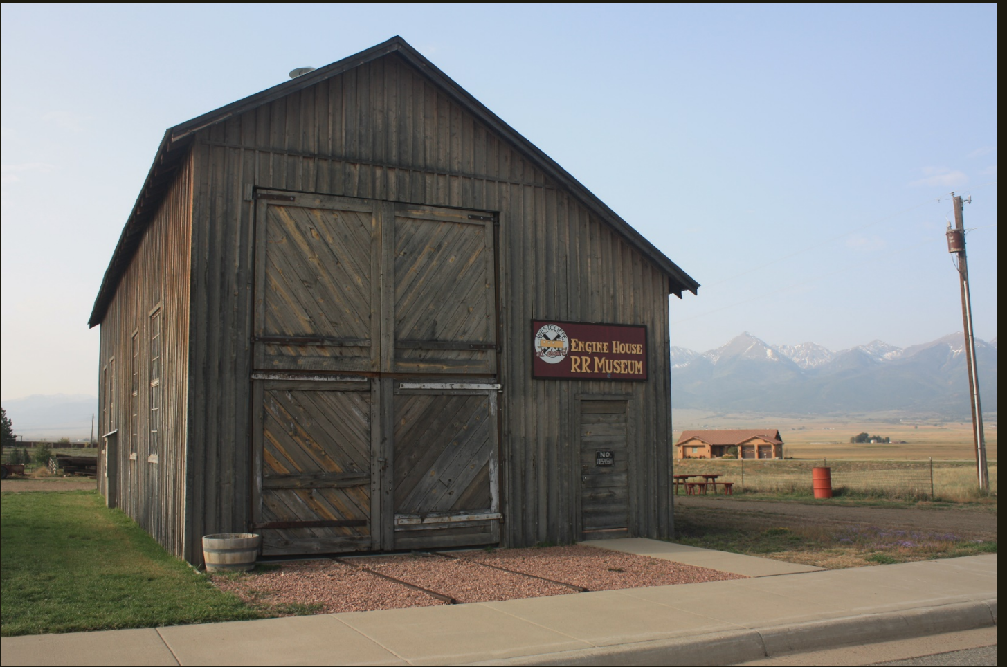
Closer view of the 1901 engine house.
