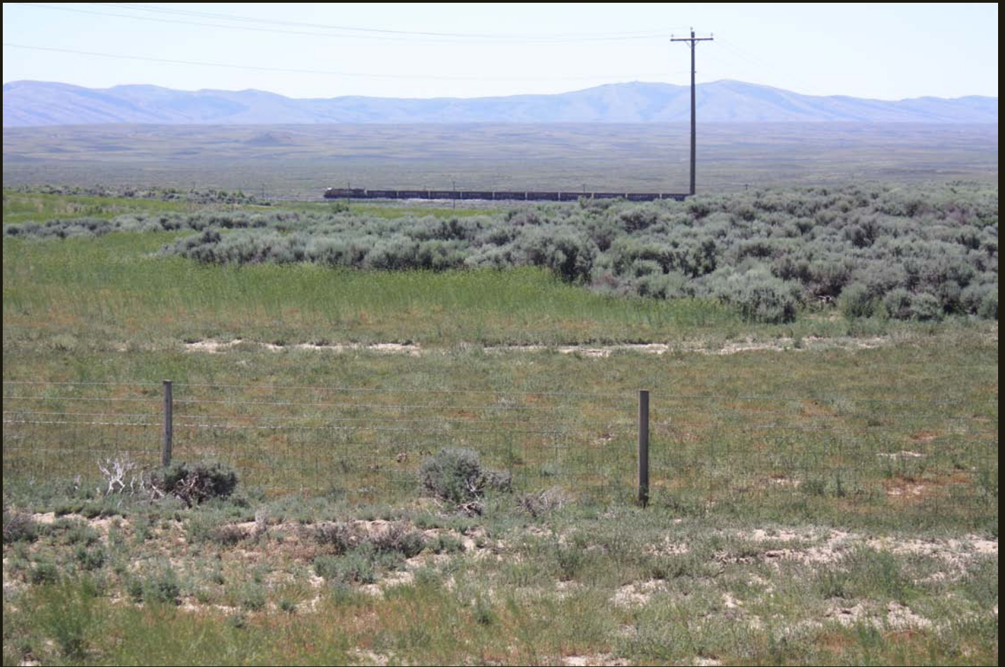
The UP mainline crosses the Great Divide Basin and therefore crosses the divide twice. This southward view of the UP mainline shows the gentle topography at the summit of the eastern of the two crossings at Hadsell, Wyoming, about 8 miles west of Rawlins.
