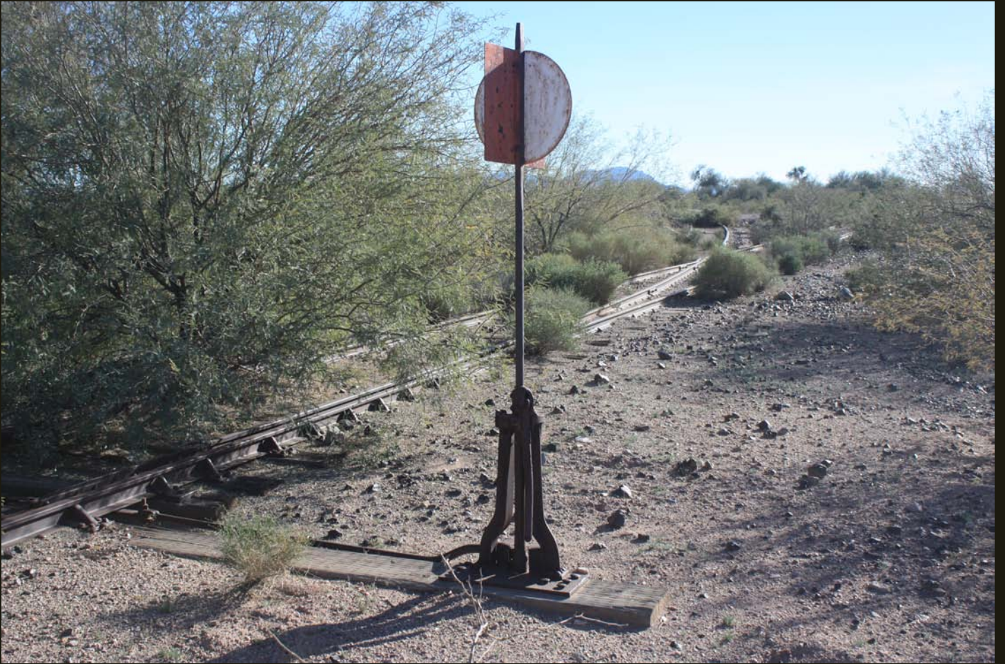
Track switch at Stout Spur.
