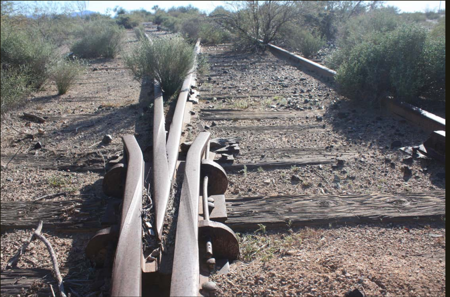
Track switch at Stout Spur.
