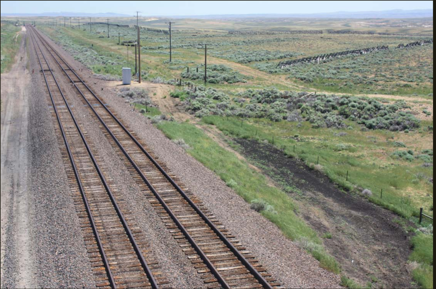
Another view of the UP mainline near Creston Junction. Note the snow drift fences.
