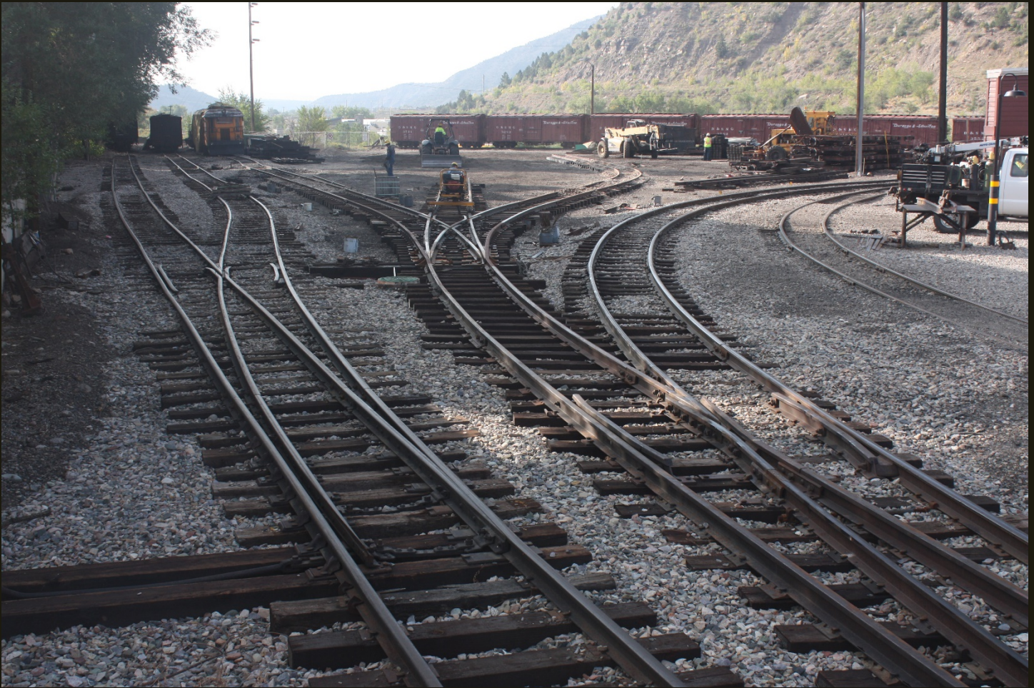
Southward view of the south end of the D&SNGRR railyard, 300 feet south of the previous location. The D&RG San Juan Extension (1881n) mainline is on the far left and ends just beyond the stored car. South from there, the grade disappears. The Animas River is 300 feet beyond the line of stored box cars. The RGS (1891n) entered the area of the current railyard to the left (west) of this location and turned southeastward to join the D&RG San Juan Extension (1881n) about 400 feet south of the current end of track, according to historical topo maps. The curved track on the far right is a turnaround loop; as far as I can tell, the turnaround loop and all tracks in the railyard except the mainline were built by the D&SNGRR and are not historic.
