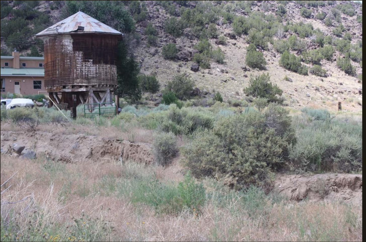
Closer view of the Embudo water tower. The grade is not discernable.
