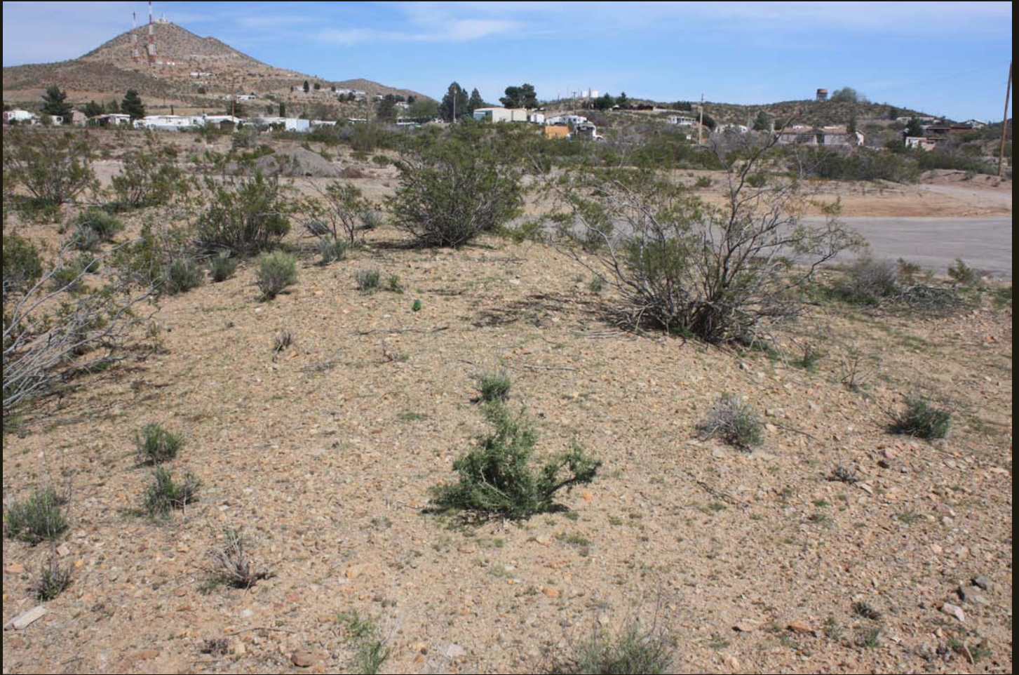
Northeastward view of the B&S (1907), same location as previous. The B&S fill grade is the mound of dirt in the foreground and breached by a paved road. The line extended through the mobile home park in the left distance and ended just beyond the park. A turning wye, water tower, and depot were once present in this view. Much to the chagrin of Searchlight residents in 1906-1907, the CE/AT&SF did not do the extra work to extend the line up the hill another half mile to the town of Searchlight, which is just beyond the old water tower on the hill in the upper right of the photo.
