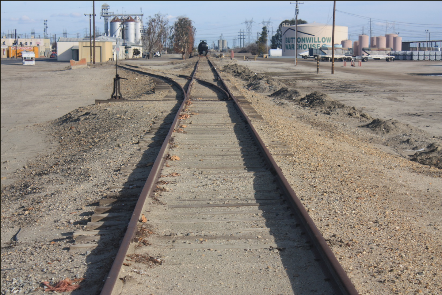
Eastward view of the MS (1893) at Buttonwillow. A tank car is stored on the main line and an agricultural siding is present on the left (north).
