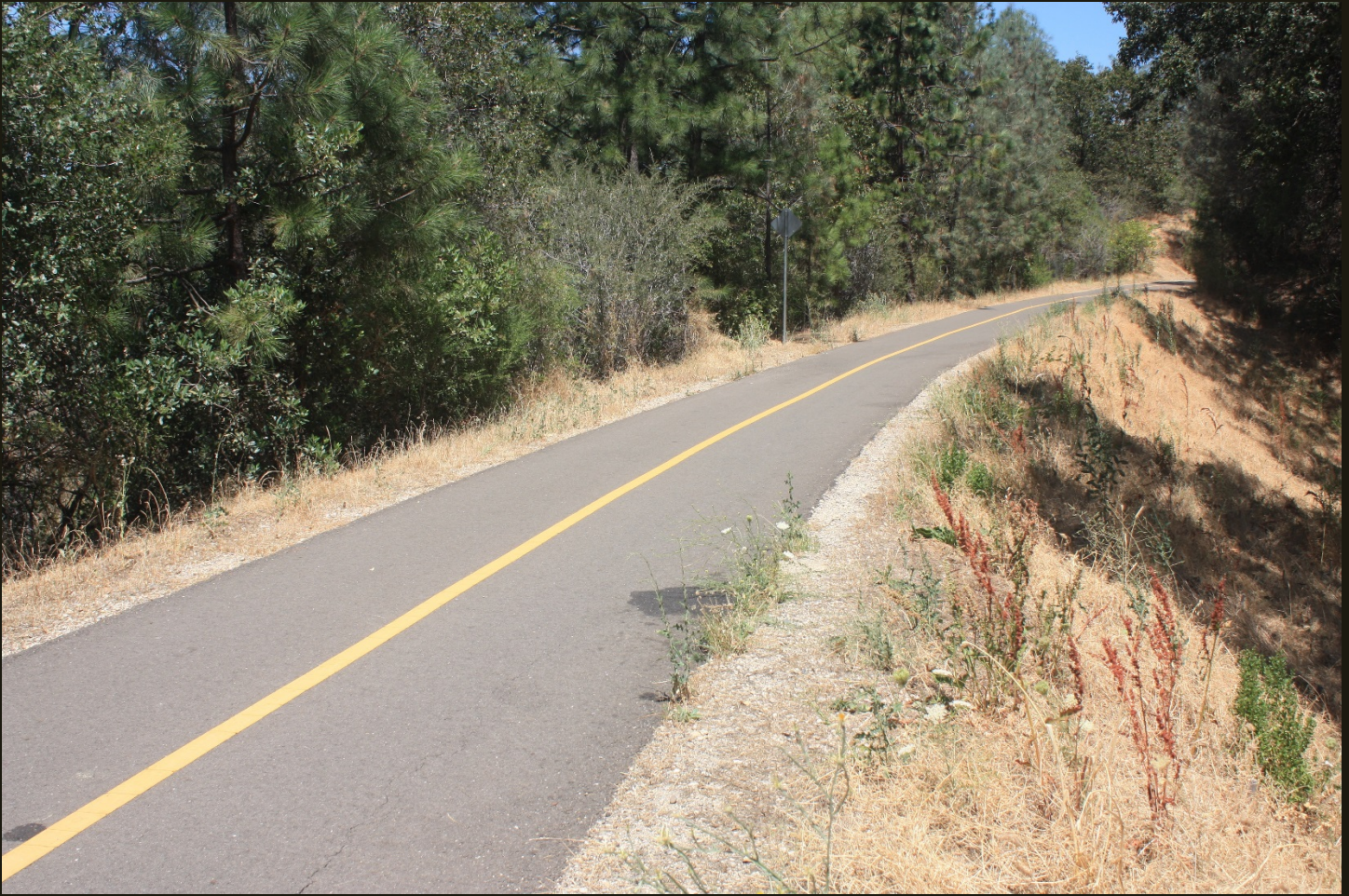
Northeastward view of a fill grade on the S&P (1888) one mile north of the Weber Creek Trestle and one mile west of the S&P end-of-the-line in downtown Placerville.
