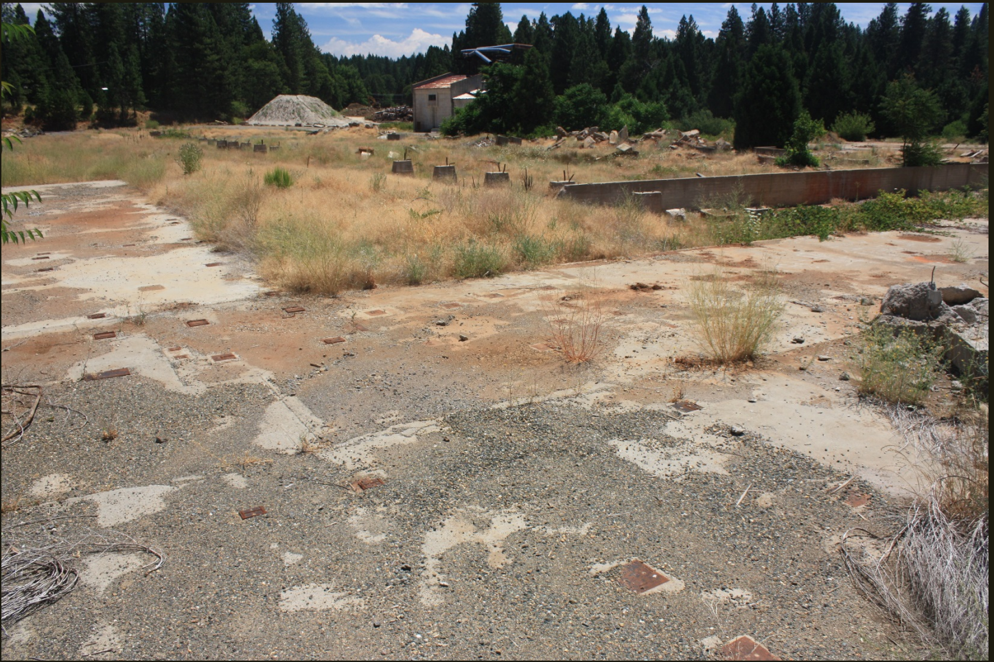
Southward view of foundations for the abandoned El Dorado Lumber Company/Michigan-California Lumber Company mill in Camino, 300 feet east of the previous location.
