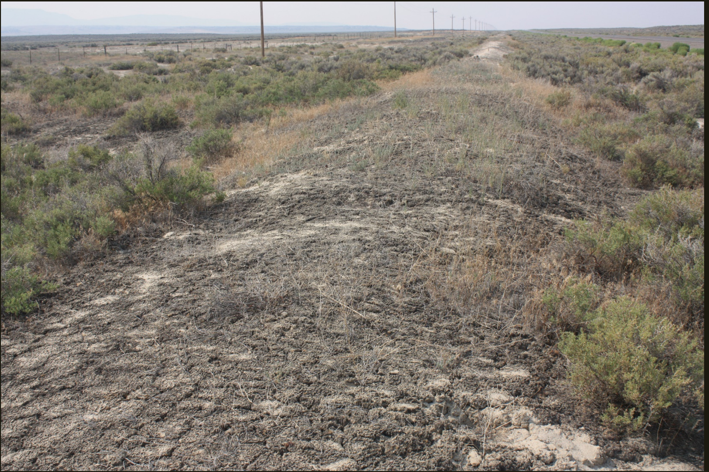
Southward view of the light fill grade of the E&P (1875n) at the same location as previous. Pine Creek is one mile west of this location.
