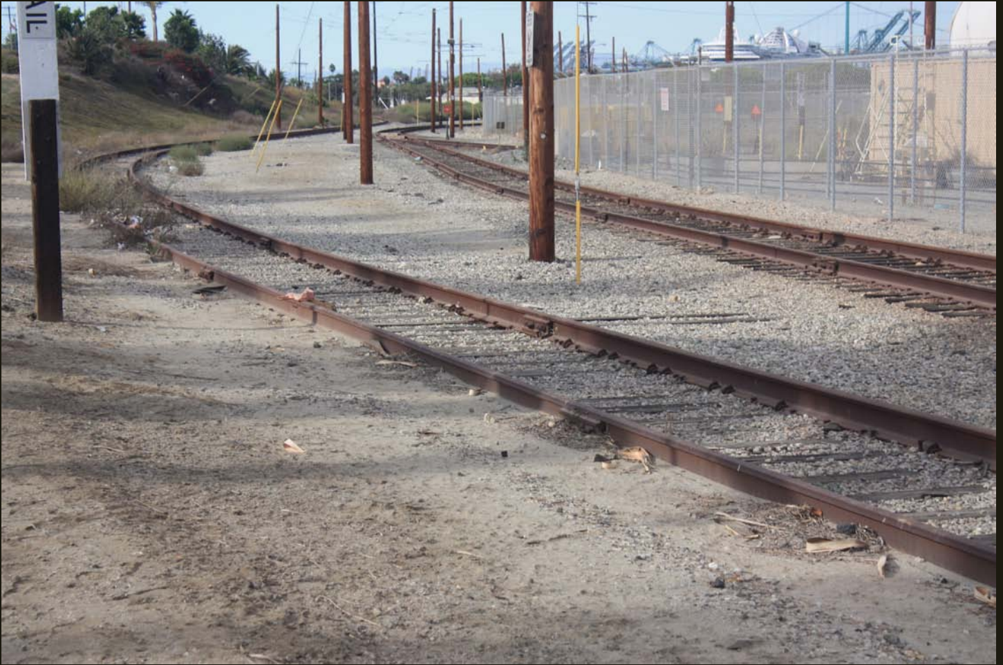
Northward view about 1,000 feet south of the previous location. All the track in this view is track, sidings, and spurs for the western of the two major wharfs built by the SP in 1911-1912. The split with the branch for the eastern wharf is just out of site in the distance.
