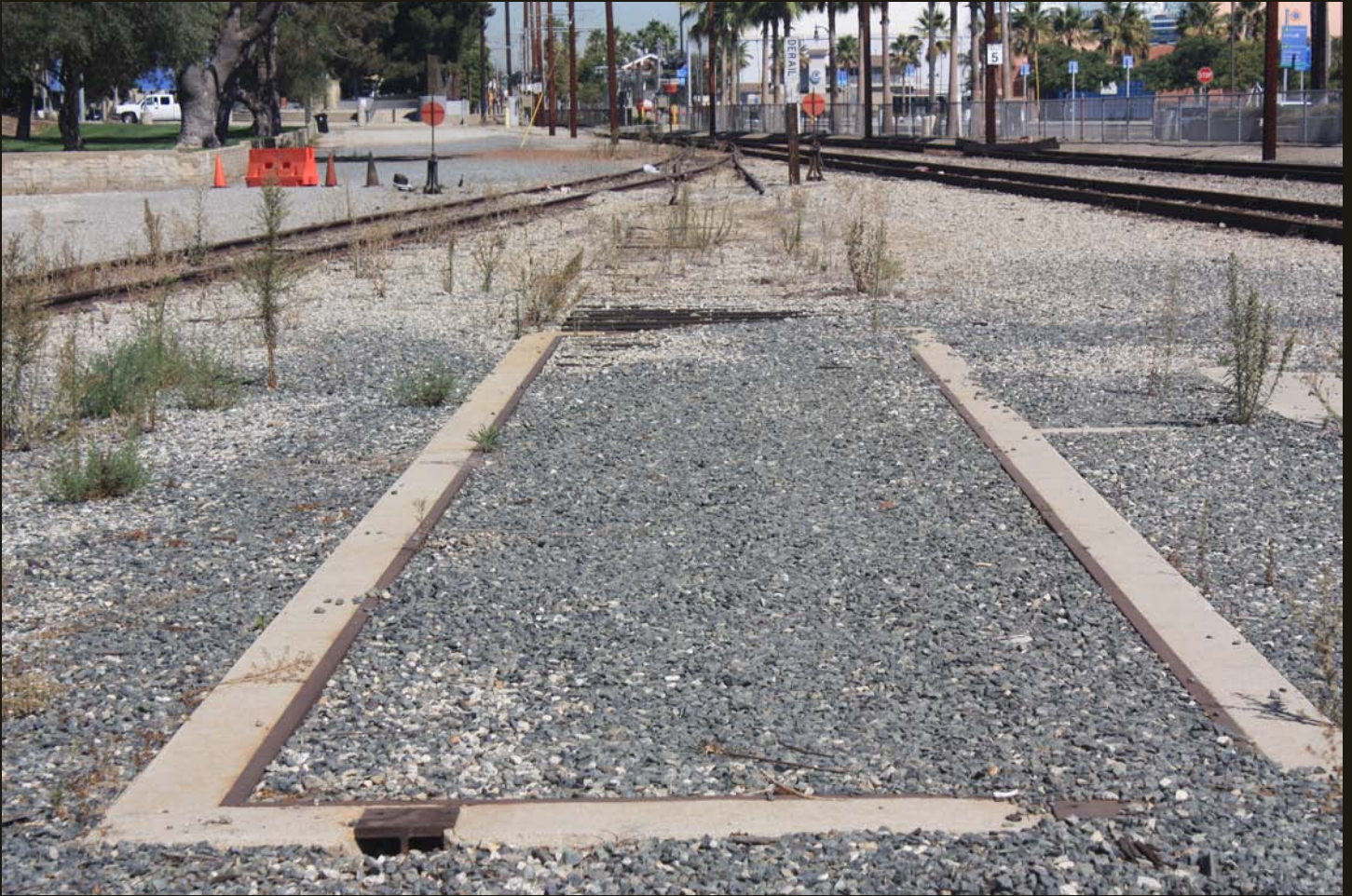
Northward view of the San Pedro yard, with some sort of abandoned facility in the foreground.
