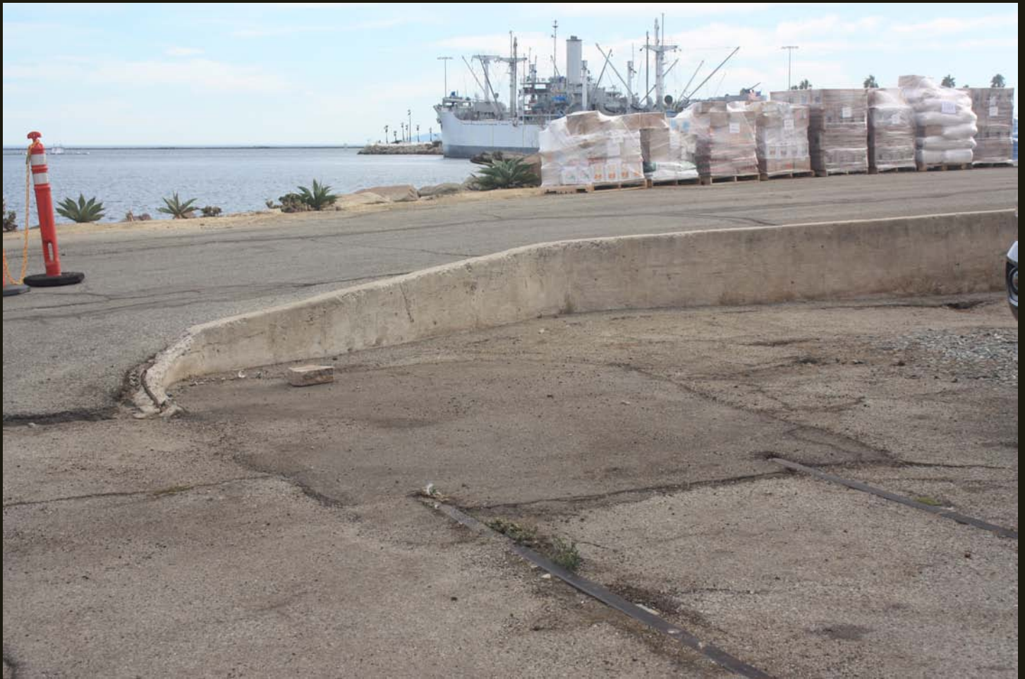
Southward view of the south end-of-track of the eastern of the two major wharfs built by the SP in 1911-1912. This is 4,000 feet south of the split with the western wharf branch line and a mile south of the San Pedro yard.
