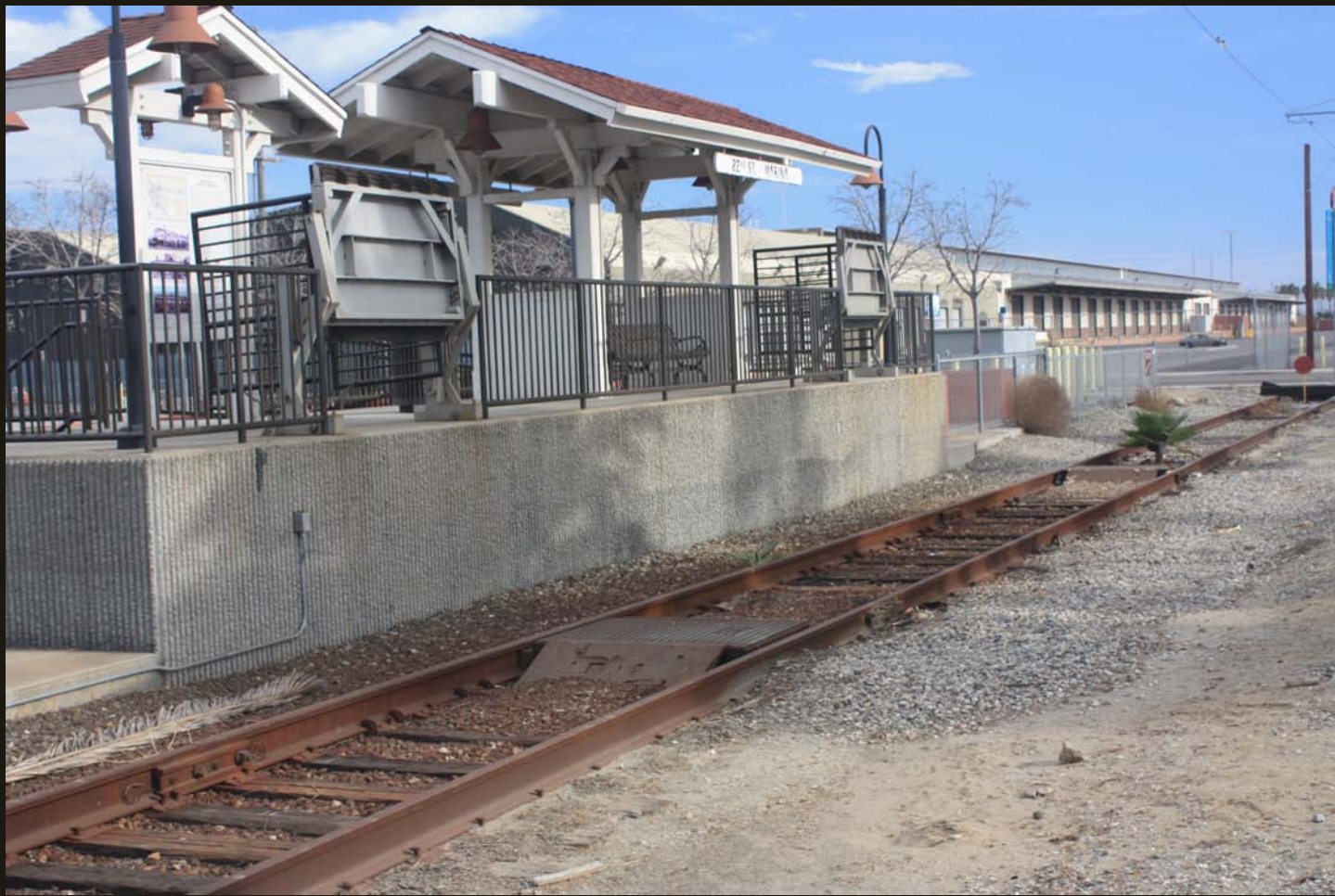
This is the end-of-track of the western of the two major wharfs built by the SP in 1911-1912, about a quarter mile south of the split with the eastern branch. The small depot in disrepair is the last stop on the closed Waterfront Red Car Line.
