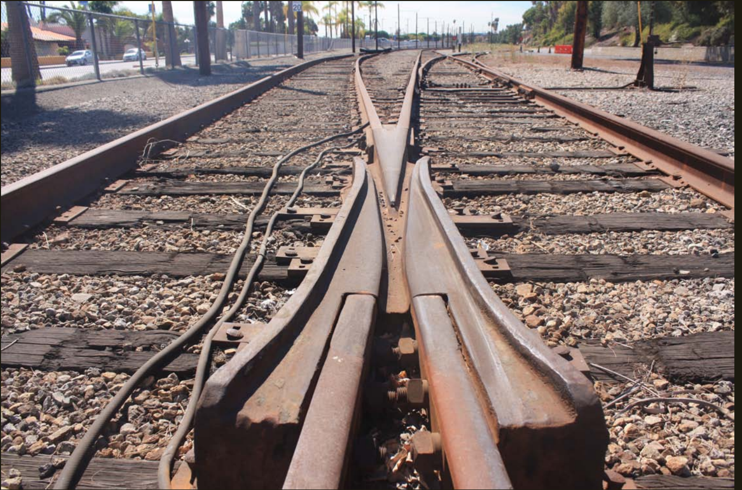
Southward view of the initial track split, same location as previous.
