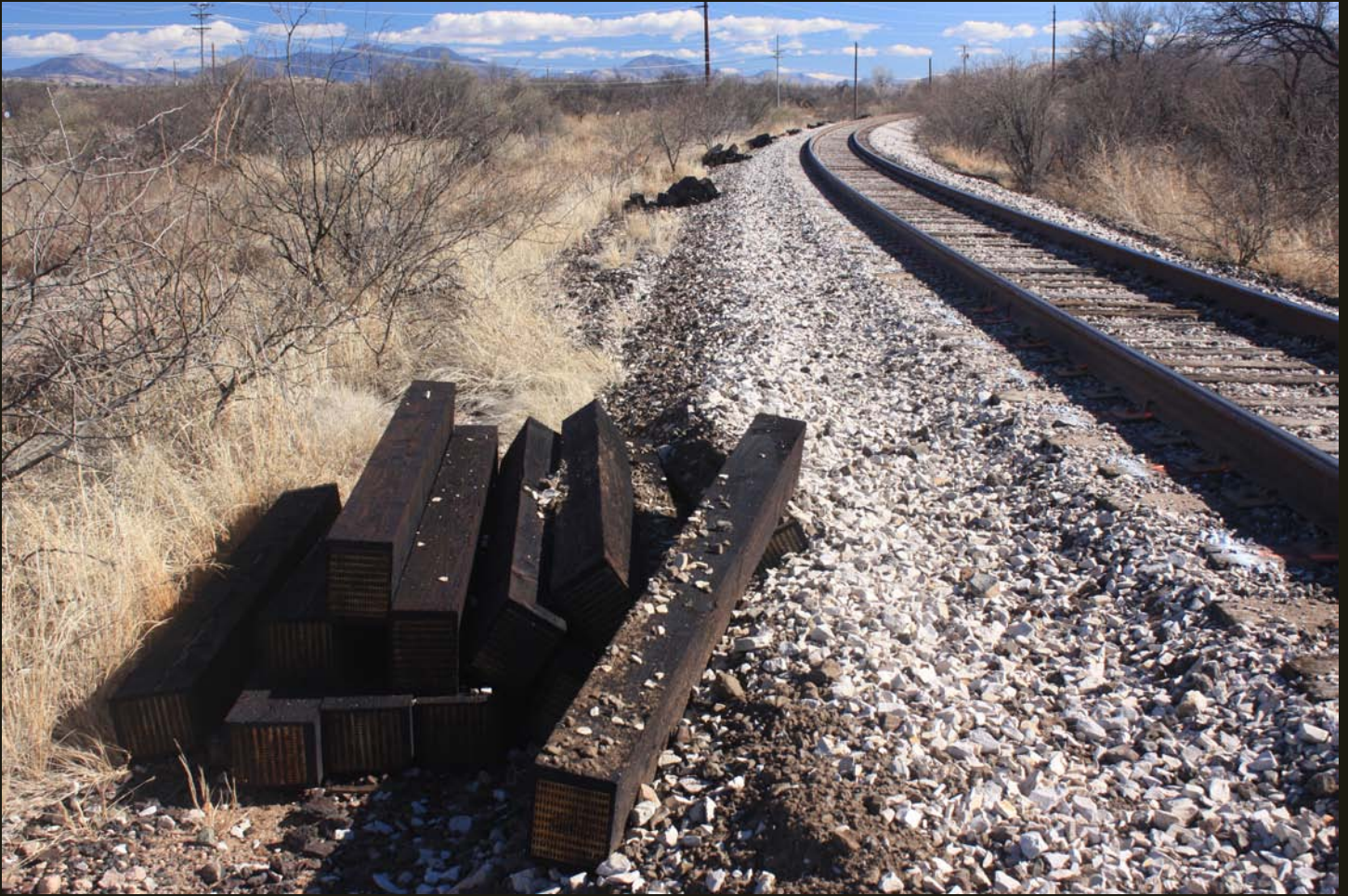
Southward view of the T&N (1910) at Calabasas, just south of the trestle over Sonoita Creek. The junction with the NM&A is probably in this view, but I could find no evidence for it on the ground, in aerial images, or in on-line maps.
