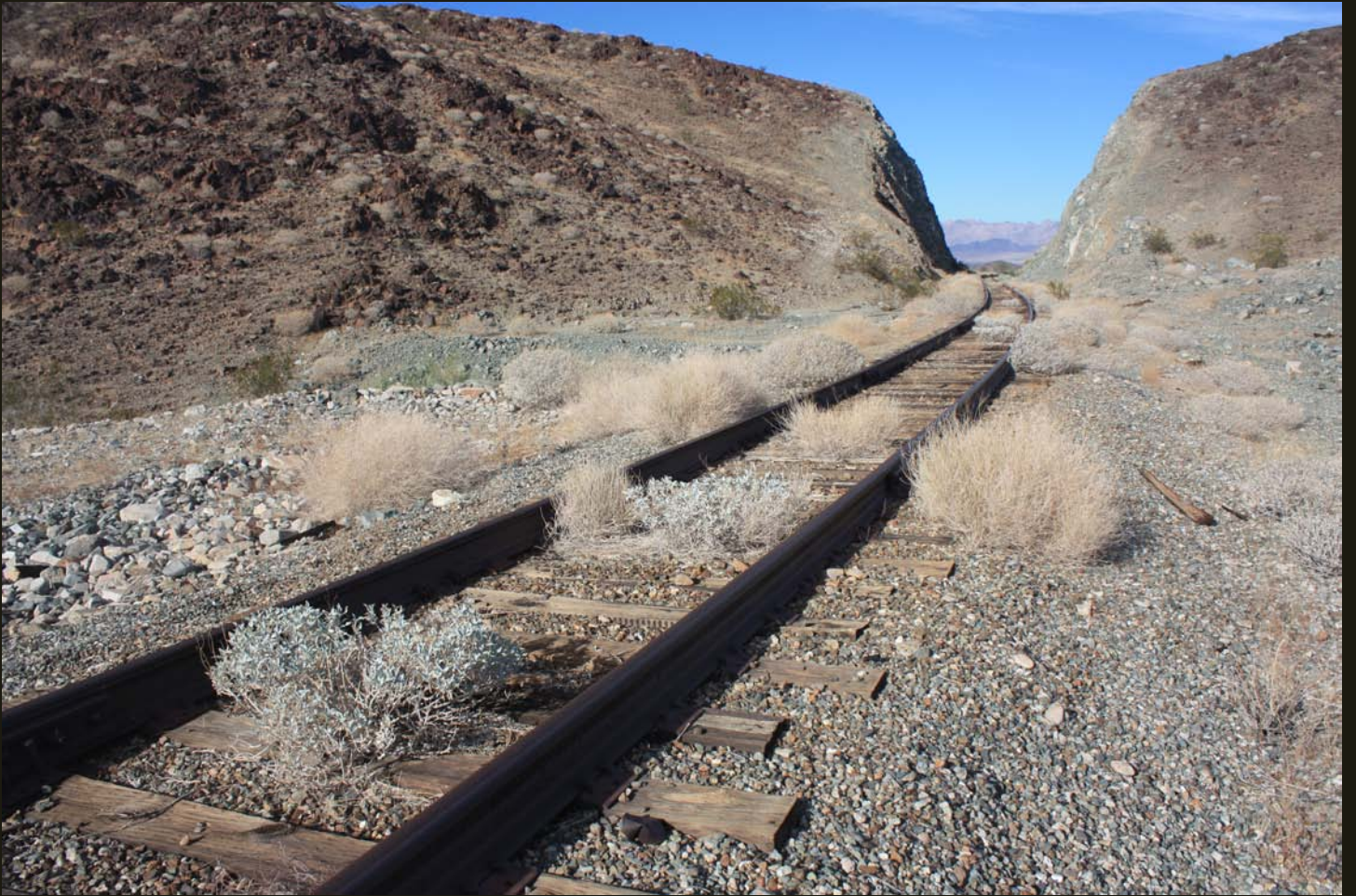
A cut through a small hill on the EMRR route.
