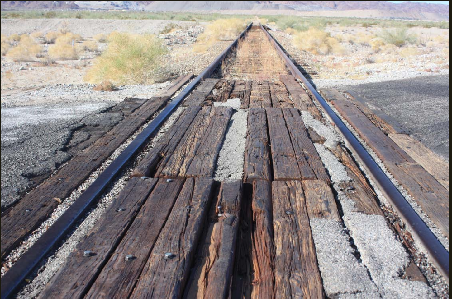
Rail ties were used for this road crossing of the EMRR.
