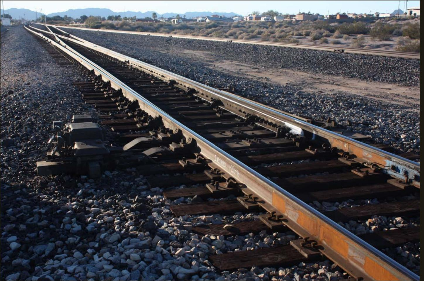
Westward view of the SP Sunset Route (1881) in the foreground, connecting in the distance with the bolted track of the SP (1926) cutoff to Phoenix.
