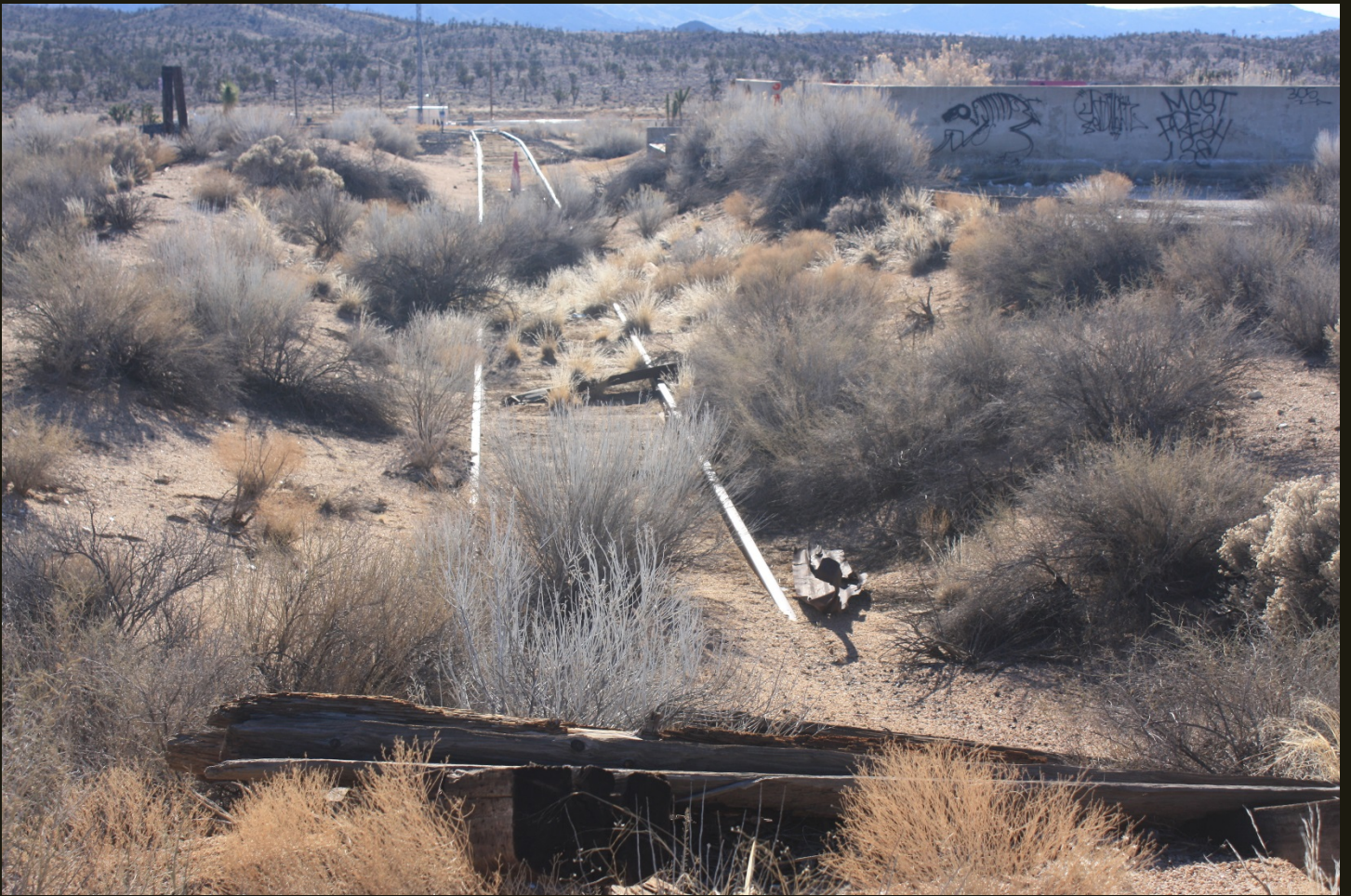
Southeastward view of the end of the Cima wye; the same concrete foundation as before is on the right.
