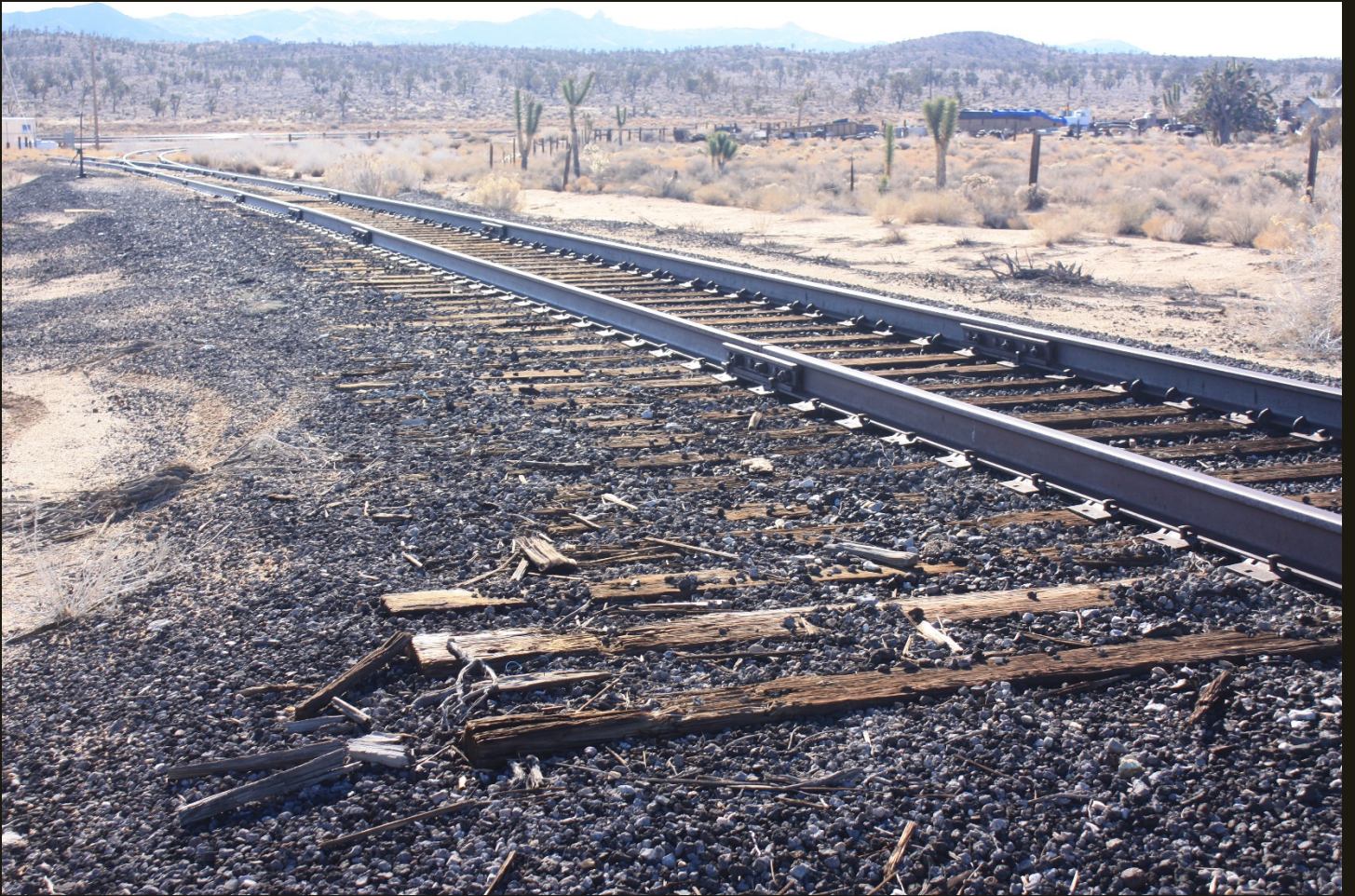
Southward view of the progressively longer ties for the former switch. The longest of the “shared” ties is in the foreground.
