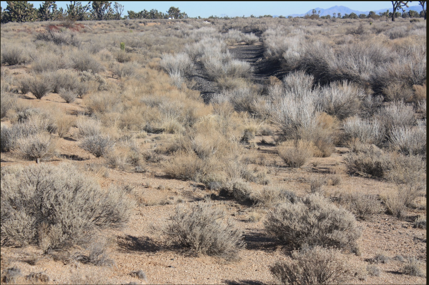
Northeastward view of the 2,000-foot abandoned spur. In this view, the curved alignment from the former switch at the wye is in the right side of the photo and we're looking directly down the 2,000-foot straight alignment. There is a linear berm to the left, with Joshua Trees on the other side; this berm could pass for a fill grade but it's more likely intended to divert surface runoff away from the track (gray gravel).
